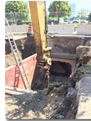
Installation of new storm pipe infrastructure
