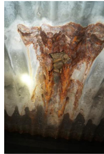
Corroded metal storm sewers require replacement
