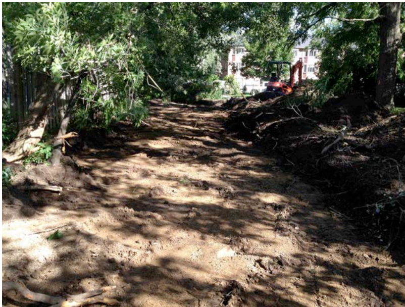
Plate 4: Stage 3 mechanical topsoil removal.
