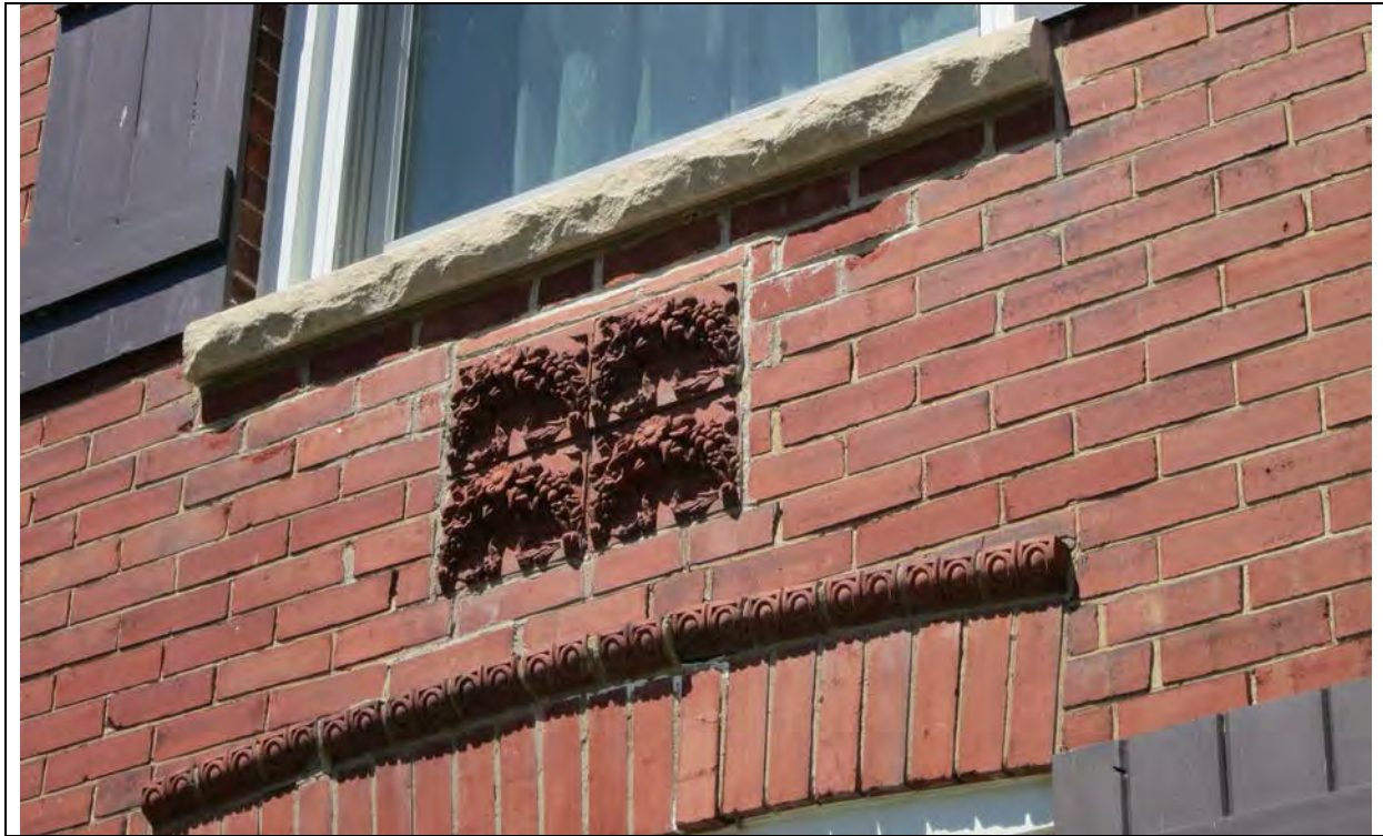
6.4 South elevation decorative terracotta brick profiles, 2017/05/08
