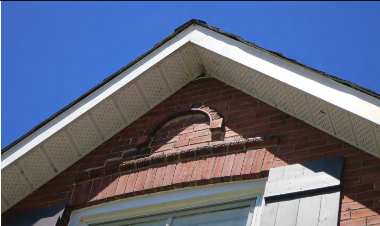
6.3 South elevation decorative terracotta brick profiles, 2017/05/08
