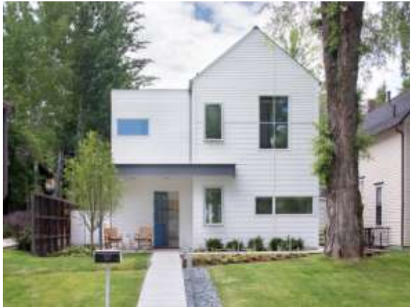
Figure 27: An example of a suitable new construction with horizontal fibre-cement siding and contextually appropriate geometries without false heritage details. The garage is separate and located in the rear. Credit: Rowland + Broughton Architects.
