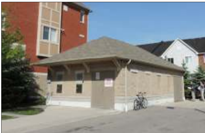
Figure 17: Waste storage room and waste collection areas should be constructed of durable materials
