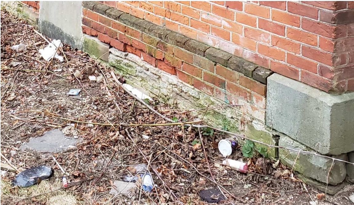
EXTERIOR – rubble stone foundation
