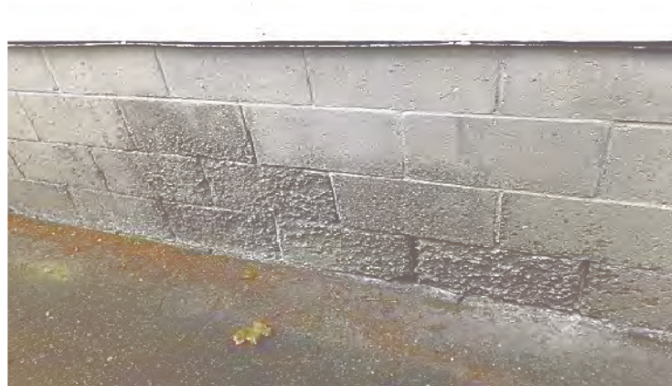
Figure 29 - Condition of cinder block foundation on southwest side
