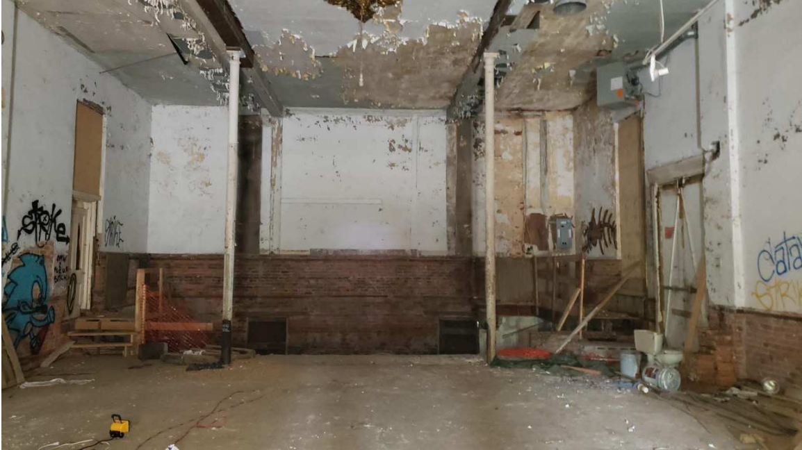
INTERIOR – 1 st FLOOR – 2 cast iron columns are original
