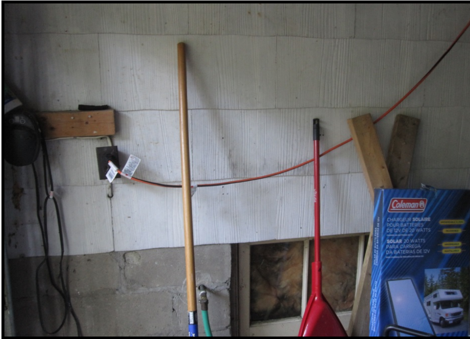
Figure 28: EXTERIOR PHOTO - View of exterior side wall of house, from inside garage, shows original asbestos siding.
