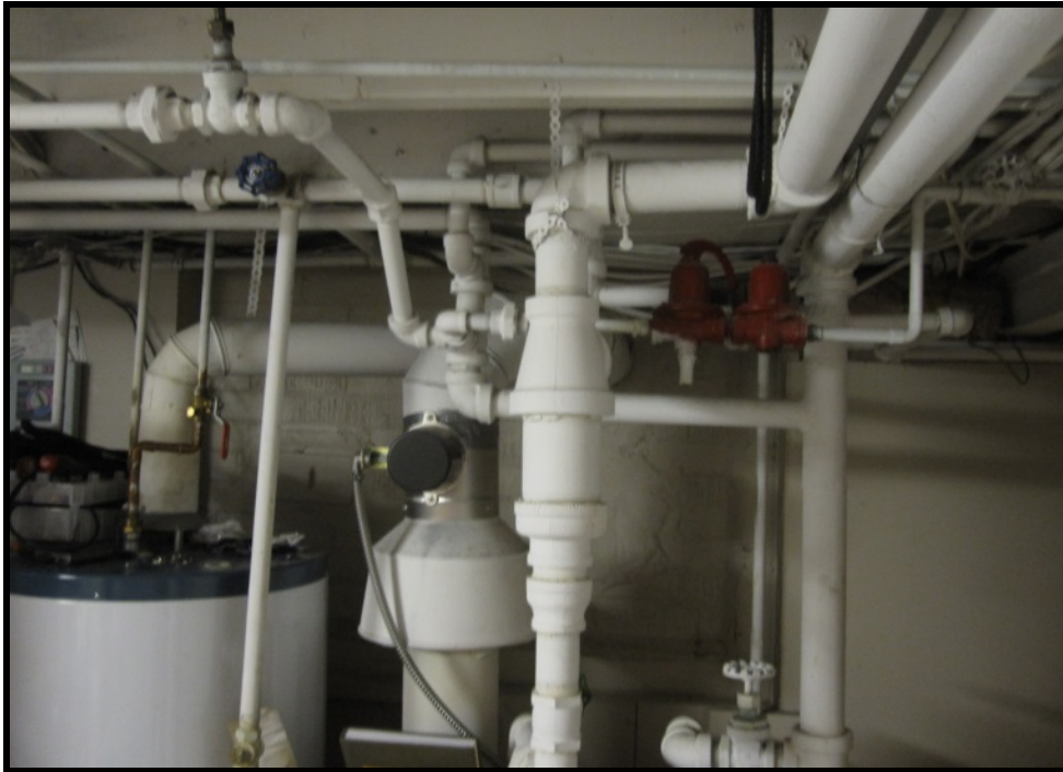
Figure 30: Basement - boiler/radiant heat plumbing.
