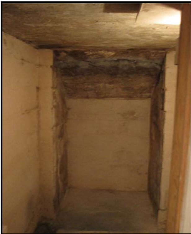
Figure 31: Basement, Cold cellar under front step, shows block foundation walls.
