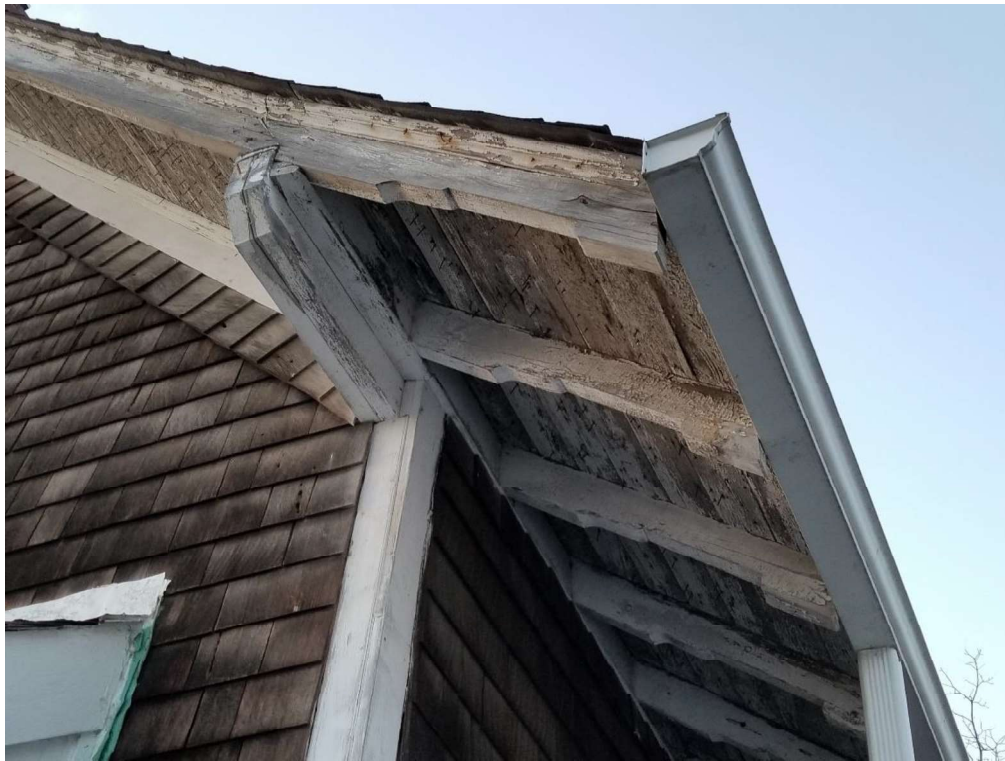
Figure 23: Projecting eaves with exposed purlins and plain fascia.
