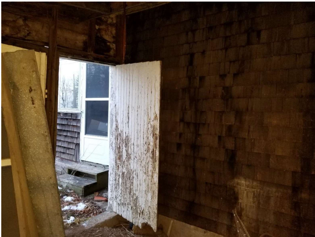
Figure 71: Wood shingles of the original structure visible from interior of the addition.
