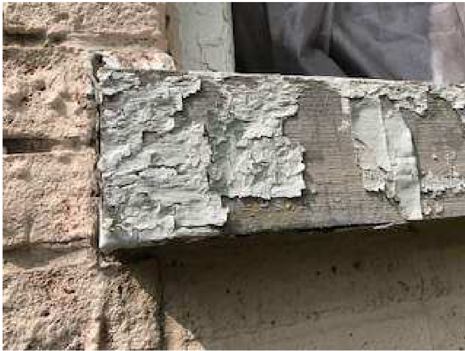
1g) Sandblasted brick, peeling paint
