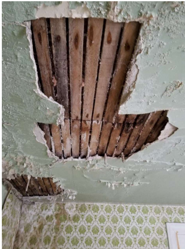
Figure 77: Exposed circular sawn lath and plaster in east living space, evidence of water damage in the left corner.
