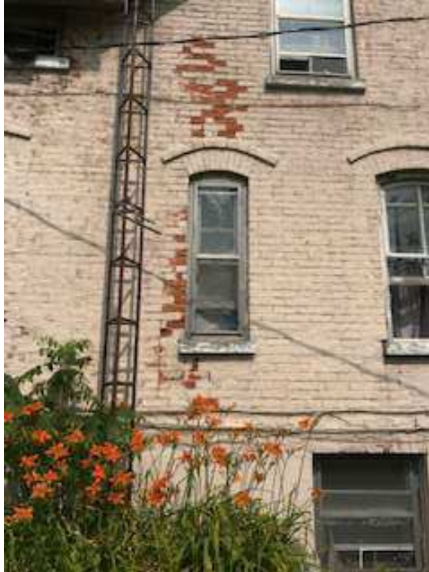
1e) Rear Façade, sandblasted brick, painted
