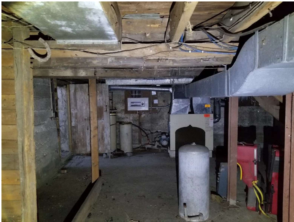
Figure 62: Machined timbers and reused beam.
