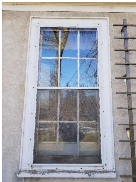
Figure 85: Typical six-over-six double hung window with storm sashes.
