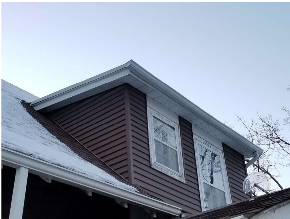
Figure 24: Shed dormer on the east façade.
