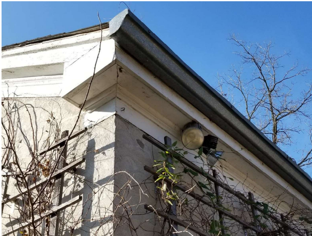
Figure 84: Boxed gable eaves and plain frieze, moulded soffit, and plain fascia of the projecting eaves and verges.
