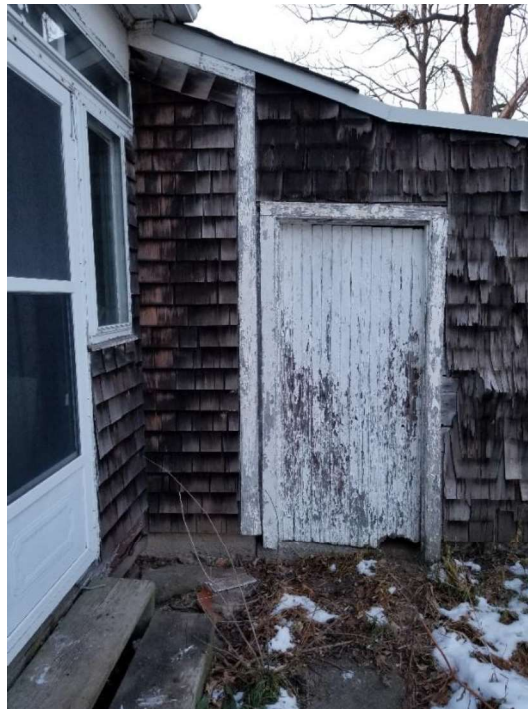
Figure 69: Vertical strip door on the addition.
