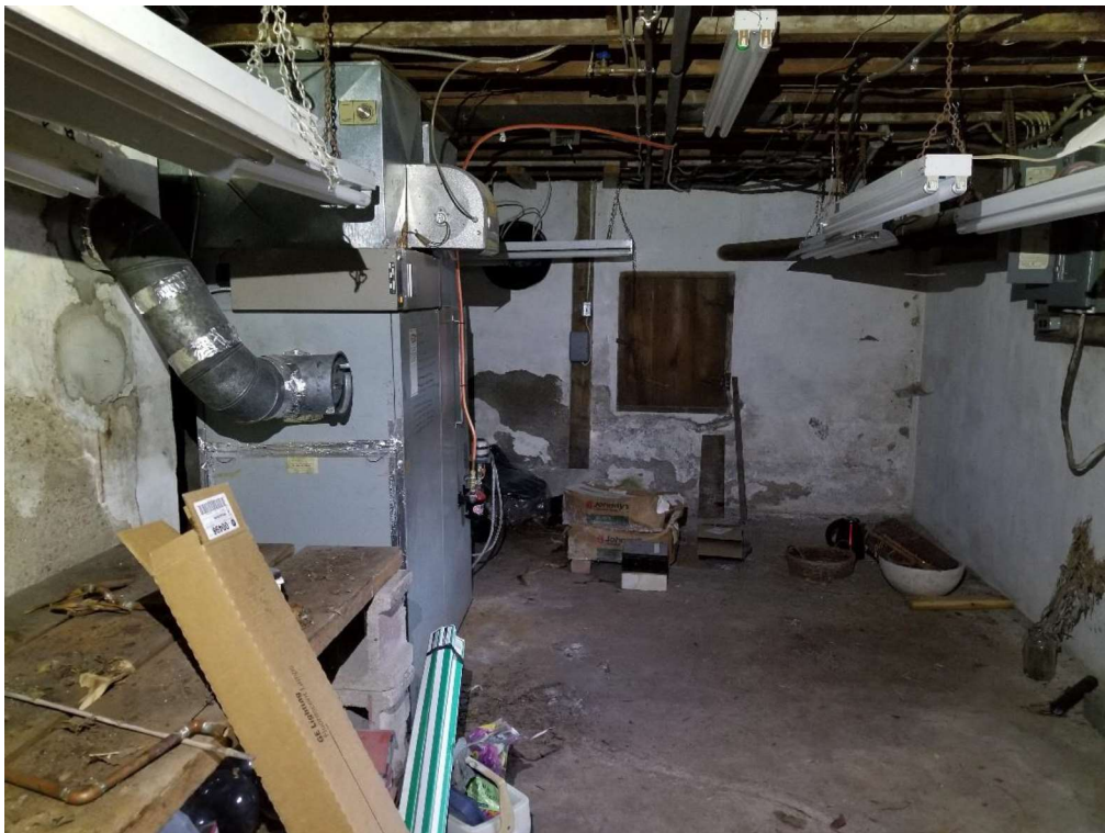
Figure 115: Original fireplace (left) now used for the furnace.
