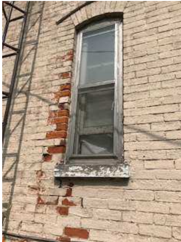
1f) Sandblasted brick, peeling paint
