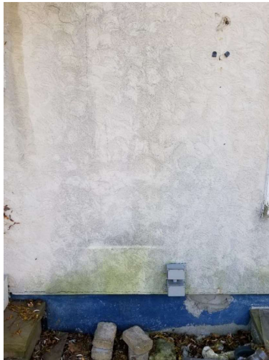
Figure 83: Concrete foundation and stucco-clad walling.
