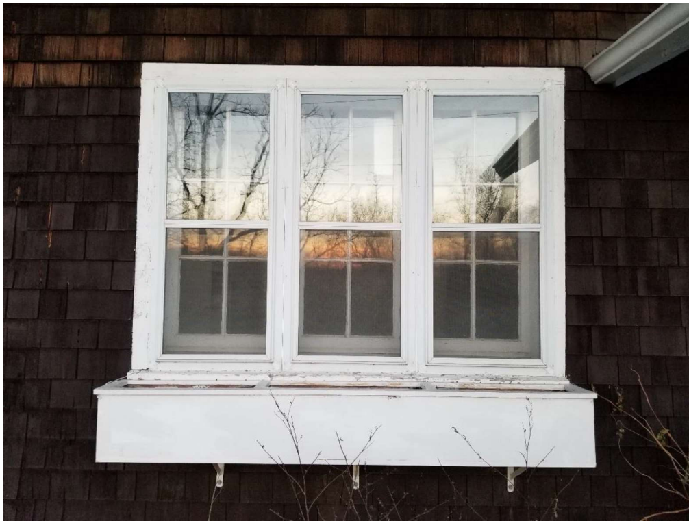
Figure 25: Adjoining casement windows with 2-over-4 fixed sashes on the west façade.
