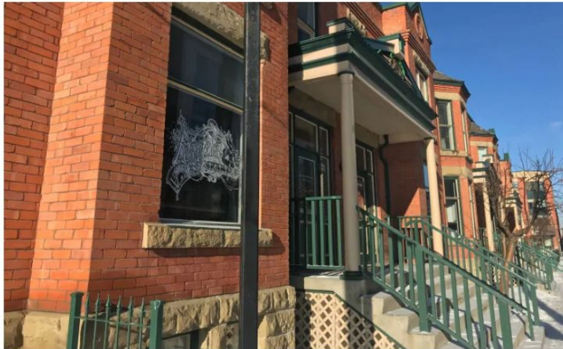
Note the sandstone foundation and trims, corbelled brick work and two-storey bay windows that make the building unique. (David Bell/CBC)
