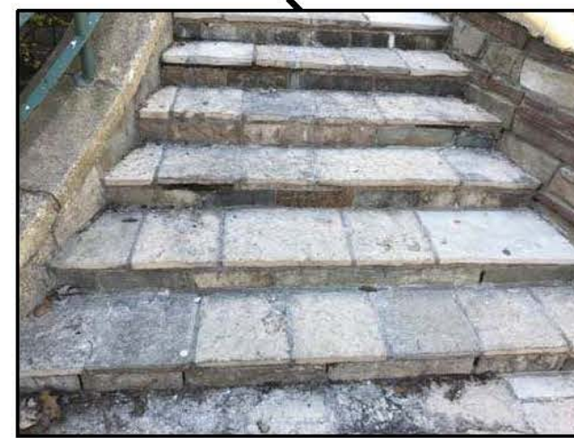
Replace South East stair to match existing Including new footing, foundation and poured concrete structure. Reuse existing flagstone if possible
