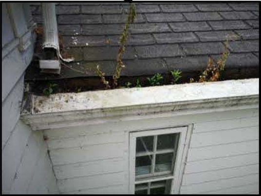
Replace gutters and downspouts to promote positive drainage and water shedding off the roof.
