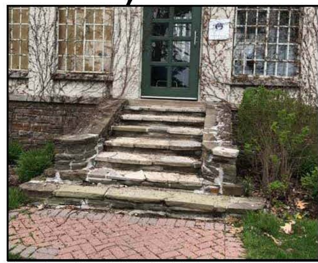
Replace South West stair to match existing Including new footing, foundation and poured concrete structure. Reuse existing flagstone if possible
