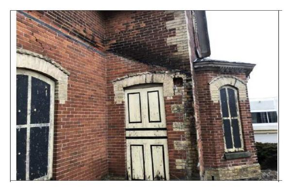
Fig # 6 – Replace all missing bricks
