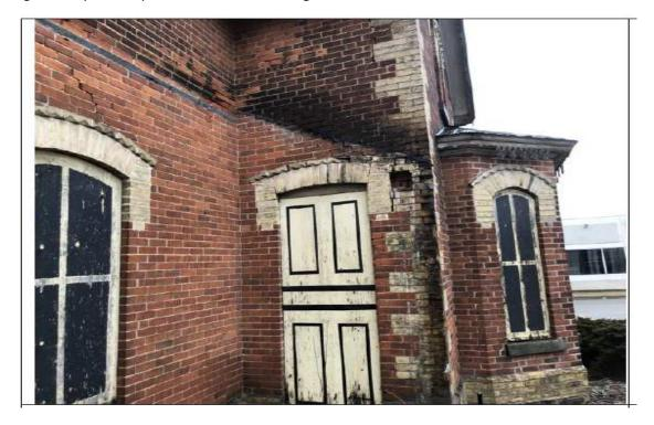
Fig # 5 Repair all diagonal cracks over windows & Doors
