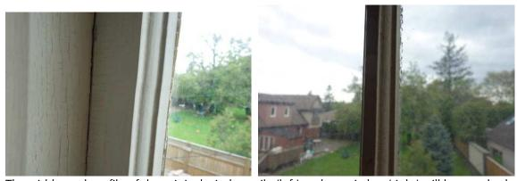
The widths and profile of the original window stile (left) and muntin bar (right) will be matched.
