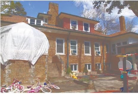
Partial south elevation (2018). The conservatory volume, on the left has wood-framed windows and an iron-framed glass dome. The base consists of bricks with stone quoins. All windows on the south elevation are modern replacements (compare with 1992 photograph on the left). Note the many dormers on the roof. The smaller ones appear as possibly be later additions. Note the water pool has been removed and the majority of the south elevation area is used as a playground.
