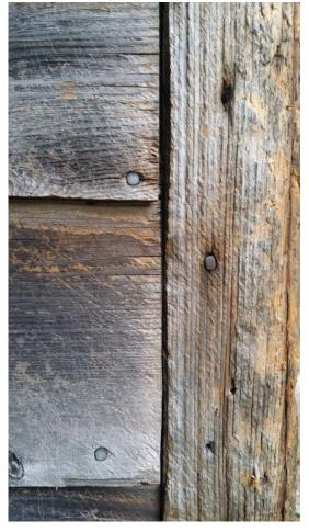
Existing siding detail showing differential nailing pattern. Horizontal siding at left fastened with newer, round galvanized nails. Vertical siding at right fastened by older, non-coated square head nail
