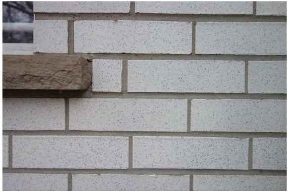
Figure 5: MATERIALS – GLAZED WHITE BRICK & CUT STONE SILLS
