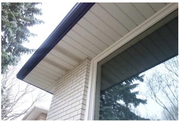
Figure 6: FEATURE - ROOF OVERHANG / MATERIALS - VINYL SOFFIT & VINYL WINDOWS
