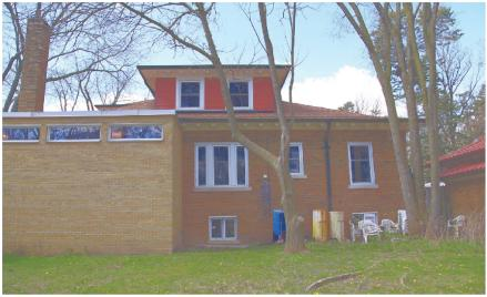
East elevation view. The 1956 addition, with buff brick, is visible on the left. Windows on the east elevation of the 1922 building appear to be modern replacements.
