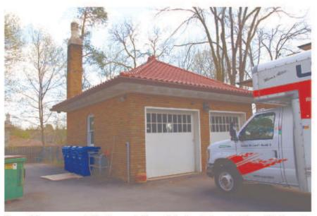
View of the garage, which shares similar architectural characteristics with the main 1922 building. The hipped roof is covered in clay tiles. The garage doors are of wood and appear to be original.
