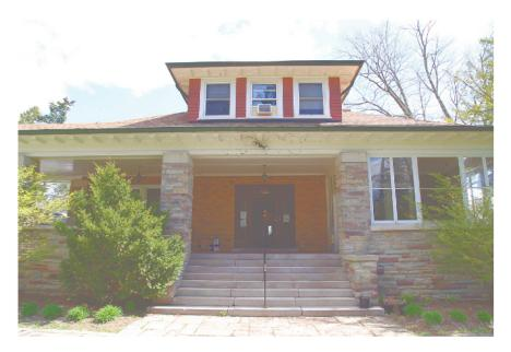
Close-up view of the west elevation and the main entrance. Note the credit valley stone cladding on the pilasters. The staircase is of concrete and is in good to fair condition, with some cracking at the joints (visible on the second step). The roof overhang is generous and features a wood soffit that is ornamented. That ornamentation is also replicated on the roof dormer. The windows to the right of the image lead to a sunroom and appear to be original.
