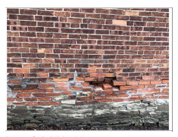
Fig # 4 – repair & replace brick where missing
