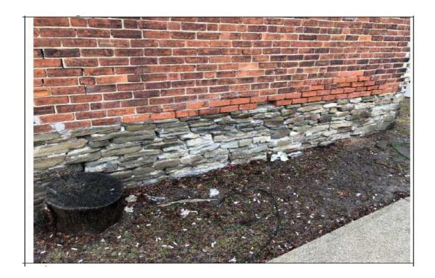
Fig #8 – re grout all brick external surfaces
