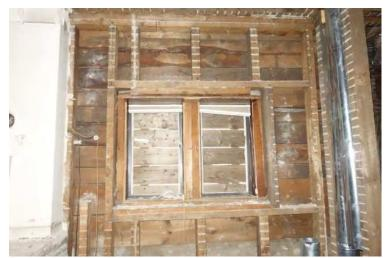
Typical condition of the original windows – missing storm window, missing lower sash, missing trim, broken sill, water damaged frame
