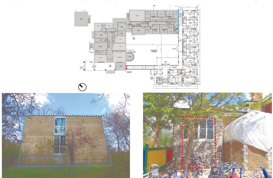
South elevation of the 1956 addition. The existing windows will be removed and the openings will be used as the passageways to the new addition.
