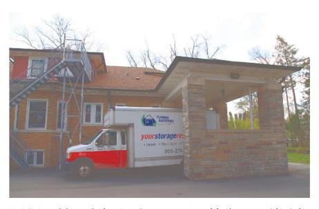
Partial view of the north elevation, showing a portion of the front verandah, clad in credit valley stone. Note the metal staircase which was added to provide a fire escape at the dormer, which has resulted in the alteration from a window to a door.
