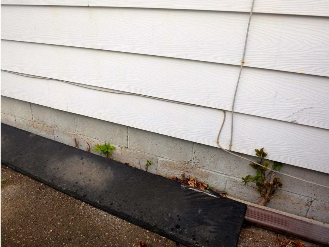
Figure 5: Concrete block foundation – no basement level
