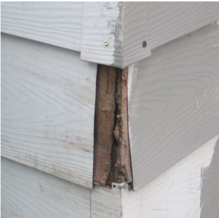
Figure 6: Corner detail – vinyl siding on top of original wood cladding
