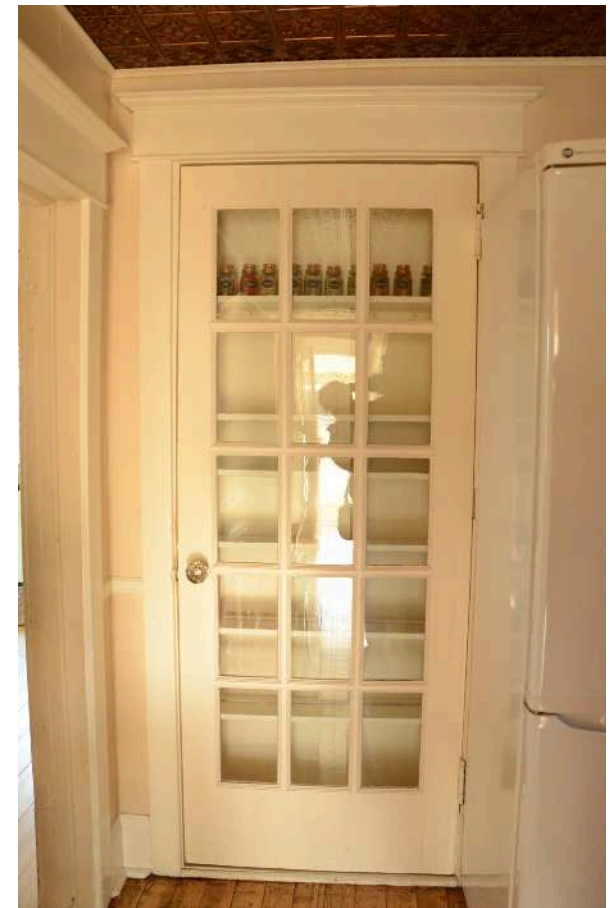
Shallow pantry/cupboard, constructed from a former doorway to the rear of the house.
