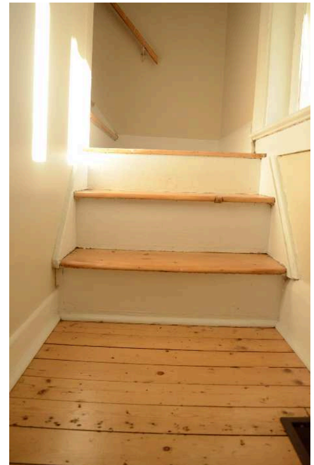
Staircase off of the entry way leading to the second floor. (Not OBC compliant - steep and narrow)
