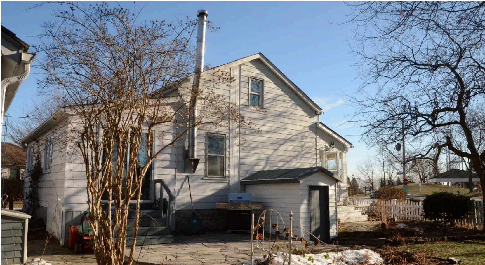
View of the house from the yard on the west: The front of the house is a 1 1/2 storey section with a smaller one storey addition at the rear (north side). A strip of vertically oriented siding indicates where the original brick chimney was located.
