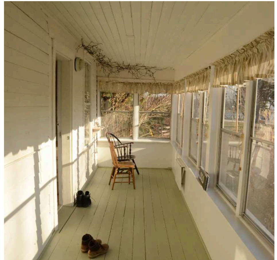
Photo taken in the enclosed porch on the south side of the house. Photo is looking east, windows are aluminum frames set between the wood columns.
