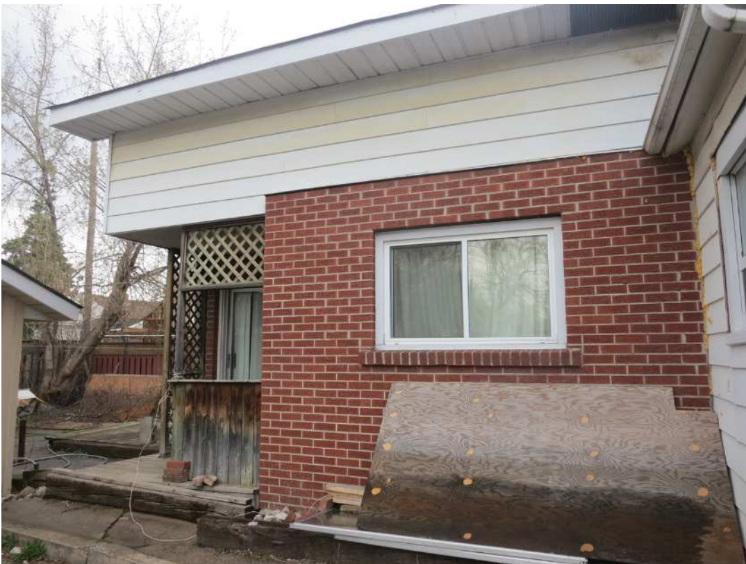
Figure 8: Rear addition – modern addition with brick and vinyl cladding
