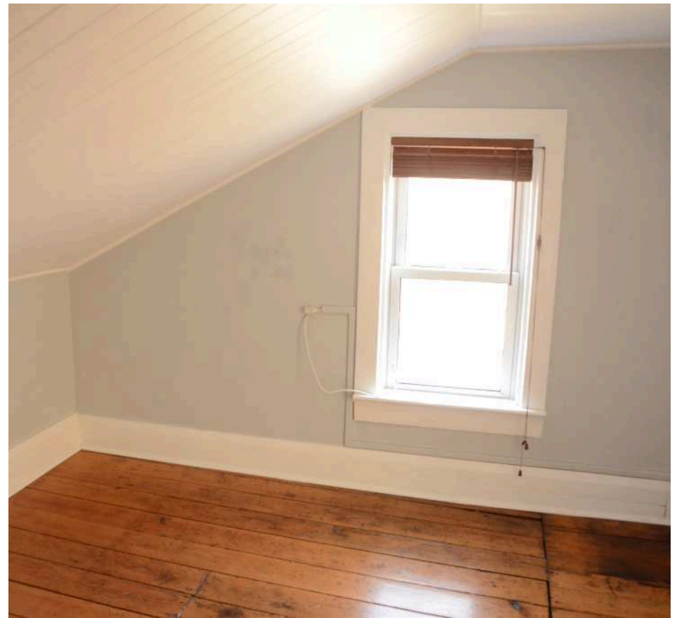
Ceiling is clad in a wainscoting pattern, above is a lath and plaster ceiling. The sloped sections are clad in wood. The flat portion is lath and plaster.
