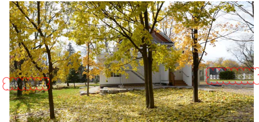
2018 PHOTOGRAPH SHOWING AS-BUILT CONDITION – PERIMETER FENCING
