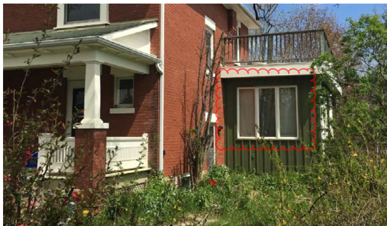
2016 PHOTOGRAPH SHOWING ORIGINAL CONDITION
