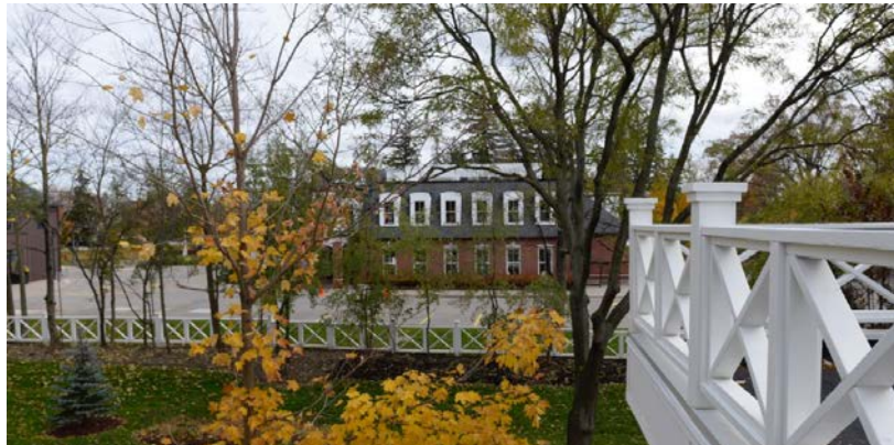
2018 PHOTOGRAPH SHOWING DETAIL OF FLAT ROOF GUARD AND RELATIONSHIP TO PERIMETER FENCING
