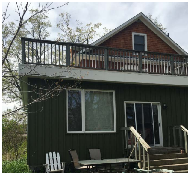
2016 PHOTOGRAPH SHOWING ORIGINAL CONDITION
