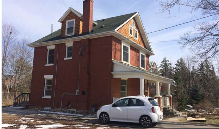
2016 PHOTOGRAPH SHOWING ORIGINAL CONDITION – NO PERIMETER FENCING
