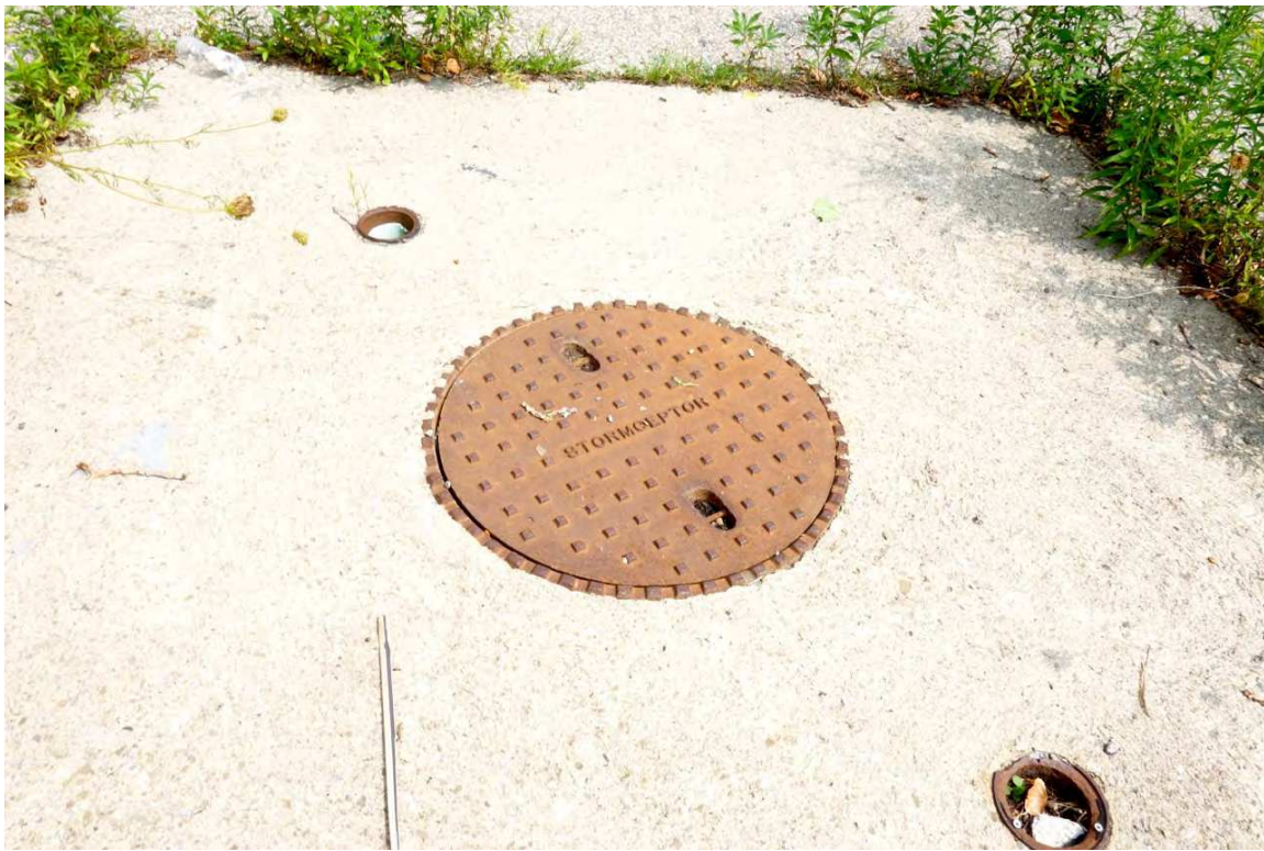
Access to storm drain located on the property
