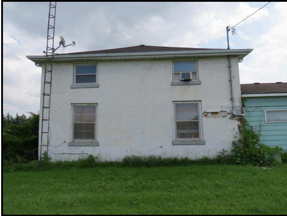
Image 27: North Elevation (Photo taken on June 13, 2018; Facing South)
