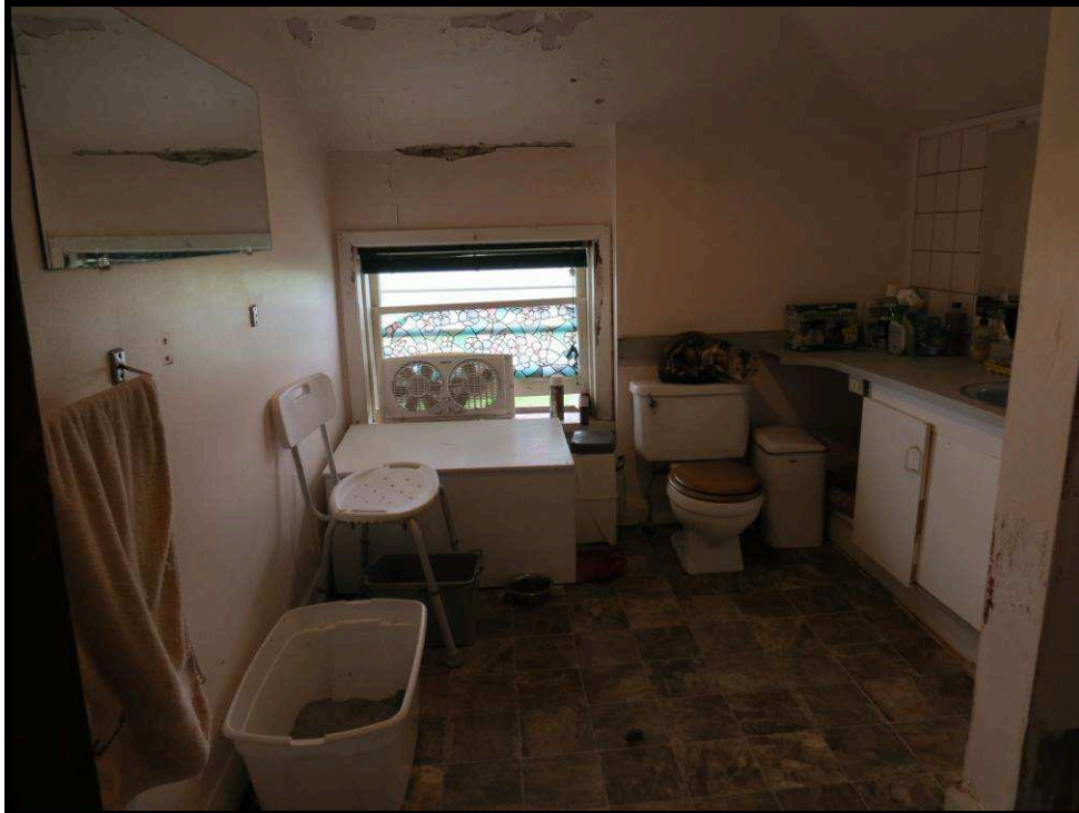
Image 48: Bathroom (Photo taken on June 13, 2018; Facing South)
