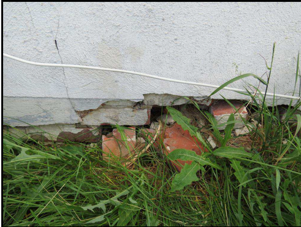
Image 30: Detail of foundation (Photo taken on June 13, 2018; Facing South)
