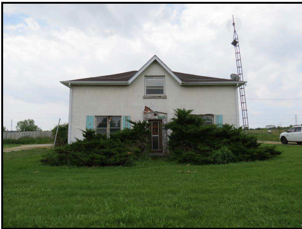
Image 8: Façade of 6432 Ninth Line (Photo taken on June 13, 2018; Facing West)
