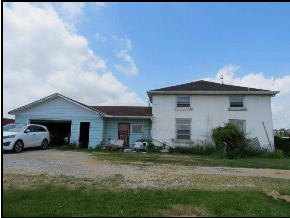
Image 19: South Elevation (Photo taken on June 13, 2018; Facing North)
