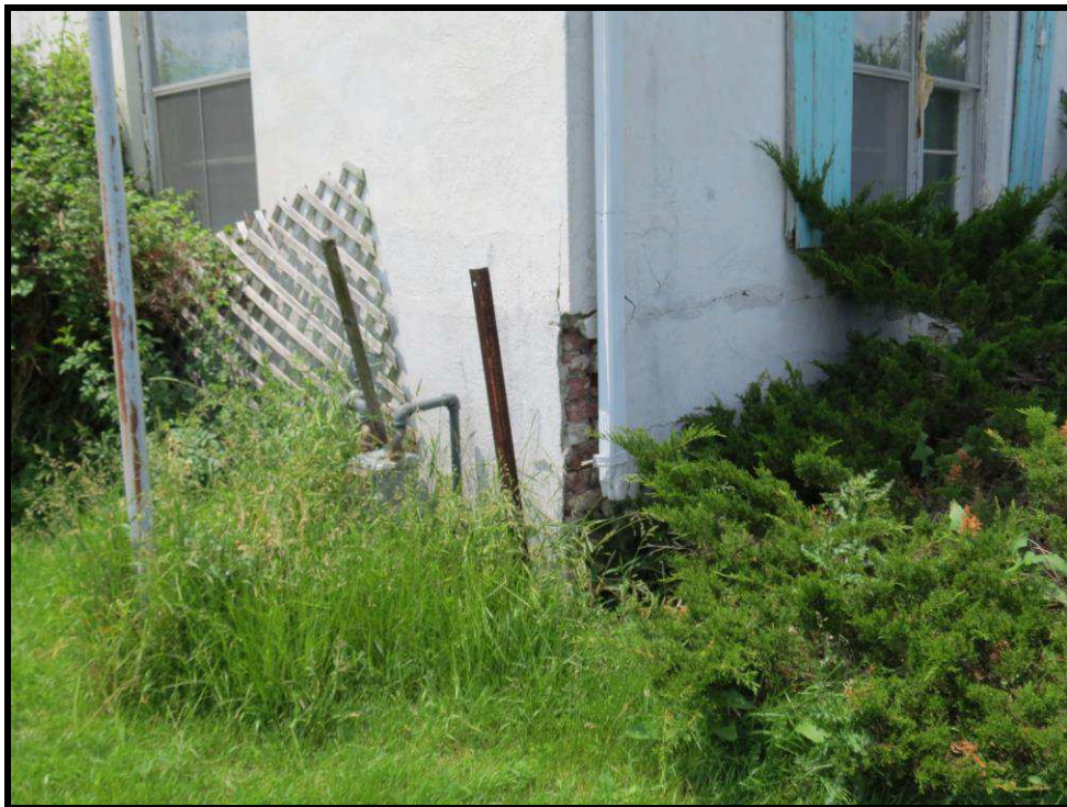
Image 18: Detail of southeast corner (Photo taken on June 13, 2018; Facing Northwest)
