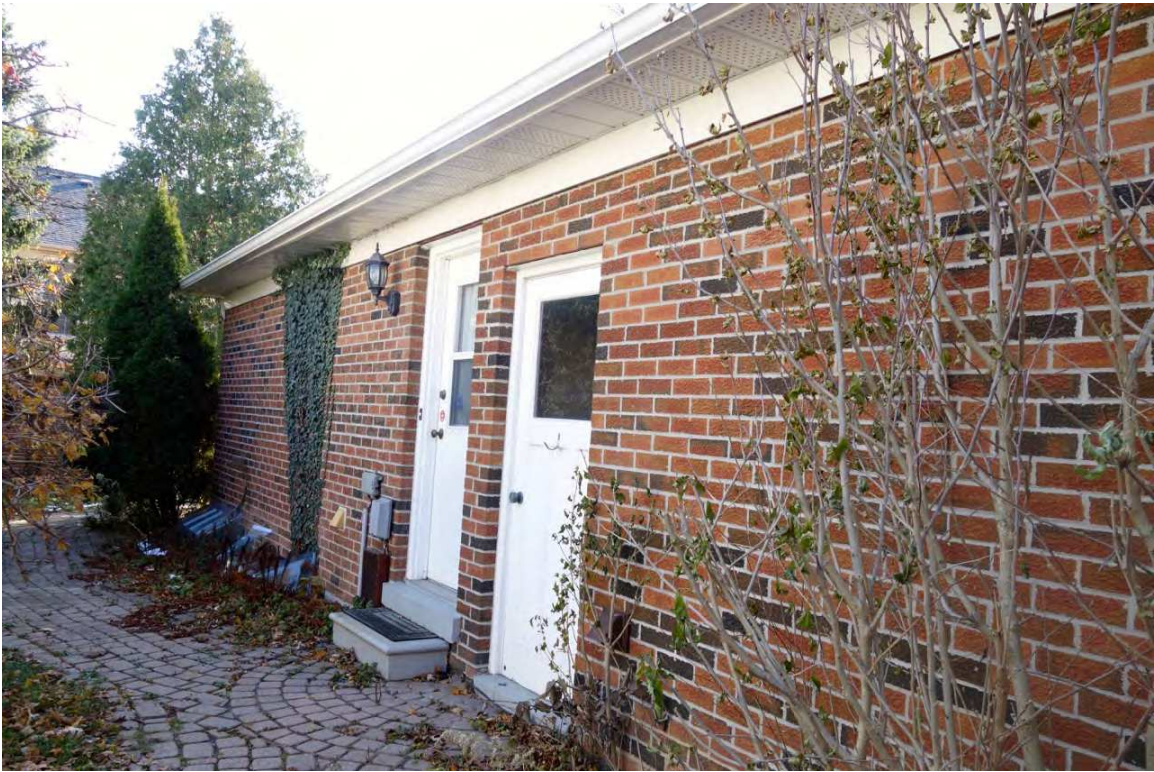
2104 Mississauga Road – SIDE ELEVATION
