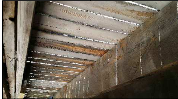
UNDERSIDE OF PORCH SHOWING OLDER JOISTS, DECK BOARDS, NOT SOME DECK BOARDS FINISHED ON UNDERSIDE, OTHERS NOT
