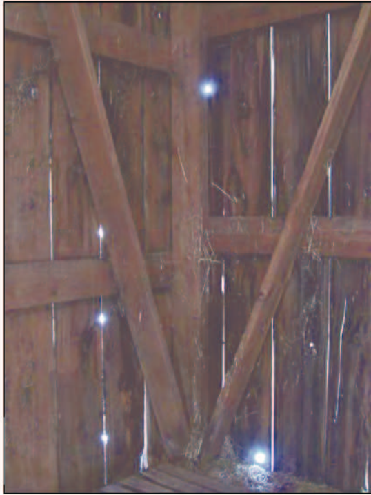
35. The corner posts contain 2 2-in. (51 mm) by 8-in. (203 mm) boards bolted directly together.
