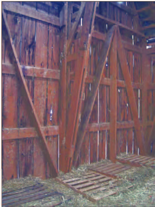
36. The truss posts are 2 2-in. (51 mm) by 8-in. (203mm) boards separated by 2-in. (51 mm) braces and bolted together.
