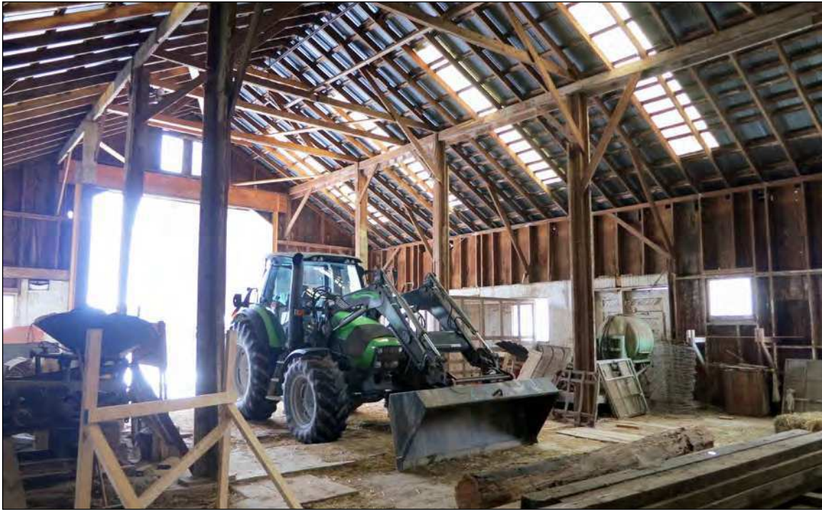
39. Atypically, the light frame construction of the upper level of the small barn has interior posts that interrupt the flow of the space.
