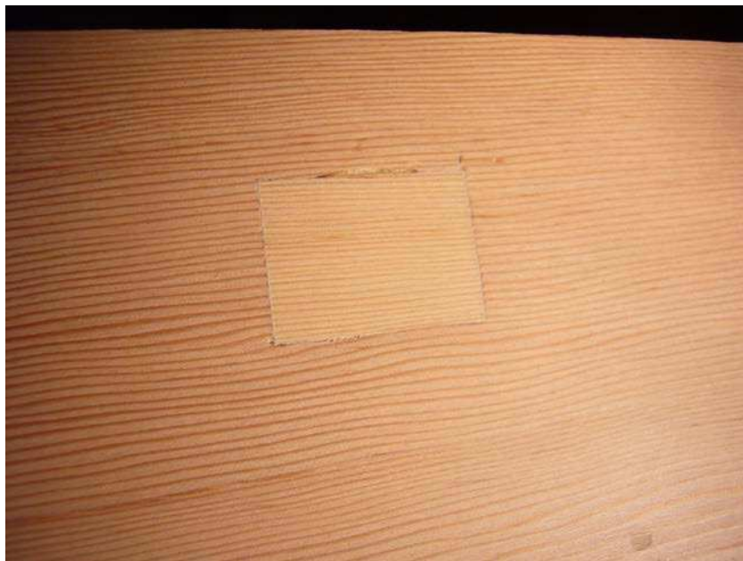
Typical "Dutchman" repair in finish grade wood – term refers to the cutting out and replacement of damaged or rotted wood elements and replacement with new wood cut to fit and glued in place
