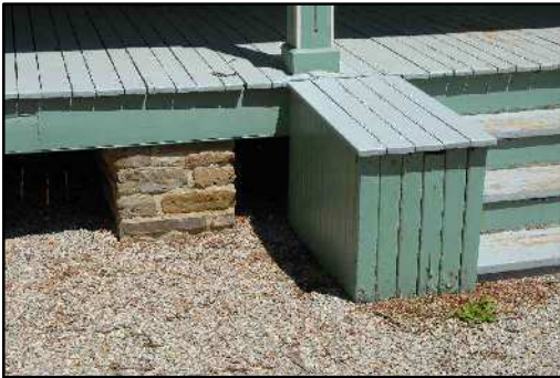
PORCH BASE SHOWING STONE FOUNDATION
