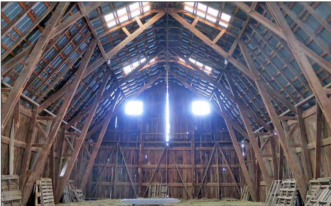
32. A large opening fitted with double-leaf hinged doors is located in the north gambrel end wall.
