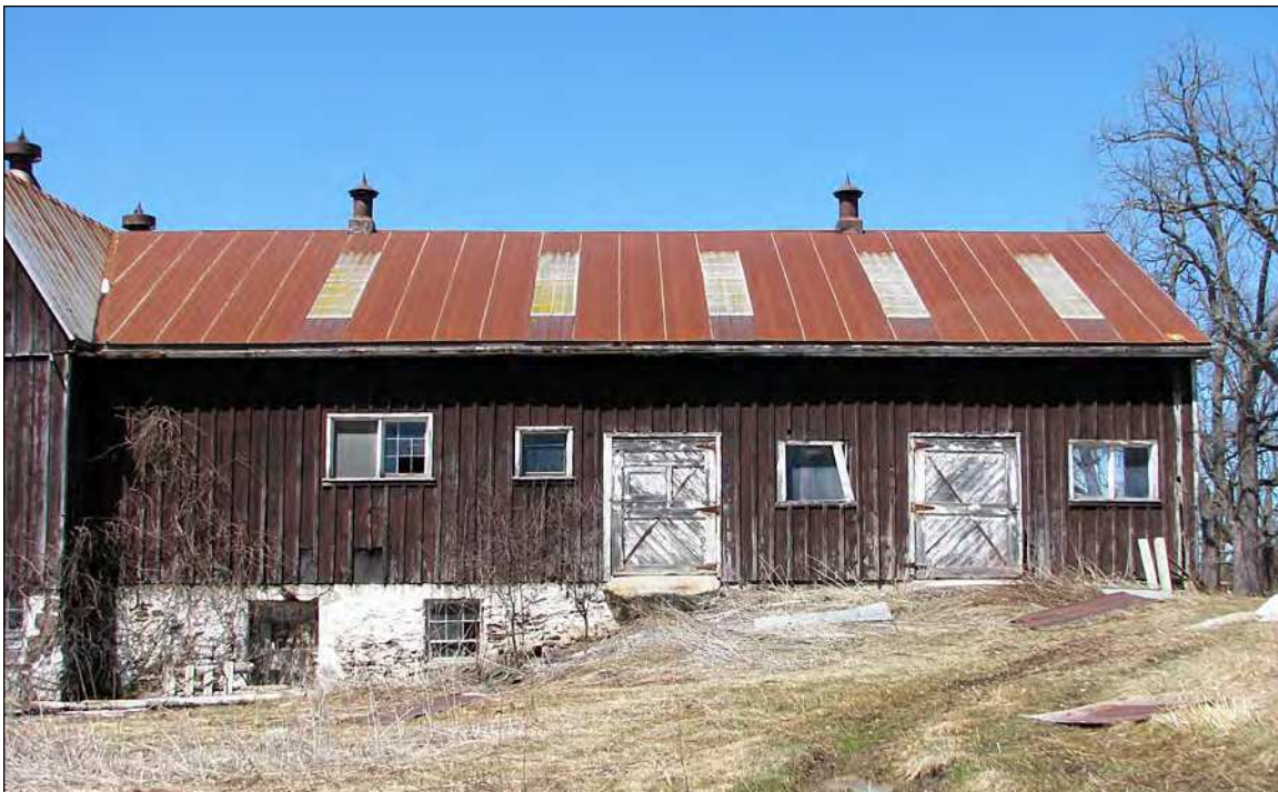
24. The exposed south foundation wall of the small barn is rubblestone. The doors on the upper level may relate the horse stable use of the building.
