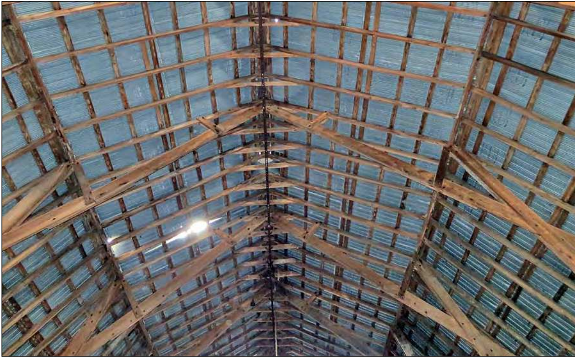
13. At the peak the roof framing comprises ridge supports, collar ties and rafters. The purlin plate and purlin supports are visible at the change in slope of the gambrel roof.
