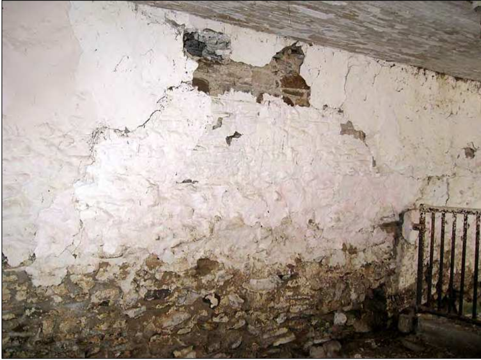
37. The interior wall between the north and south rooms on the lower level of the small barn is rubblestone.
