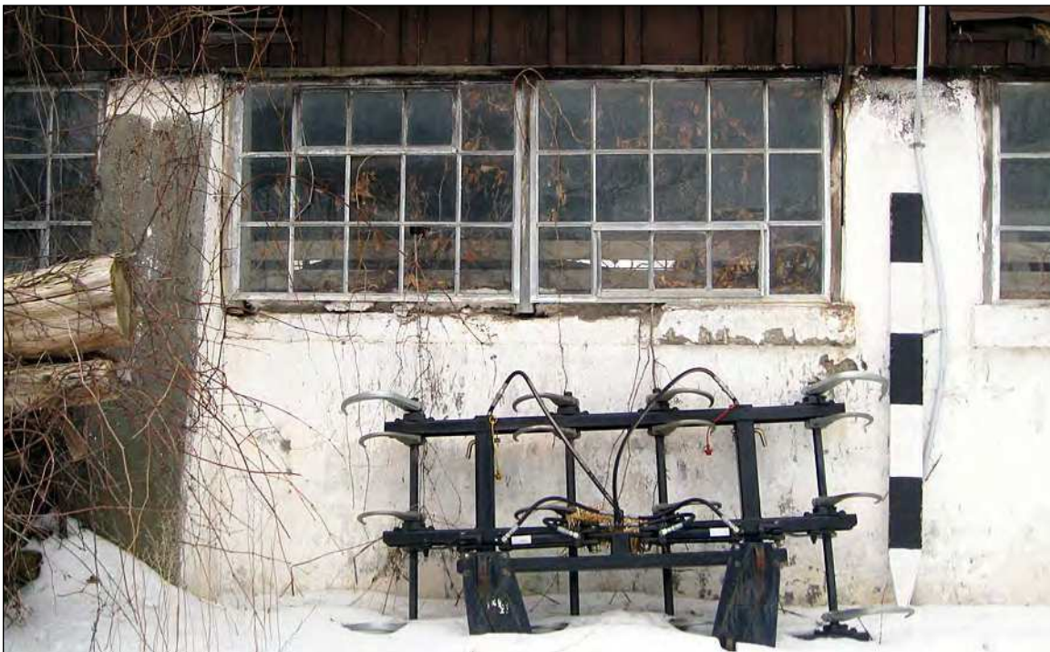
6. Pairs of window openings fitted with multi-paned metal sash are located in the upper part of the foundation wall. A portion of the sash is operable for ventilation purposes.
