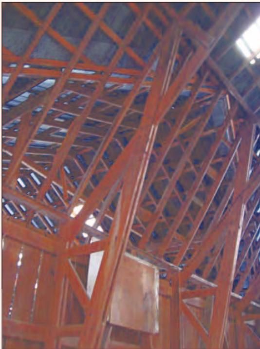
33. The roof framing contains ridge supports, collar ties and rafters with the purlin plate and purlin supports located at the change in slope of the gambrel roof.
