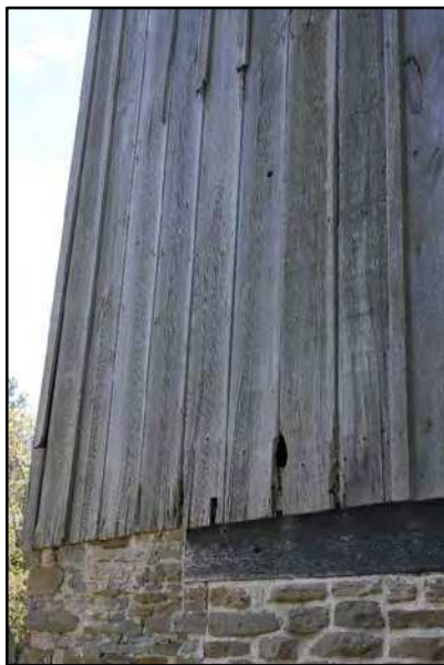
NOTE DETERIORATED BOARDS, MISSING BATTENS, TYP ALL ELEVATIONS
