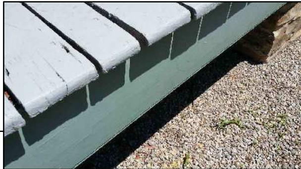
PORCH FLOOR SHOWING RANDOM WIDTH OF BOARDS
