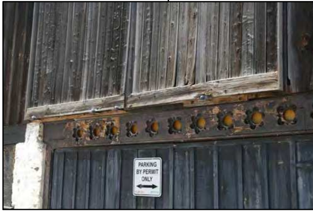
NOTE GENERAL DETERIORATION OF UPPER DOOR, FILAGREE DETAIL
