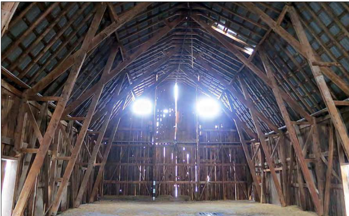
12. The plank frame was built up of sawn lumber normally 2-in. (51 mm) by 4-in. (102 mm) to 12-in. (305 mm) bolted together.
