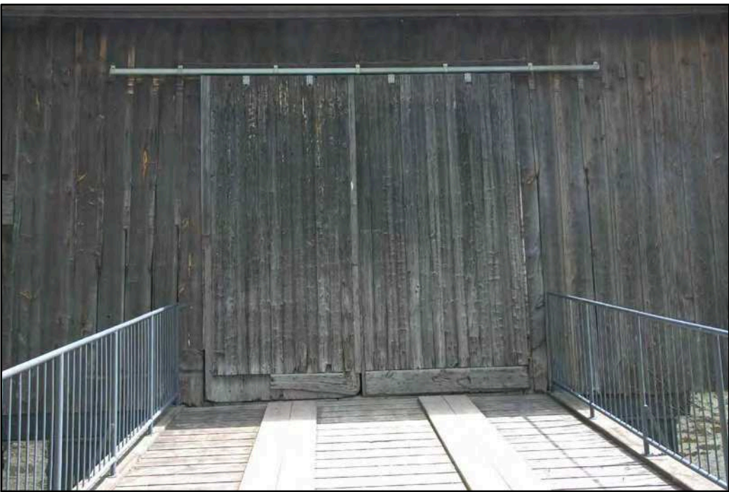
BARN DOOR ASSEMBLY - NOTE NEWER GUARDS, RAILS AND RAMP
