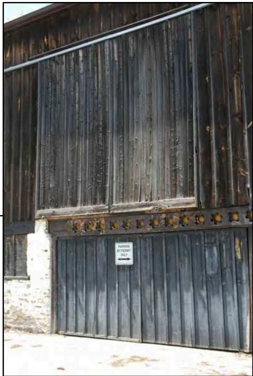
NOTE UPPER AND LOWER DOORS. UPPER DOOR IS FIXED IN POSITION. LOWER DOOR IS NEWER AND OPERATES
