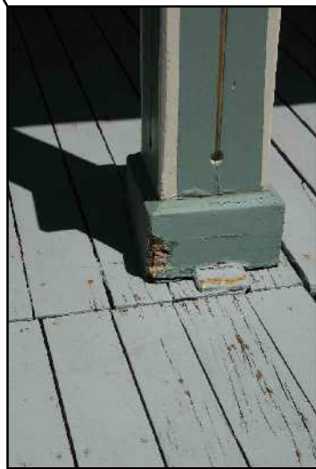
COLUMN BASE SHOWING MECHANICAL DAMAGE, DETERIORATION
