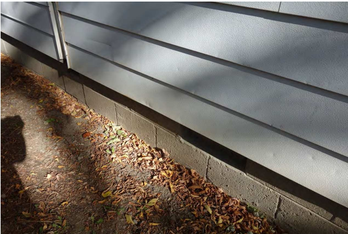
Figure 10: Raised concrete block foundation, vinyl siding.
