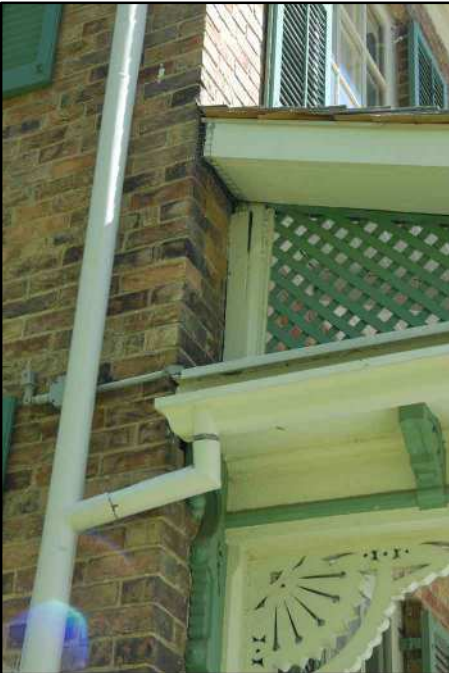
SOFFIT SHOWING ANIMAL INTRUSION, TRIM SHOWING DETERIORATION
