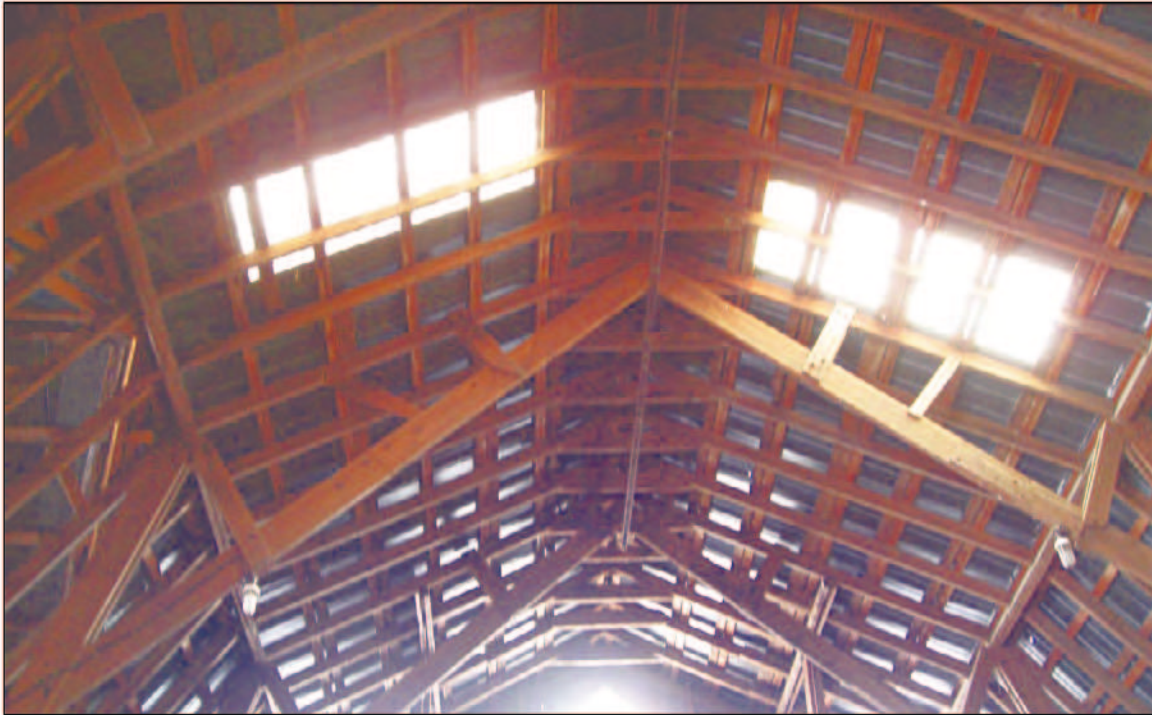
33. The roof framing contains ridge supports, collar ties and rafters with the purlin plate and purlin supports located at the change in slope of the gambrel roof.
