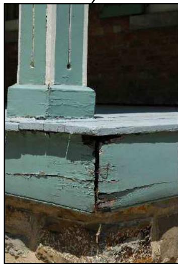
SKIRTING BOARD SHOWING DETERIORATION
