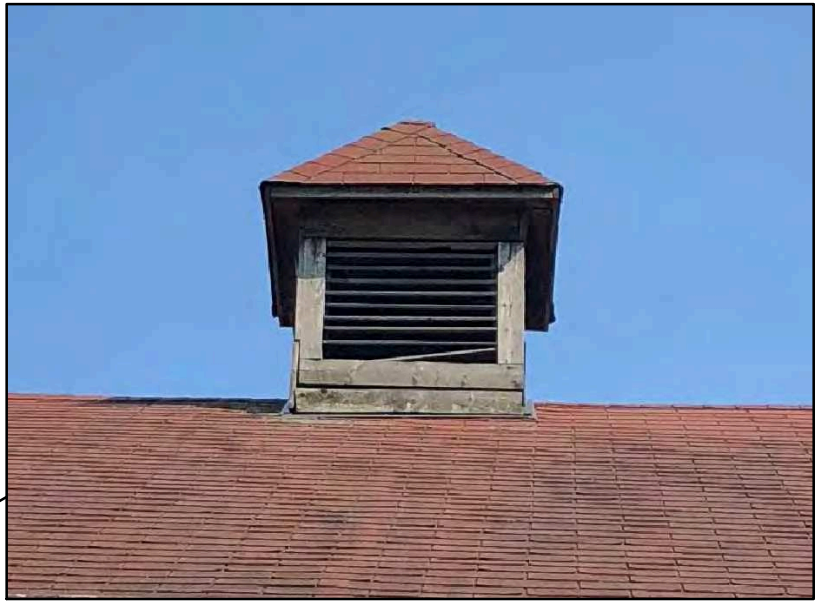
CUPOLA SHOWING GENERAL DETERIORATION, MISSING/BROKEN PIECES
