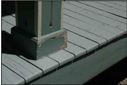
POST BASE SHOWING PAINT LOSS, DETERIORATION (TYP ALL POSTS)
