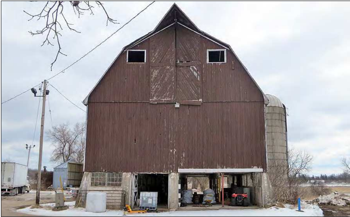
3. Large openings in the foundation wall provided access to the lower level for livestock and equipment. Note the large opening on the upper level for the movement of hay to the mow.
