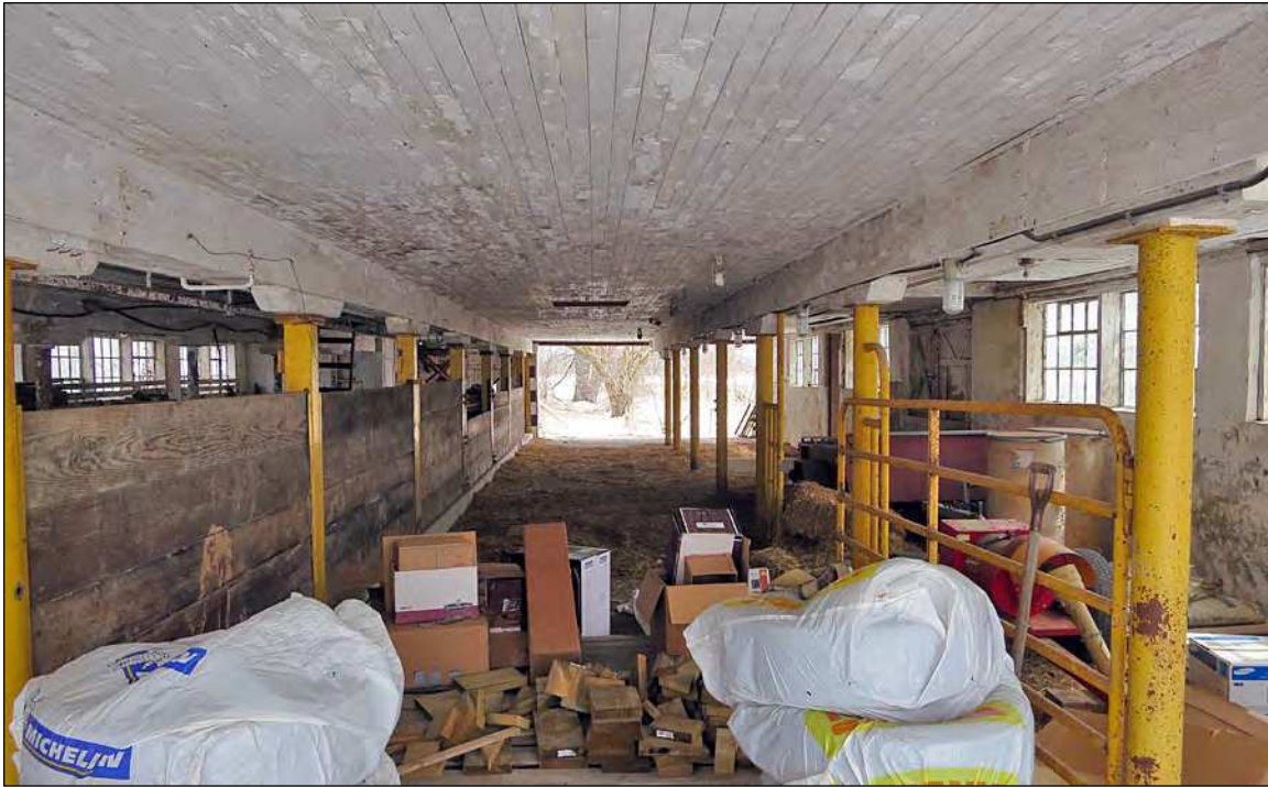
9. A view south depicts the longitudinal beams and posts, which divide the lower level into three parts. Note the tongue and groove ceiling boards. The walls and ceiling are painted white.
