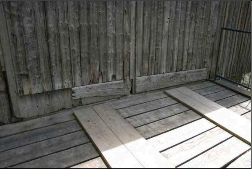
BARN DOOR MISSING/BROKEN PIECES AT BOTTOM
