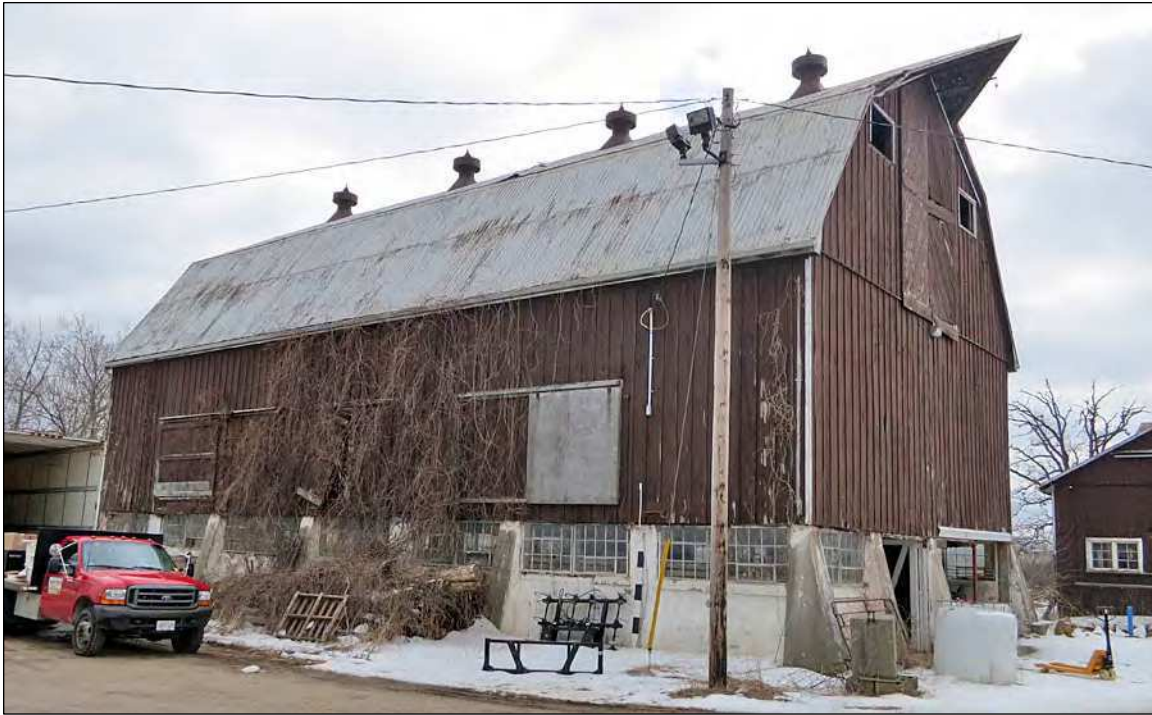
1. The two-storey Upper Barn has a cast-in-place concrete foundation, plank frame superstructure clad in board and batten siding and gambrel roof finished in corrugated sheet metal.
