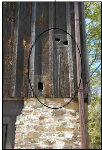
NOTE HOLES GNAWED BY ANIMALS (TYP ALL ELEVATIONS)
