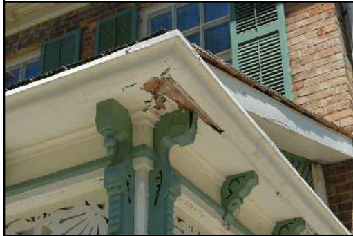
SOFFIT SHOWING WATER DAMAGE
