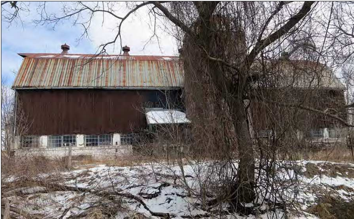
22. Characteristic elements of the Lower Barn include pairs of windows in the foundation wall, dark coloured board and batten siding and metal clad gambrel roof with ventilators.
