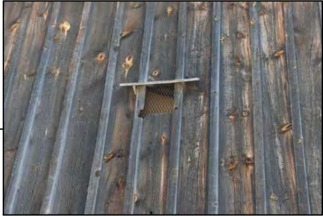
NOTE VENTILATION OPENING WITH WOODEN DRIP EDGE DETAIL
