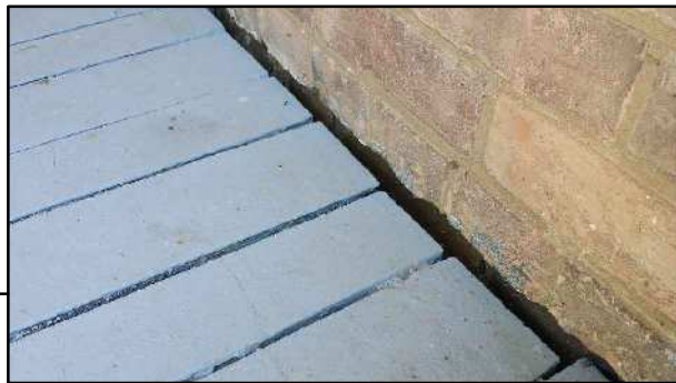
PORCH FLOOR SHOWING SEPARATION OF BOARDS FROM HOUSE WALL
