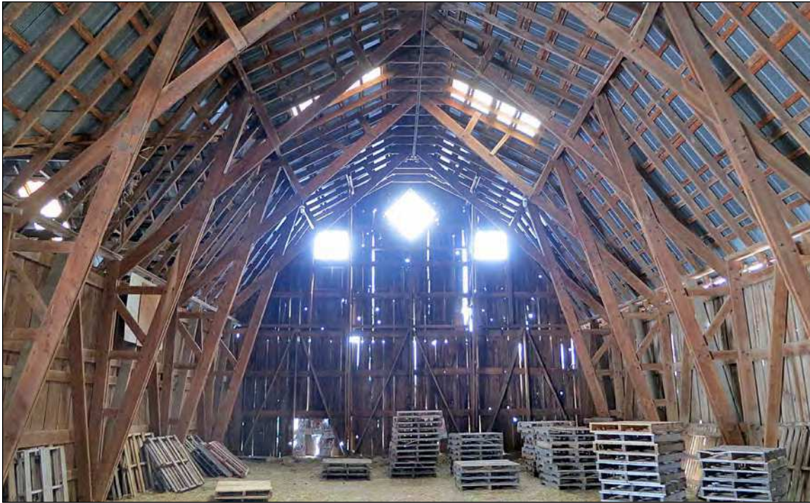
31. A view south through the upper level of the large barn shows the plank frame construction.
