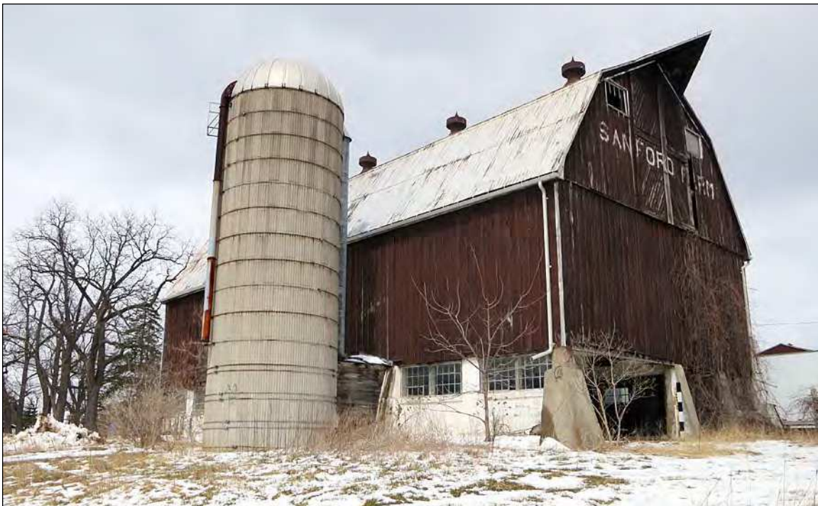
2. Concrete buttresses around the foundation wall may have been added to provide additional structural support.
