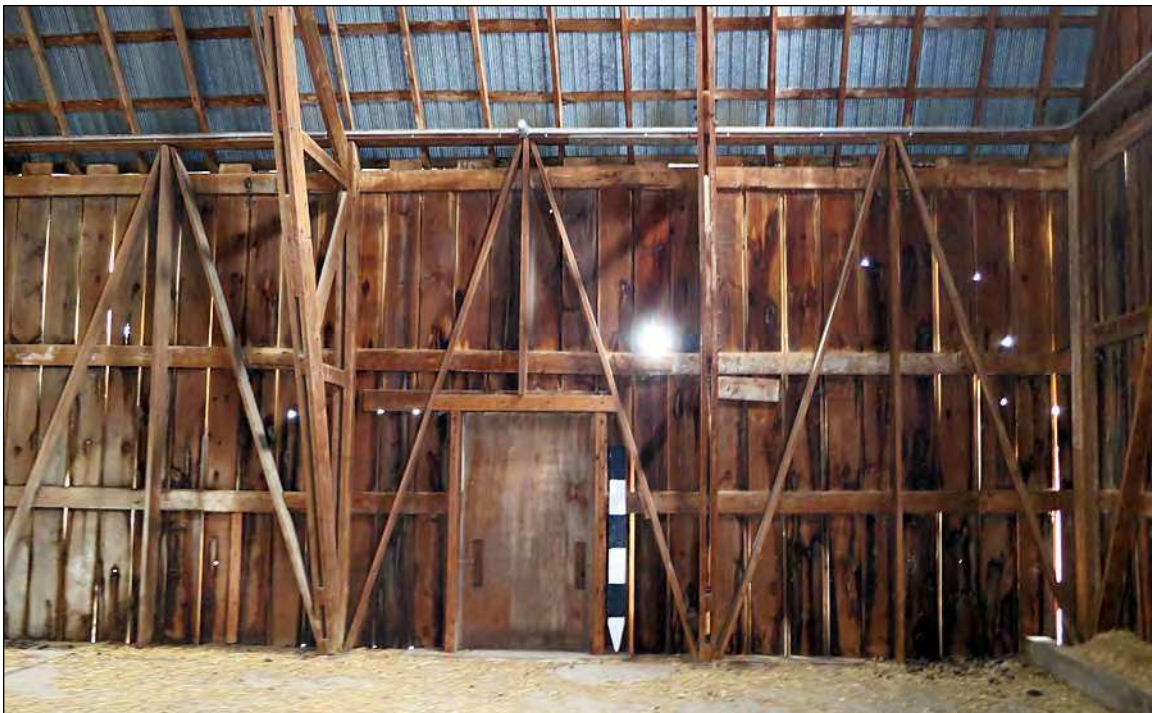
14. The wall framing contains a truss post tied into the purlin support. The bays between the truss posts feature girds, wall plate, stud and diagonal bracing.
