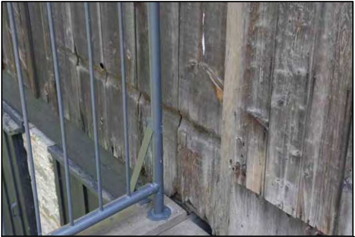
BARN DOOR MISSING BOTTOM GUIDE - NOTE GROOVE WORN IN SIDING BOARDS
