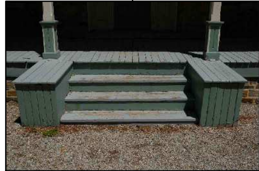
PORCH STEPS SHOWING PAINT LOSS
