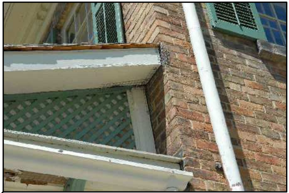
SOFFIT SHOWING WATER DAMAGE, ANIMAL INTRUSION
