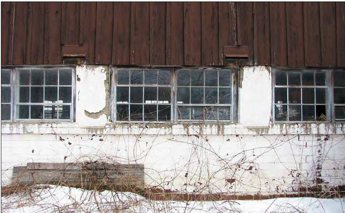
28. A detail of the foundation depicts the paired window openings set between concrete piers and with concrete sills in upper wall. The white paint obscures the hollow-clay tile of the lower wall.
