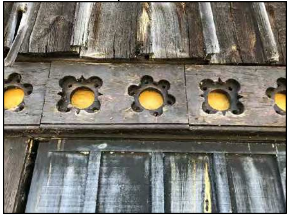
FILAGREE DETAIL AT SOUTH DOORS TO BE CONSERVED. NOTE DETERIORATION OF BOARDS & BATTENS ABOVE, NEWER PAINTED GARAGE DOOR
