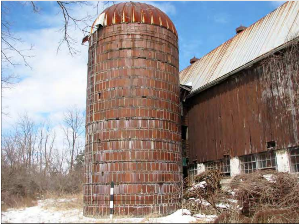
27. The use of fireproof hollow-clay tile for the silo is considered an unusual application of the material.
