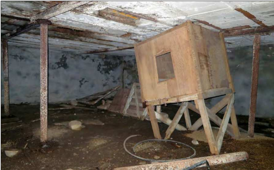
38. The north room, a former root cellar, appears to use a steel structure.
