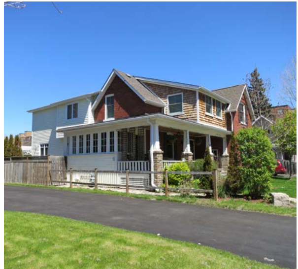
Figure 24: An example of a suitable rear 1.5 storey addition to an existing house on a contributing property with preferred materials of horizontal siding, brick, and wood shingle. The scale and landscaping are complementary to the District. Photo credit: GRA.
