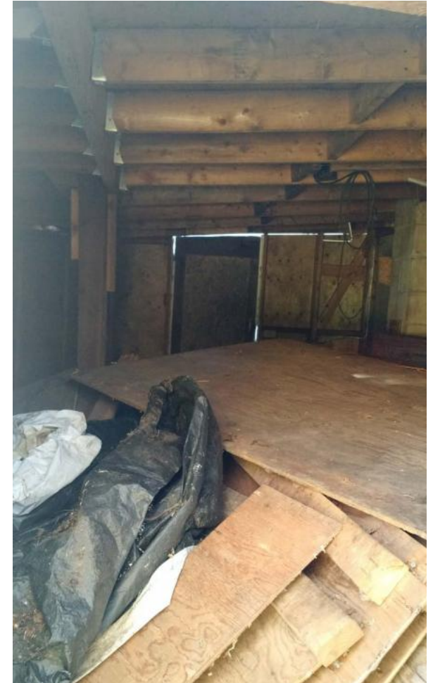
Interior of Garage Addition - currently holding wood scraps. The construction is simple and is not weatherized.
