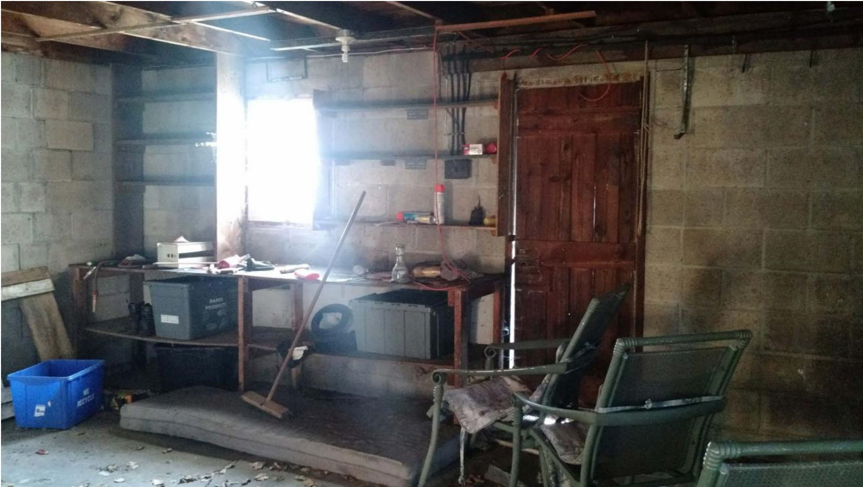
Interior View of the Garage - South East Wall - the Window and Door are not in good condition. The door lacks a solid frame, and is not weatherized.
