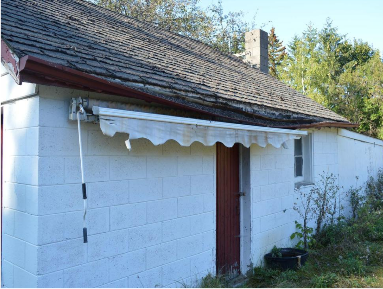
The eavestrough is in need of repair and the block walls also contain cracks.
