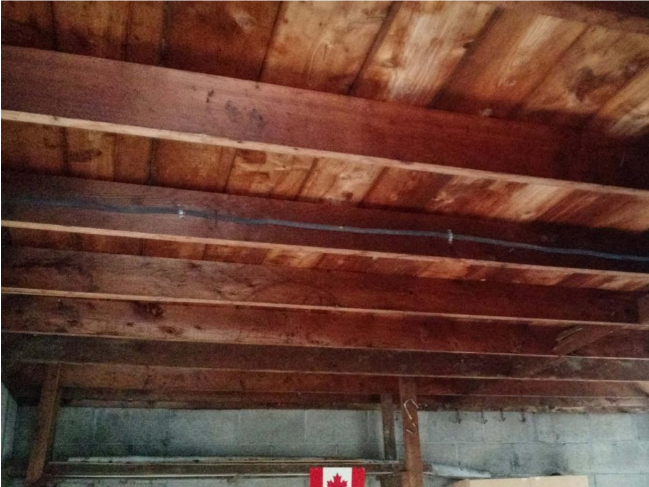
Interior view of the Garage - Ceiling - The wood joists appear to be in good condition, with a wood floor laid above them for potential storage. No access to the upper portion was visible
