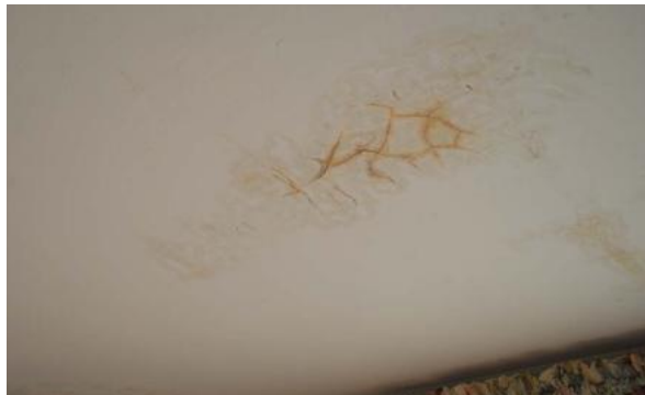
Ceilings show areas of water damage
