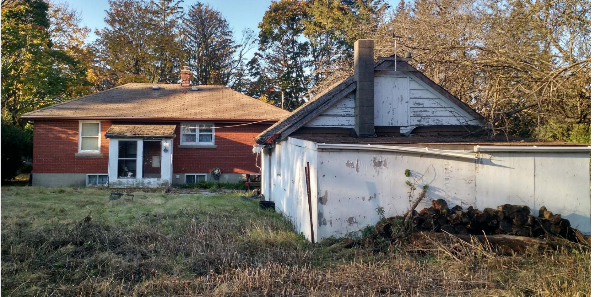
View from the back of the property, looking South West. The garage addition is deteriorating, with peeling paint and a broken eavestrough
