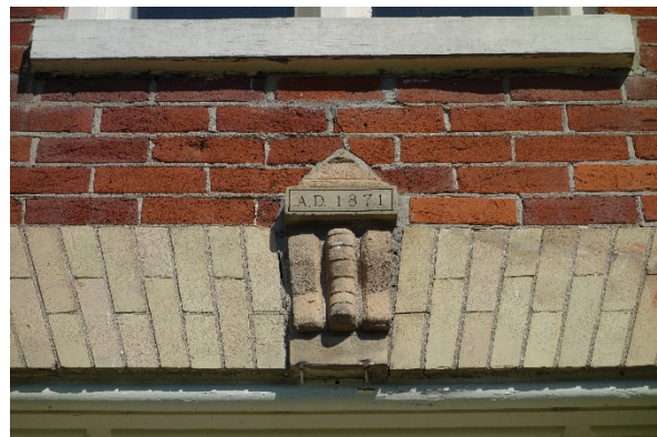
Plate 17: Flat arch structural head and keystone with 1871 date plaque on the front façade
