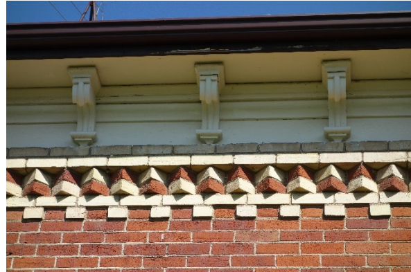
Plate 13: Brackets, moulded frieze imbrication, and dentils along the front façade roofline
