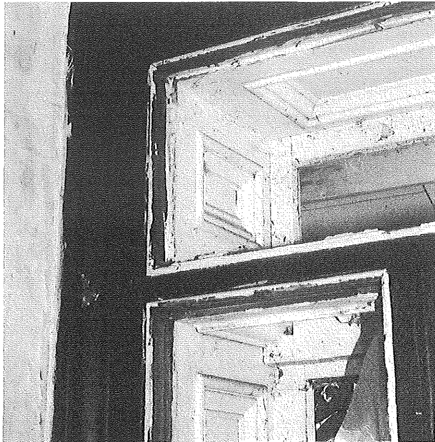
Figure 5 – Bolection mouldings at Front Door recess, with later screen beyond
