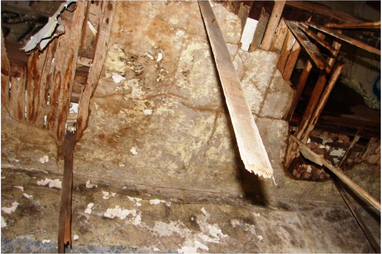
#20 – Living Room ceiling; hand split lath on left, machined made lath on right
