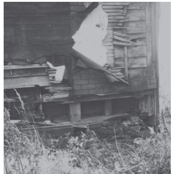
Figure 3.16 Britannia Farmhouse. NW corner showing timber construction & multiple claddings. 1987.
