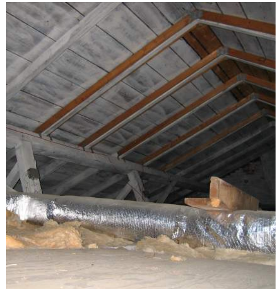
Figure 4.31 Attic showing ridgeless roof structure & reinforcing from 1990 renovation. 2009.
