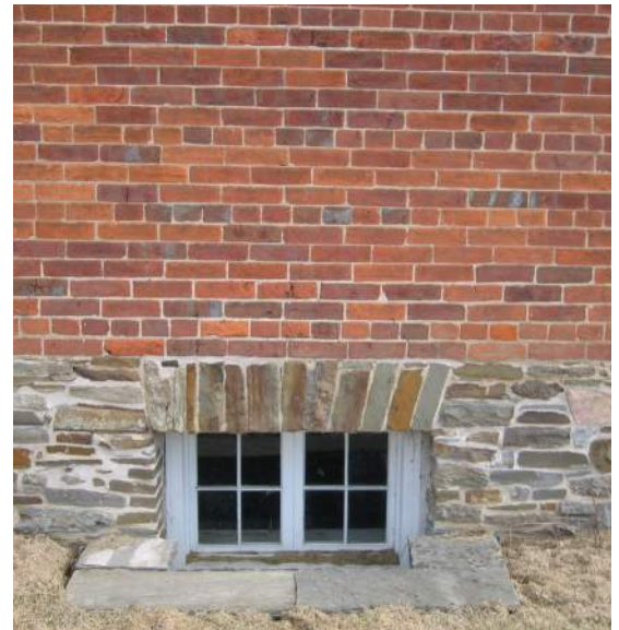
Figure 4.26 Dunton House. Early Ontario Modular red brick. 2009.
