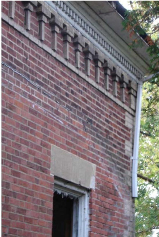
Fig. 11 – Brick cornice, east elevation
