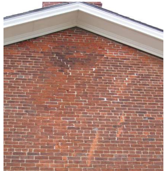
Figure 4.37 South wall showing brick deterioration. 2009.
