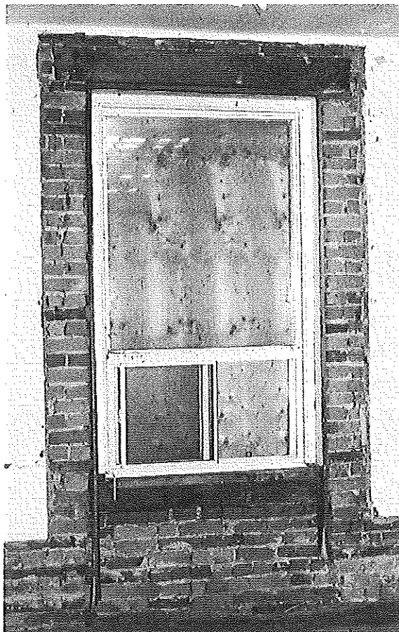
Figure 14 – Parlour, east wall: window recess and witnesses of lost baseboards and casings
