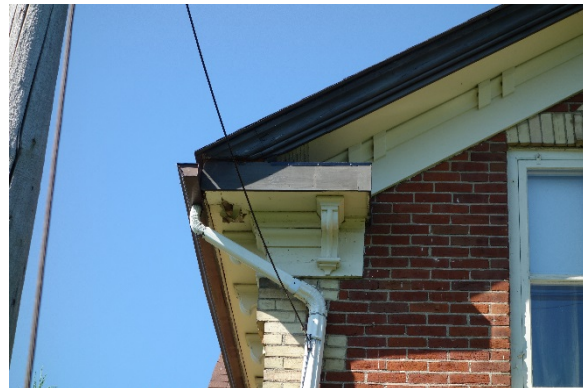
Plate 26: Returned eaves with brackets on the north elevation
