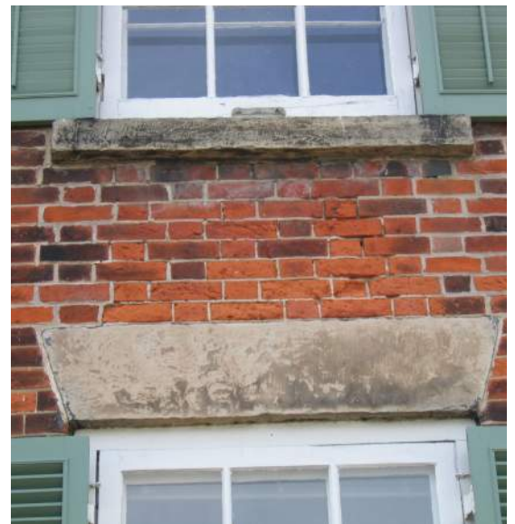
Figure 4.38 East wall showing brick deterioration. 2009.
