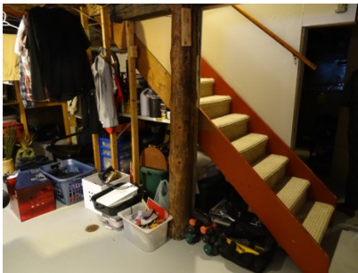
Remnent Pole Column in Basement
