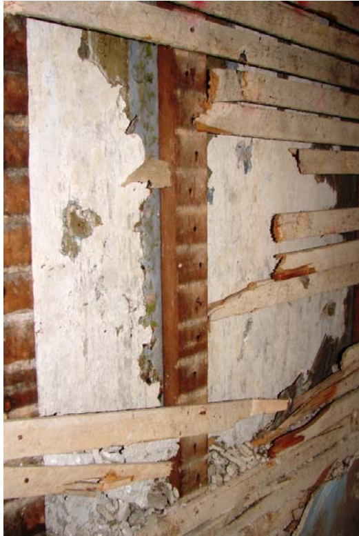
Fig. 17 – Strapping over original plaster with wallpaper beneath.
