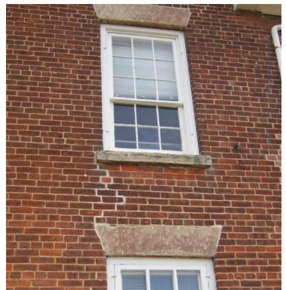
Figure 4.39 North wall showing brick deterioration. 2009.
