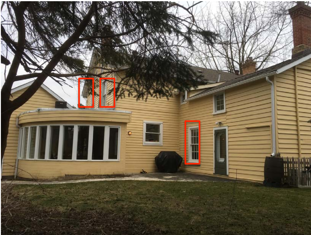
Side elevation – Repair of 3 original 6.6 wood windows – installation of 3 new 1/1 wood storms
