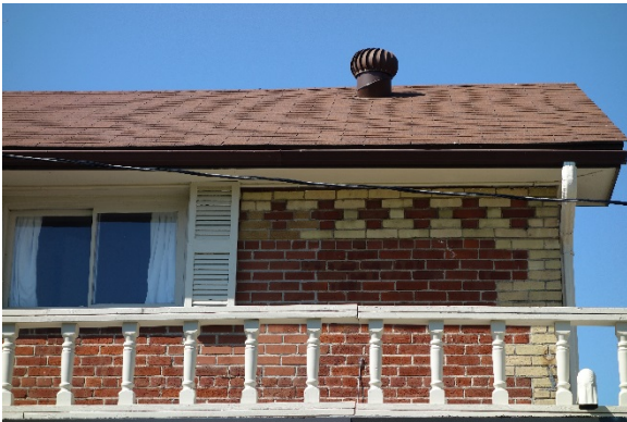
Plate 29: Dichromatic brickwork and quoins on the rear section of the north elevation
