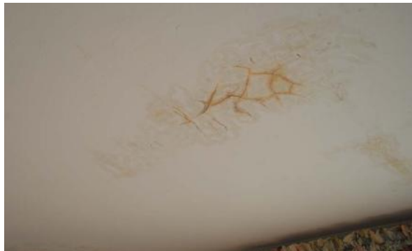
Ceilings show areas of water damage
