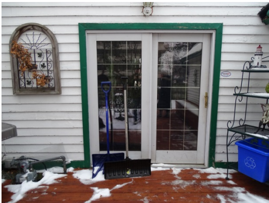
Metal Clad Sliding Doors onto Deck
