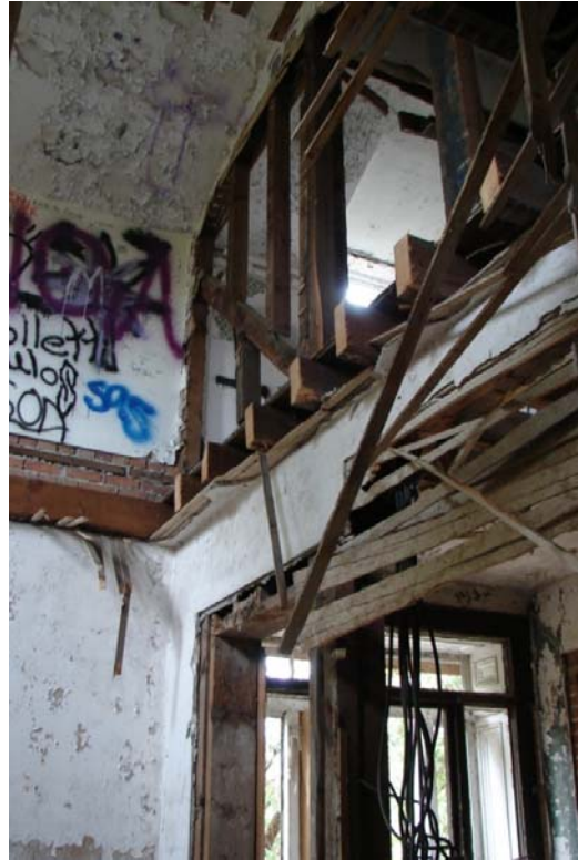
Fig. 14 – View from Parlour up through removed floor joists. Hand split lath is also visible.
