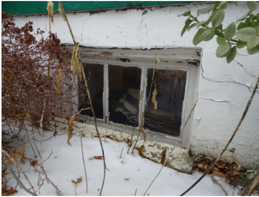
Exterior Foundation Showing Heavy Parging at Side
