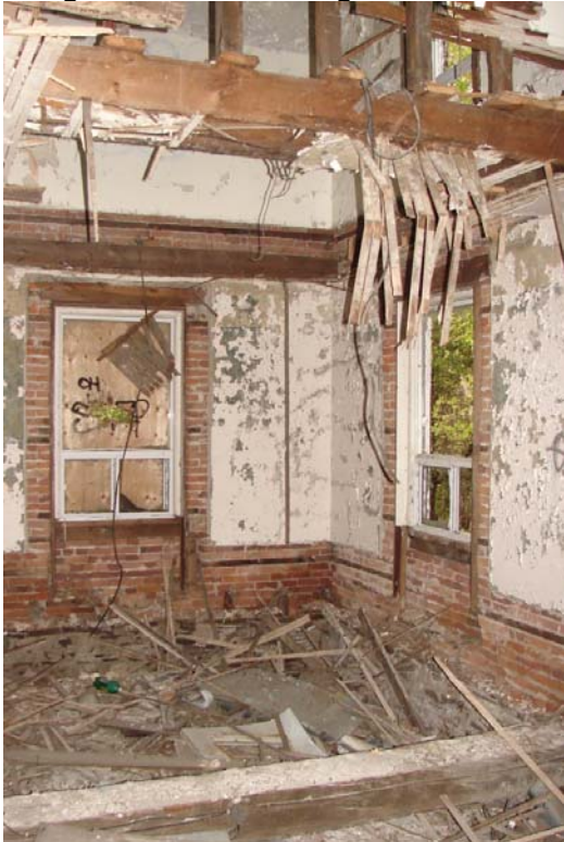
Fig. 13 – Front Hall looking east. Note line of stair stringer removed from right hand wall.
