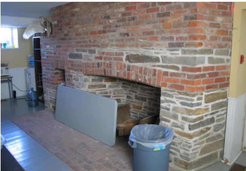
Figure 4.36 Dunton House. Basement interior showing rebuilt hearth and bakeoven. 2009.
