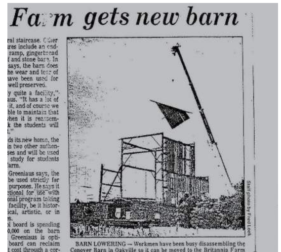
Figure 2.14 Barn Disassembly.
