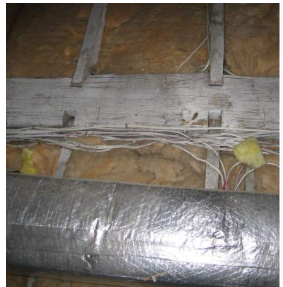
Figure 4.33 Displaced ceiling joists at north hall bent. 2009.
