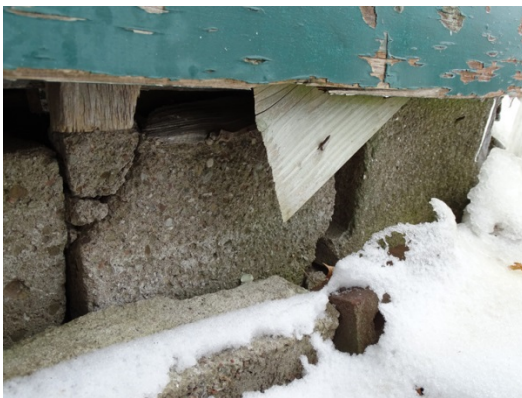
Failed Block Foundation Wall Under Porch
