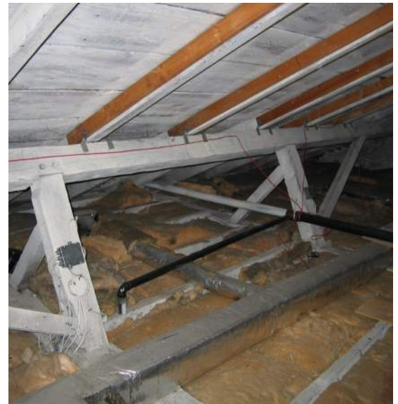
Figure 4.32 Purlins - bearing to hall structural bents. 2009.
