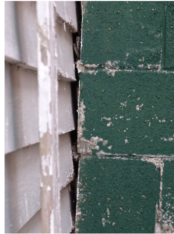
Gap Between Chimney and Siding
