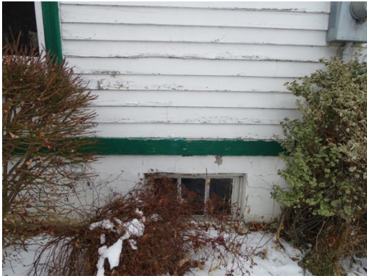
Horizontal Wood Main House Siding
