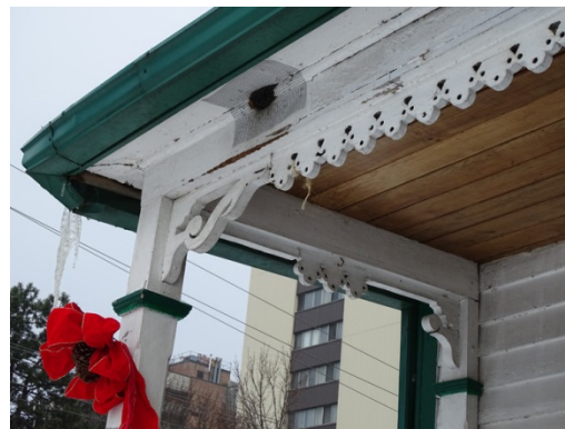
Post , Corner Bracket and Gingerbread Trim.
