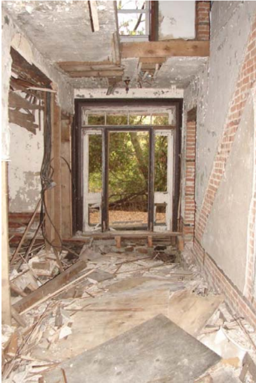
Fig. 13 – Front Hall looking east. Note line of stair stringer removed from right hand wall.
