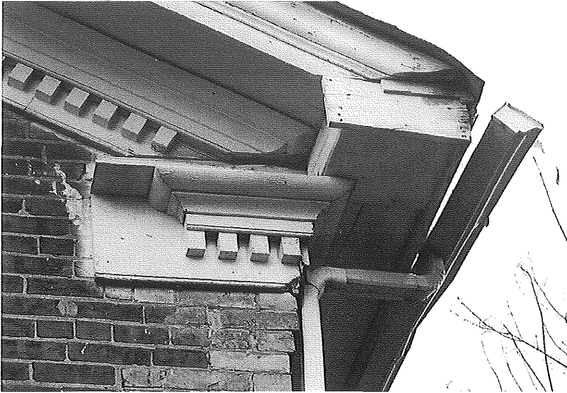
Figure 7 – Southeast corner: trim details, missing fascia returns and paint witness of gutter (?)
