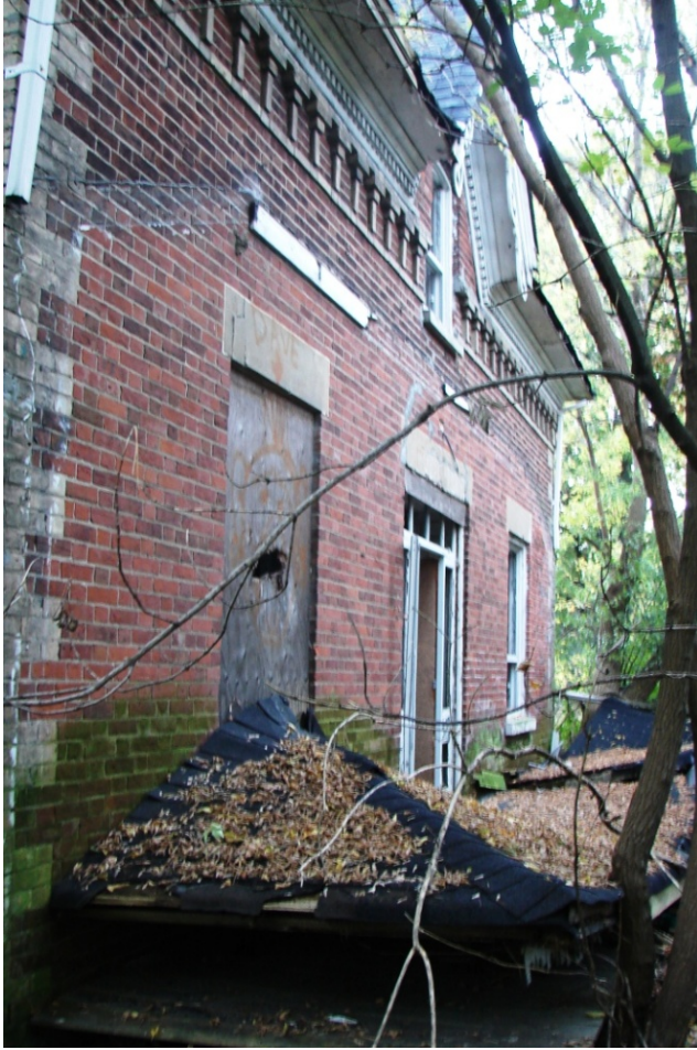
Fig. 4 – East Elevation as found October 10, 2012; note collapsed Porch
