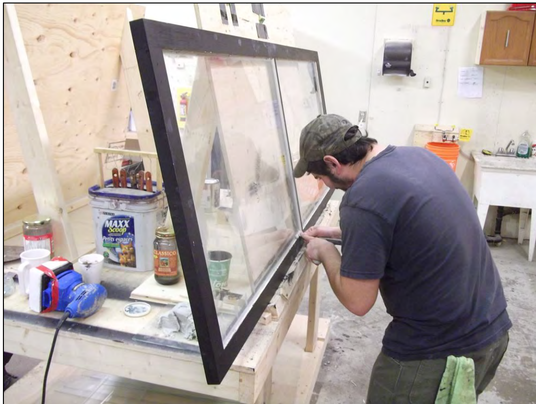
Glass installed with glazing points and Sarco putty
