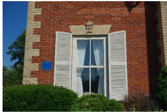
Plate 21: First storey window on the front façade showing flat structural opening, radiating voussoirs, key stone, and shutters
