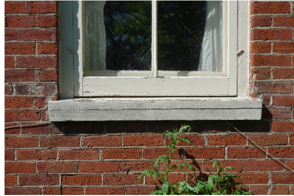
Plate 28: Window on the north elevation showing wood lugsill and wood window frame
