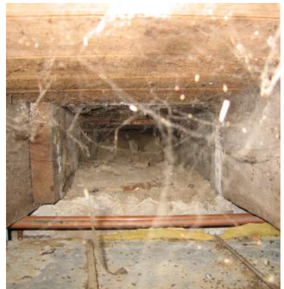
Figure 3.27 Britannia Farmhouse. Floor joists on earth. 2009
