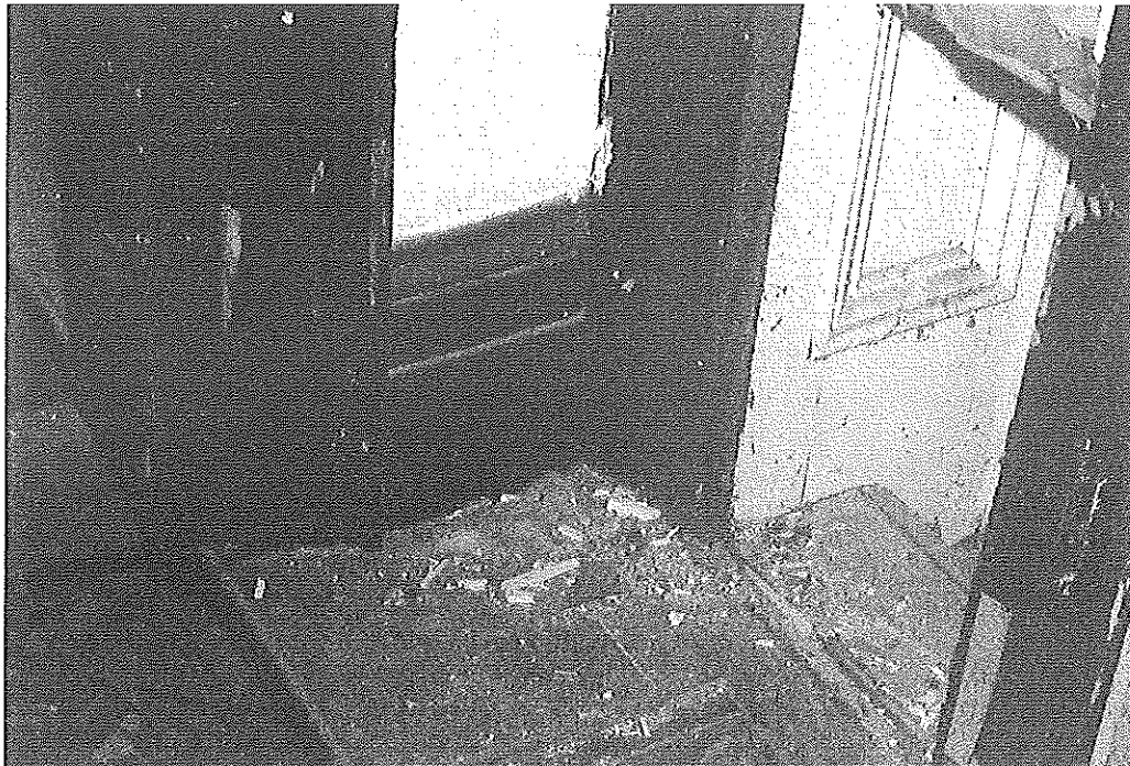
Figure 15 – Front Hall, northeast corner: baseboard, casings and door recess panelling
