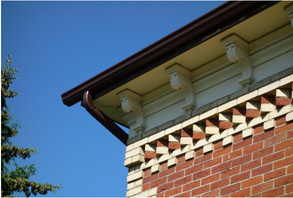
Plate 12: Projecting eaves with brackets, on the front façade
