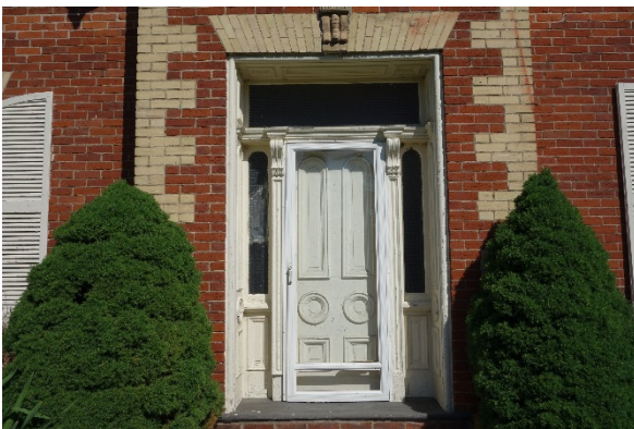
Plate 16: Front entryway showing buff brick, flat arch with keystone, and decorative door frame with transom, sidelights, and moulding
