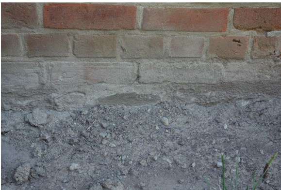
Plate 36: Stone foundations, visible on the south elevation
