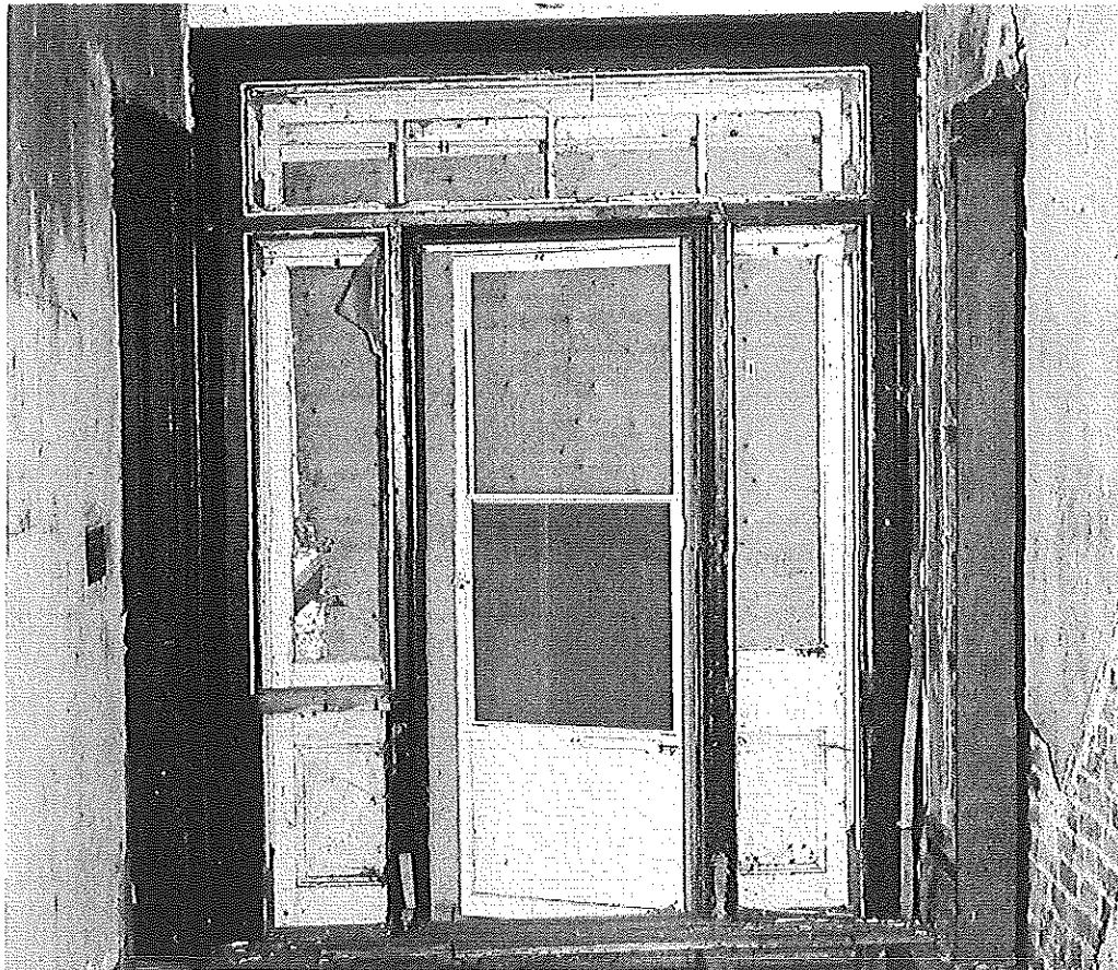
Figure 4 – Front Doorway, with later (exterior) panels and transom window
