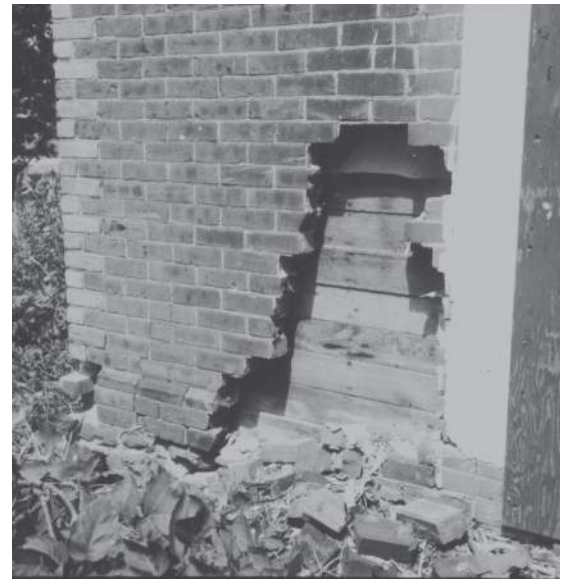
Figure 3.15 Farmhouse. Masonry veneer with nail ties. 1987.
