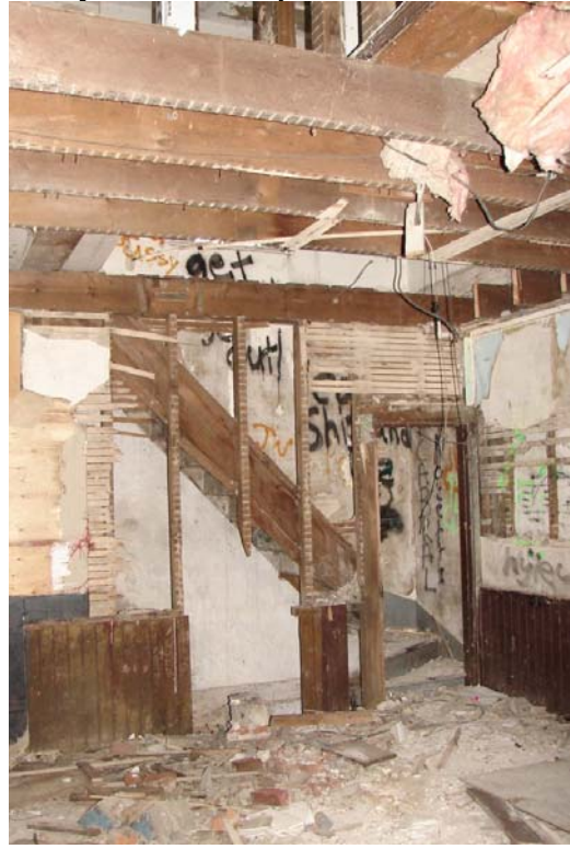
Fig. 14 – View from Parlour up through removed floor joists. Hand split lath is also visible.
