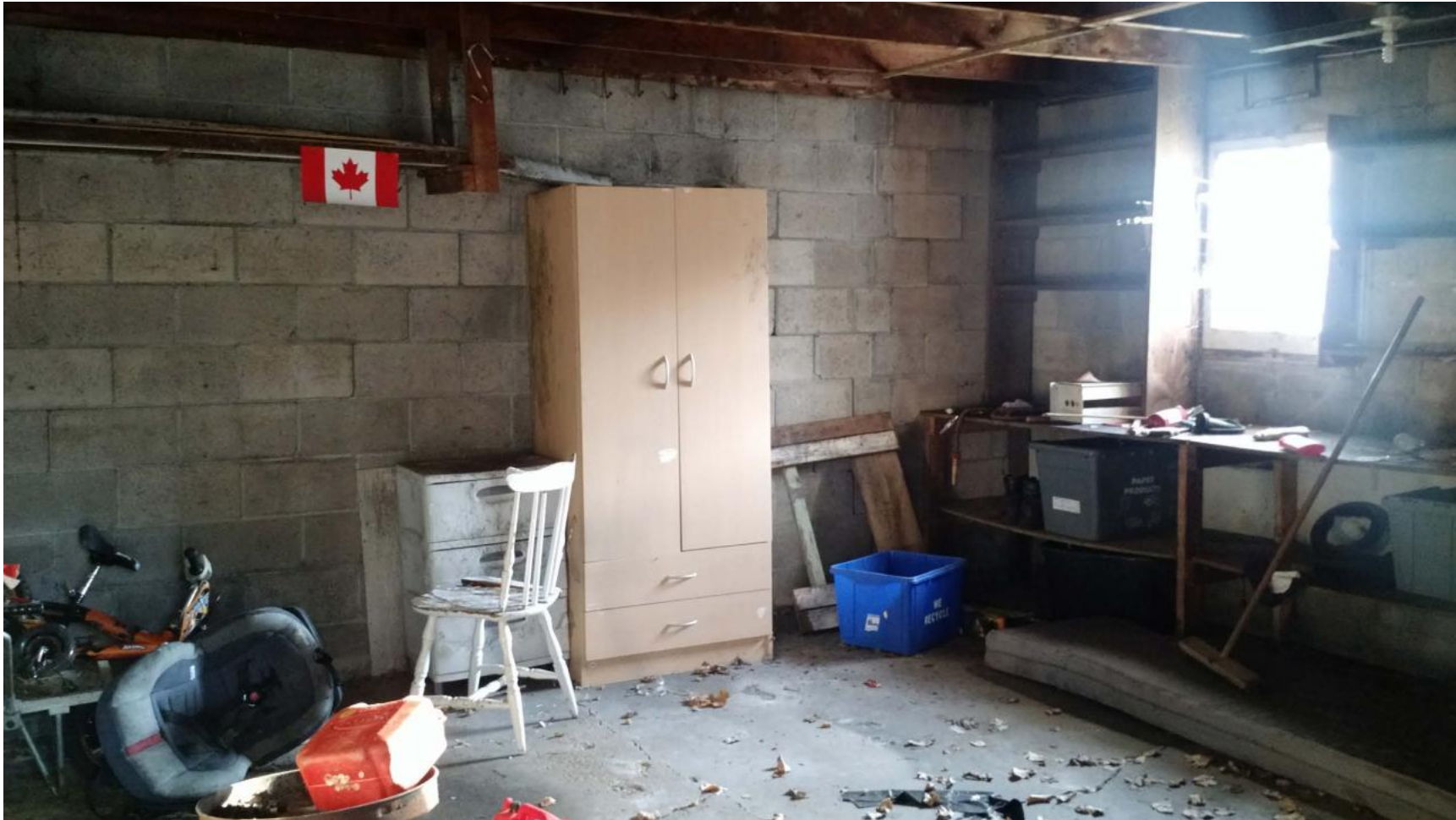
Interior view of the Garage - North East and South East Walls. The concrete floor contains cracks and water damage.
