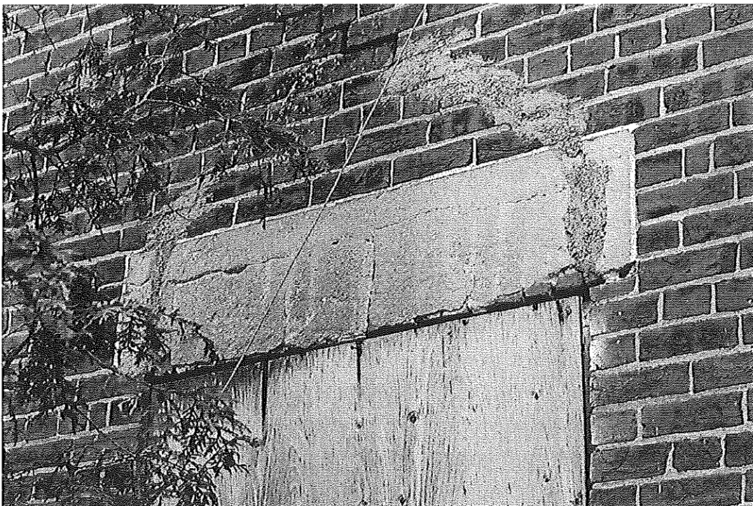
Figure 6 – South elevation, ground floor - rendered flat arch (with crude repair)
