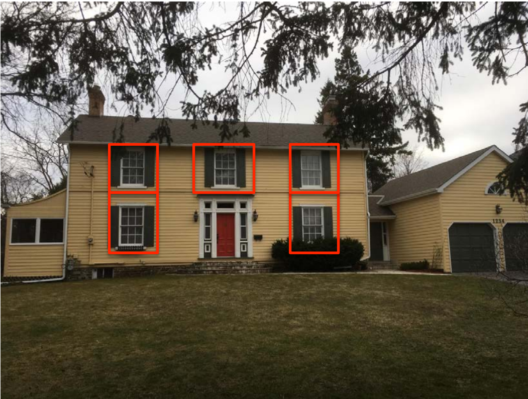
Main elevation – repairs of 5 original 6/6 wood windows – installation of 5 new 1/1 wood storms
