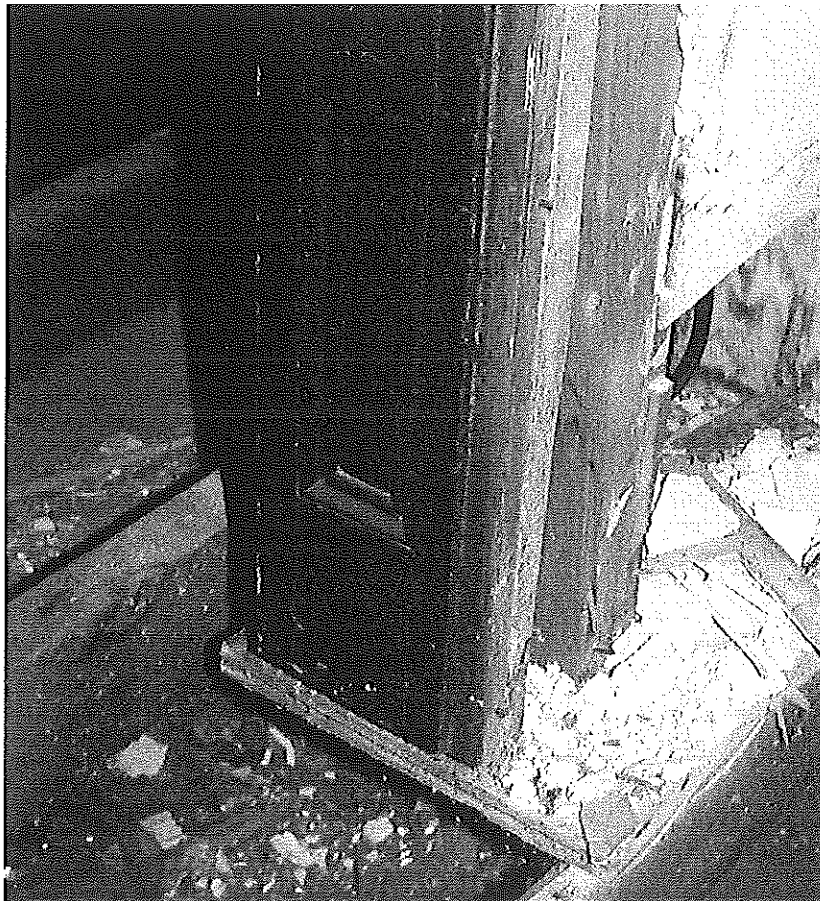
Figure 16 – Dining Room doorway: fielded panel and stud partition built off floorboards
