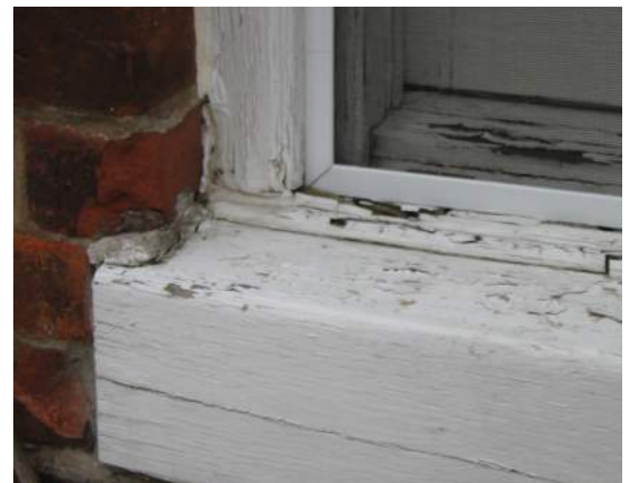
Figure 3.22 Britannia Farmhouse. Rotting sill. 2009.
