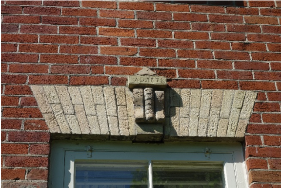
Plate 27: Buff brick structural window head with flat-arch radiating, voussoirs and carved keystone with 1871 date
