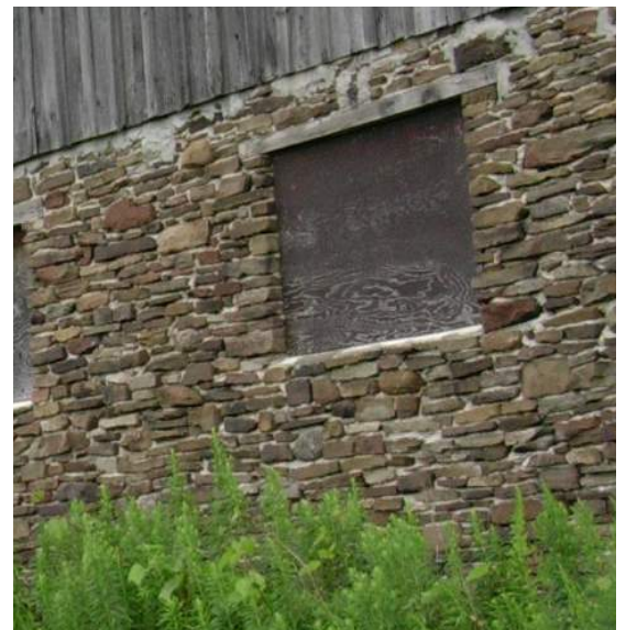
Figure 8.11 Conover Barn. Foundation veneer.
