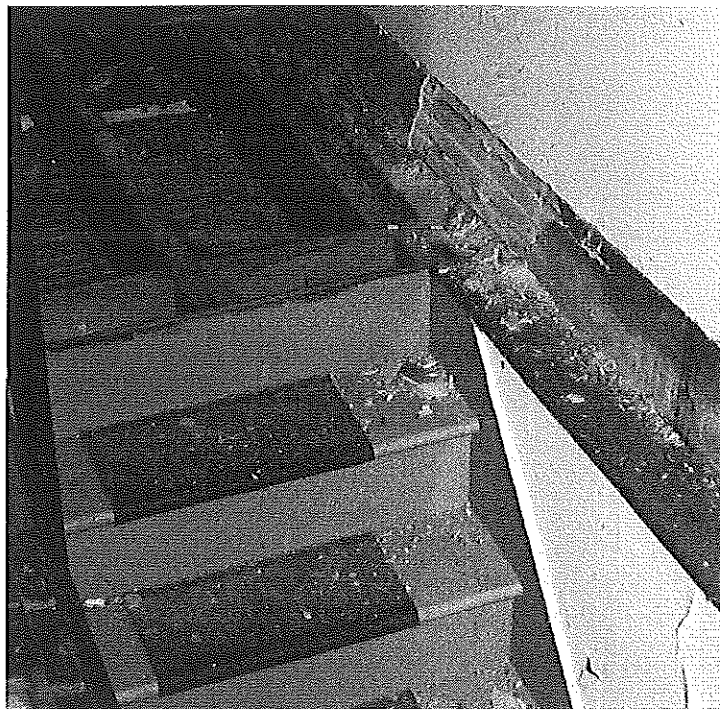
Figure 8 - Top of back stairs, showing reduction in brick wall thickness
