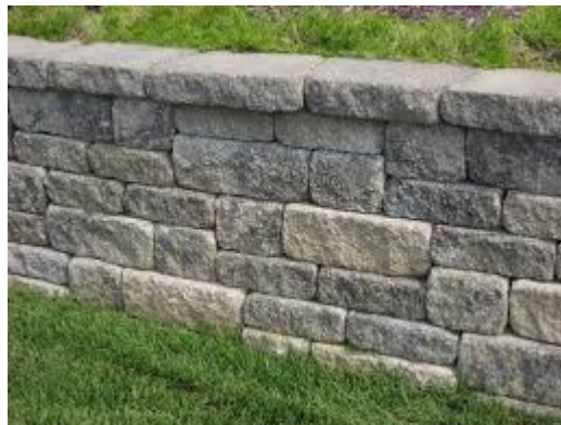
TYPICAL DRY-LAID RETAINING WALL WITH NATURAL STONE APPEARANCE
