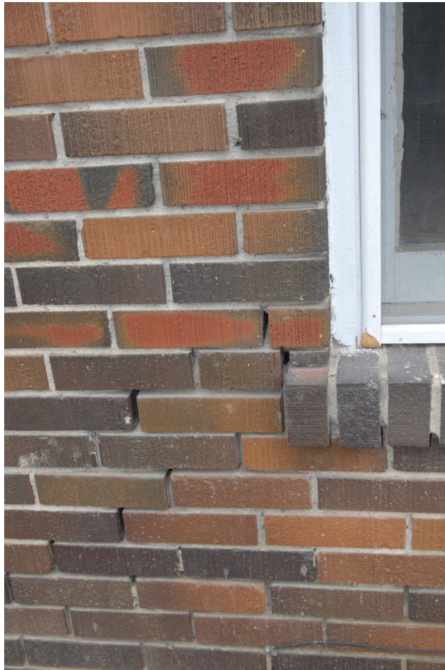
BRICK FINISH – NOTE “RUG” BRICK, MISSING MORTAR
