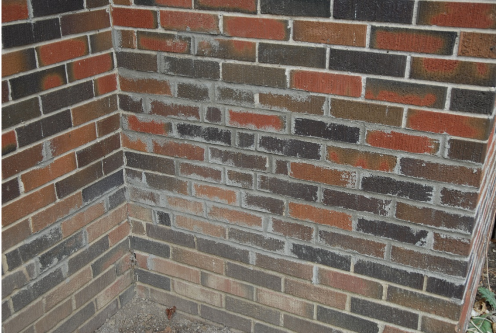
POOR BRICK REPAIR – MORTAR NOT MATCHING, SMEARED ON FACE OF BRICK
