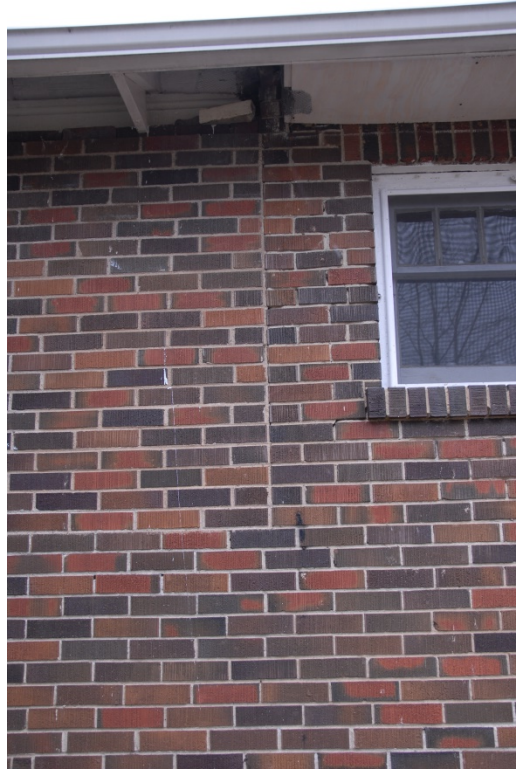
WEST ELEVATION - TRANSITION AT FORMER OPEN PORCH - NOTE DIVISION AT BRICK, DIFFERENT SOFFIT CONDITIONS, ANIMAL ENTRY HOLE IN SOFFIT
