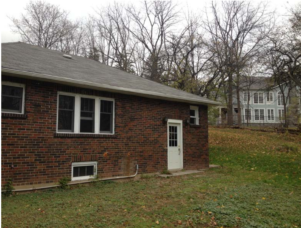
PARTIAL WEST ELEVATION - NOTE HIGH GRADING CONDITIONS AT REAR OF EXISTING HOUSE
