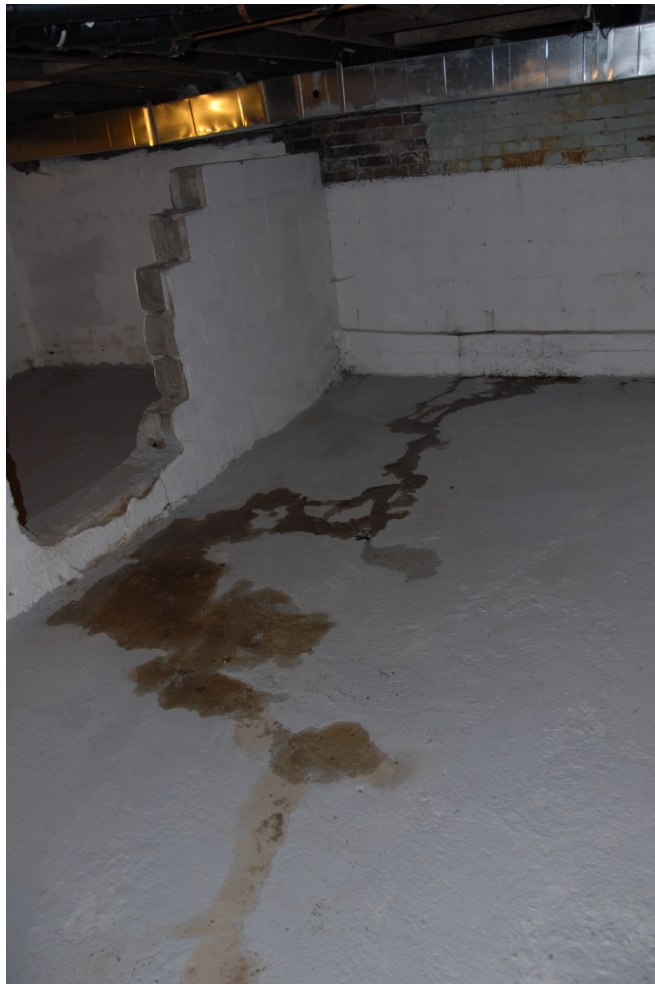
BASEMENT - NOTE STAINING, STANDING WATER
