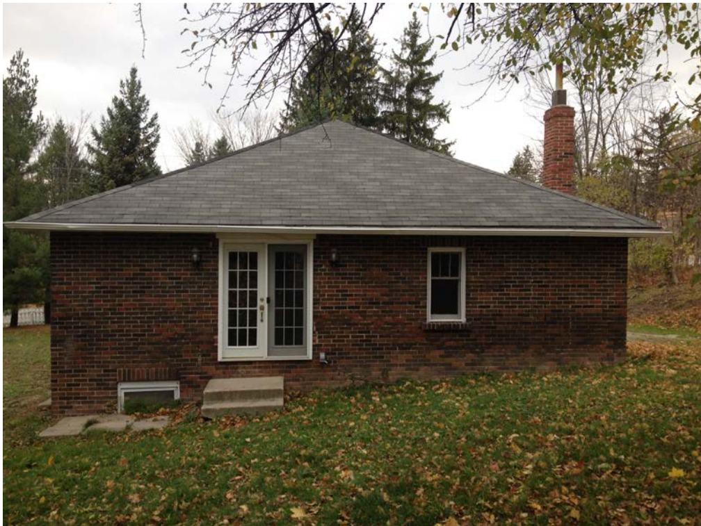
REAR ELEVATION - NOTE SLOPING GRADE CONDITION, AWKWARD STEP AT REAR EXIT
