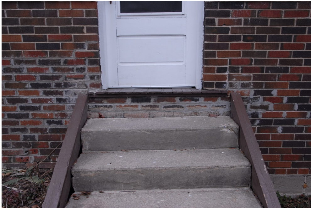
POOR BRICK REPAIR AT FRONT STEPS
