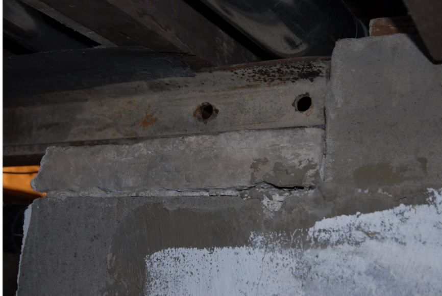
BASEMENT – RE-PURPOSED STEEL RAILROAD TRACK USED AS BEAM - NOTE POURED CONCRETE FILLER AT BEARING POINT - THIS MAY HAVE REPLACED AN EARLIER WOOD BEAM
