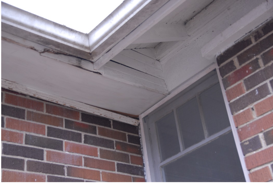
TYPICAL SOFFIT - NOTE TRANSITION OF OPEN AND CLOSED SOFFIT, POOR DETAILING, POOR CONDITION
