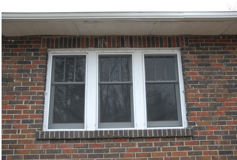
WEST ELEVATION, NOTE ORIGINAL GANGED WINDOWS, BRICK VOISSIORS AND SILLS, OVERALL POOR BRICK CONDITION, POOR SOFFIT CONDITION AND DETAILING
