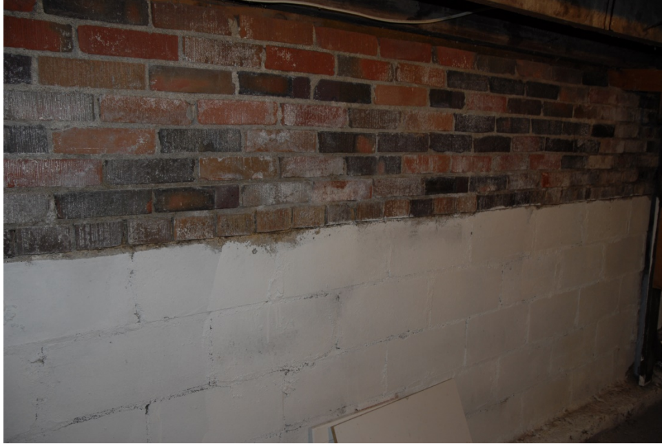
BASEMENT BLOCK/BRICK WALL - NOTE MOISTURE PENETRATION AT BRICK – THIS IS LIKELY CAUSED BY IMPROPER GRADING
