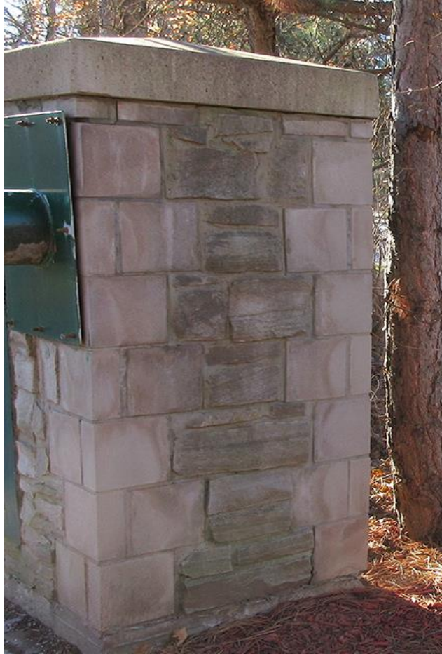
Detail of kiosk construction: smooth and rusticated stone and cast concrete coping stone roof
