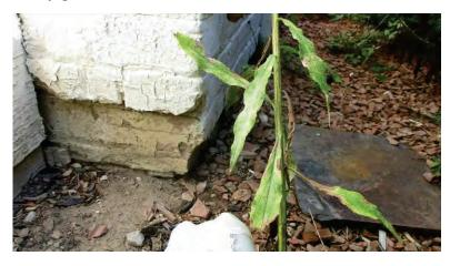
Figure 4: Deteriorated coatings near grade
