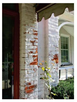
Figure 5: Deterioration on south side of entry canopy
