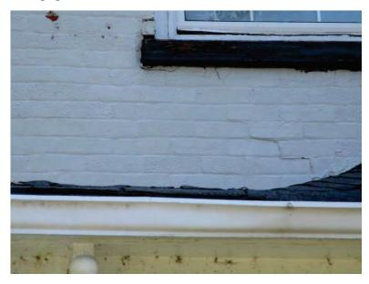
Figure 7: Step cracking below second storey window
