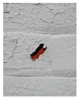
Figure 3: Soft brick exposed below coatings
