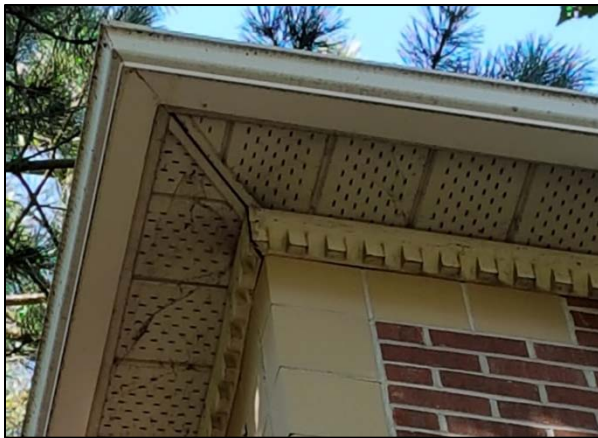
Figure 28: Dentil cornice
