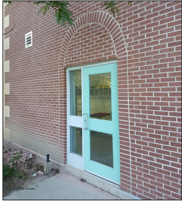
Figure 27: Brick arch above the north elevation doors
