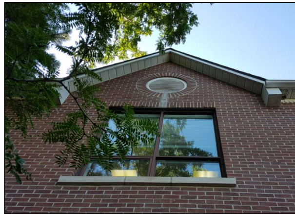
Figure 29: Gable with circular vent
