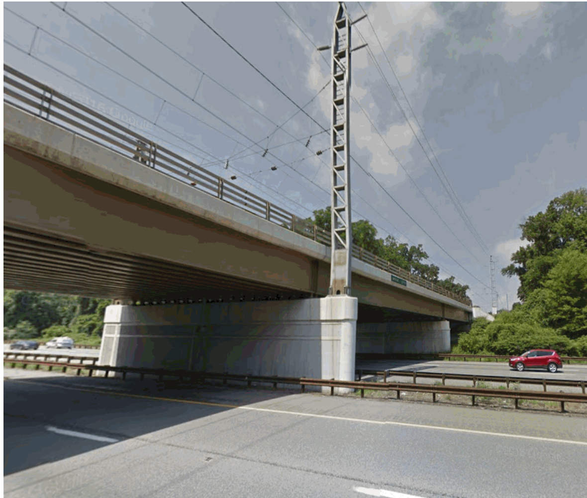
Figure 4-6: Example of anchor and bolt attachment. Source: Gannet Fleming 2017
