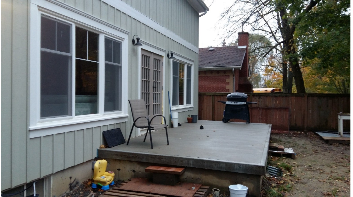
Figure 5: Side view of Concrete deck from backyard - note width of deck is less than width of house
