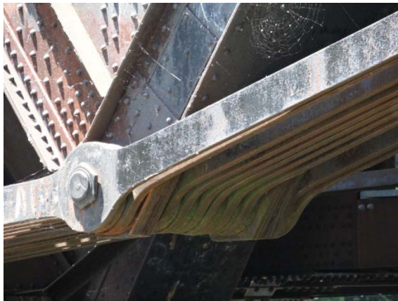
Plate 3-7: Detail of eyebar bundles
