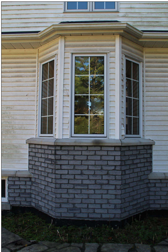
Figure 27 bay window at rear - concrete brick veneer
