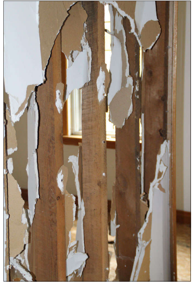
Figure 40 rough sawn, pre WW II 2" x 4" studs
