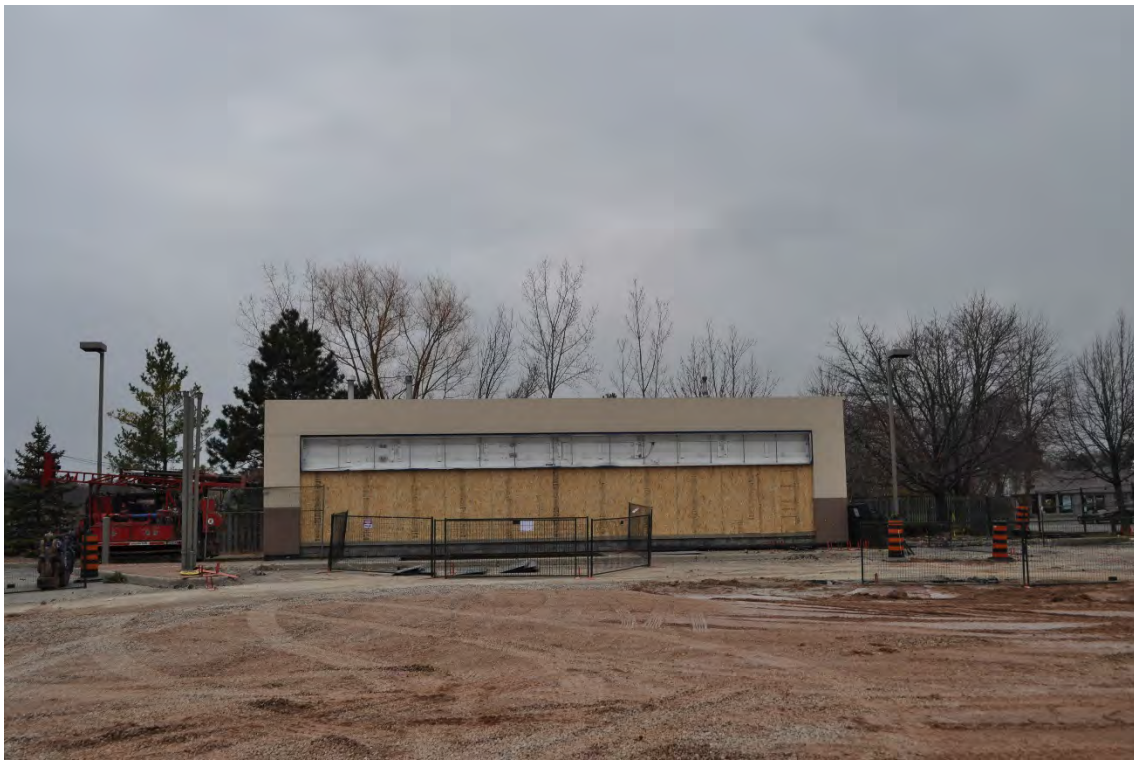
Figure 11: Car wash building, east facade (CU 2016).
