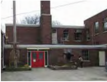
FIG 45: East elevation at east courtyard (ERA, 2016).
