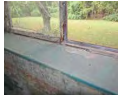
FIG 21: Painted interior masonry sill on west wall (ERA, 2016).
