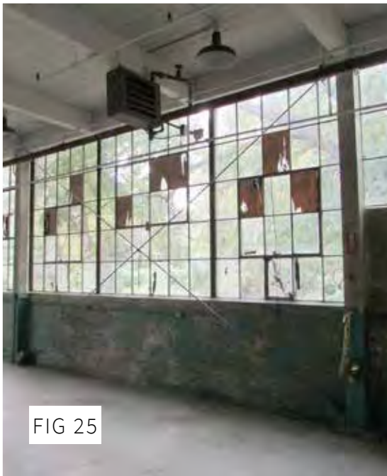
FIG 25: Steel cross-bracing between columns on the interior west elevation (ERA, 2016).
