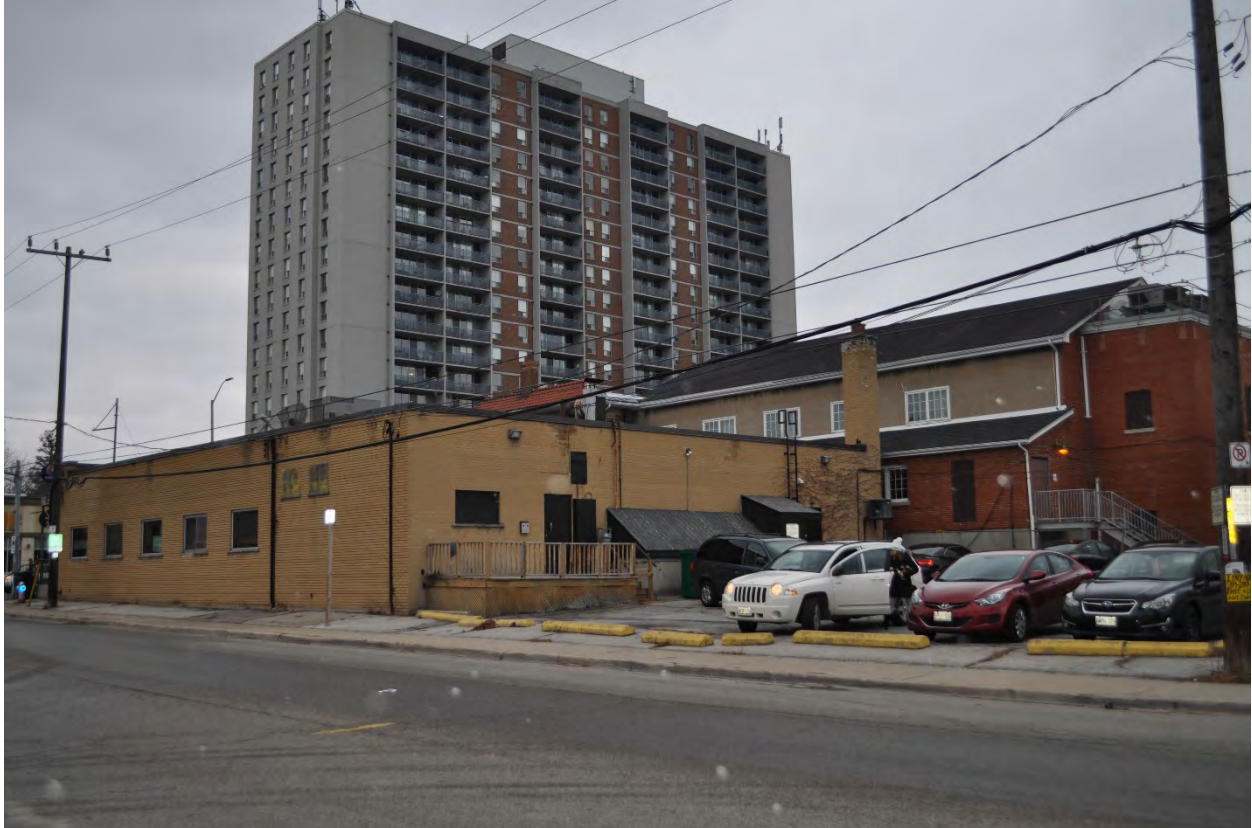
Figure 31: Rear of Clarke Memorial Hall (redbrick building) from 181 Lakeshore Road West, facing east (CU 2016).
