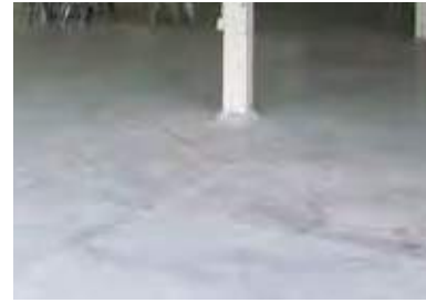
FIG 64: Concrete floor in South Building (ERA, 2016).
