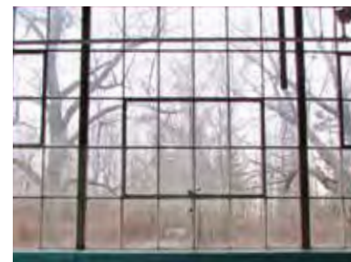
FIG 55: Typical window bay on South Building (ERA, 2016).
