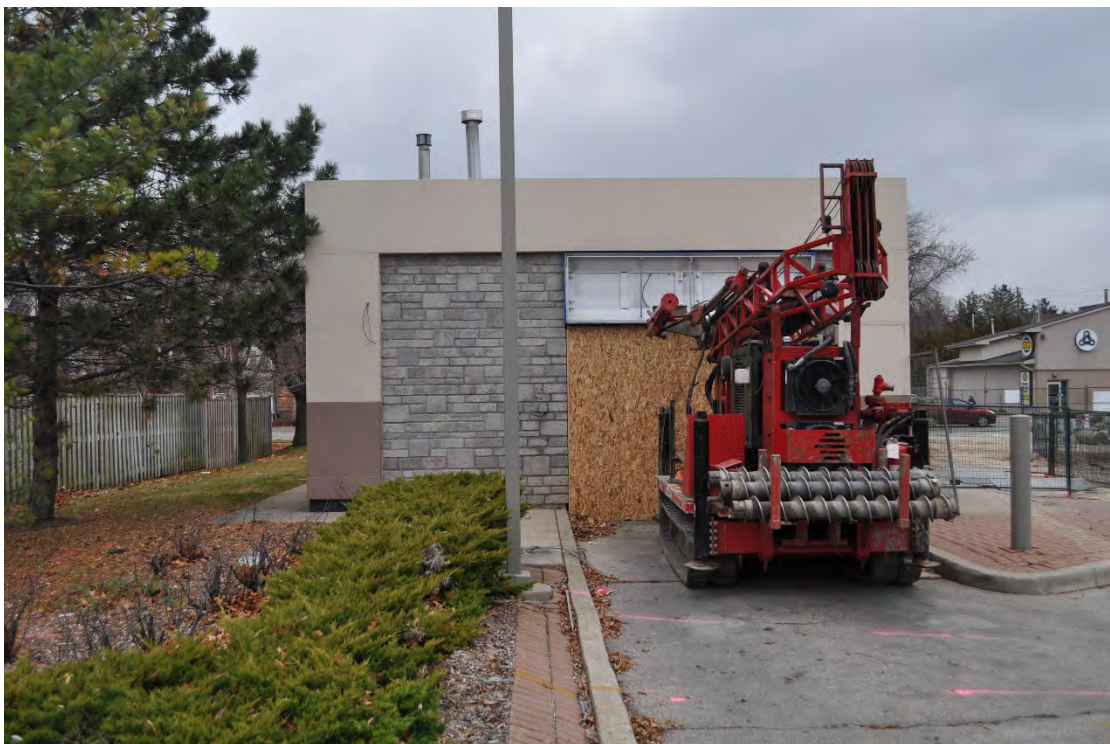
Figure 13: Car wash building, south facade (CU 2016).
