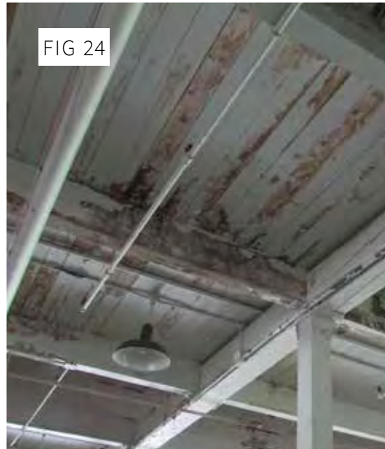
FIG 24: Condition of wood structural elements showing severe paint peeling (ERA, 2016).
