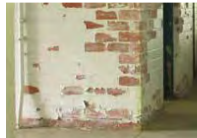
FIG 66: Painted hollow-core brick wall (ERA, 2016).
