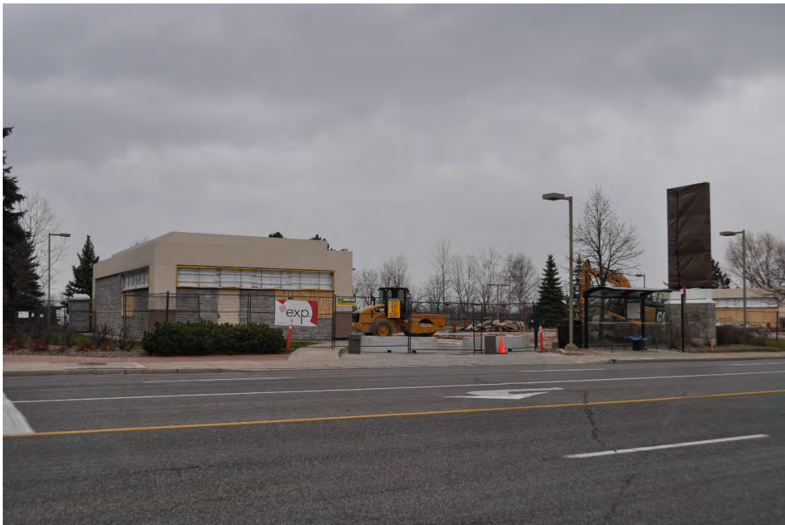
Figure 5: Convenience Store building, north facade (CU 2016).
