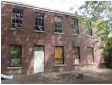
FIG 50: West elevation at west courtyard (ERA, 2016).
