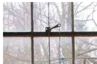
FIG 36: Interior detail of original window hardware (ERA, 2016).
