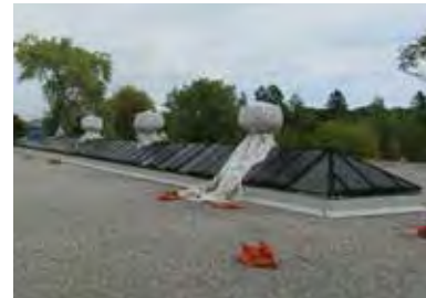
FIG 15: Large skylight showing boarding, wrapped vents, and new flashings (ERA, 2016).
