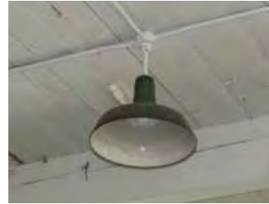
Fig 69: Original interior light fixture (ERA, 2016).
