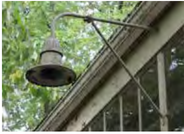
FIG 62: Existing original exterior lighting unit on the west facade (ERA, 2016).
