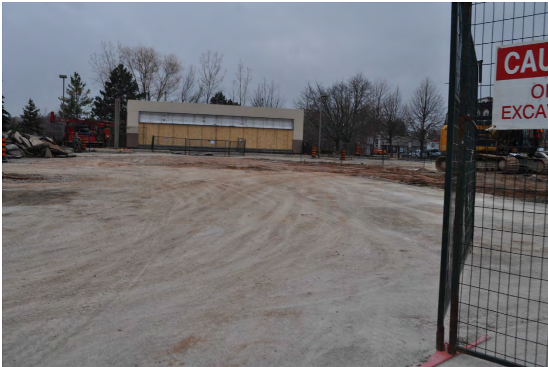
Figure 17: Property overview, facing west (CU 2016).
