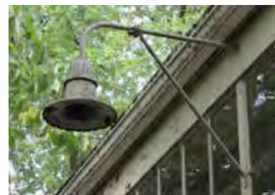
FIG 17: Existing original exterior lighting unit on the west facade (ERA, 2016).
