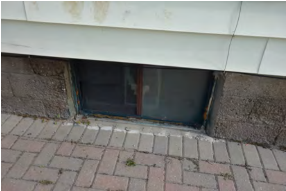
Figure 10: Raised concrete block foundation, vinyl siding and windows.
