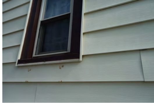
Concrete block foundation, metal windows, vinyl windows and vinyl wall cladding.
