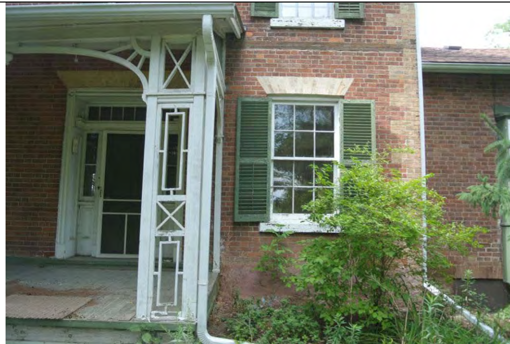
Plate 7: Detail of a representative six-over-six sash window.
