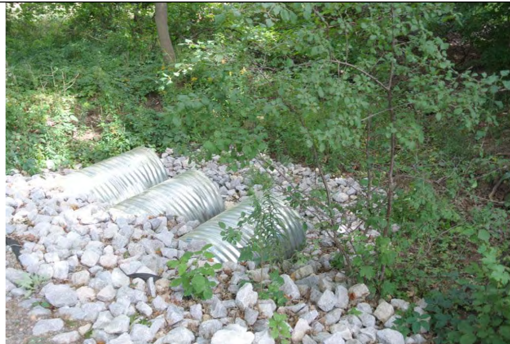
Plate 38: Detail of the three culverts passing under the gravel laneway to the east of the through truss bridge.
