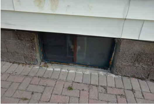
Concrete block foundation, metal windows, vinyl windows and vinyl wall cladding.
