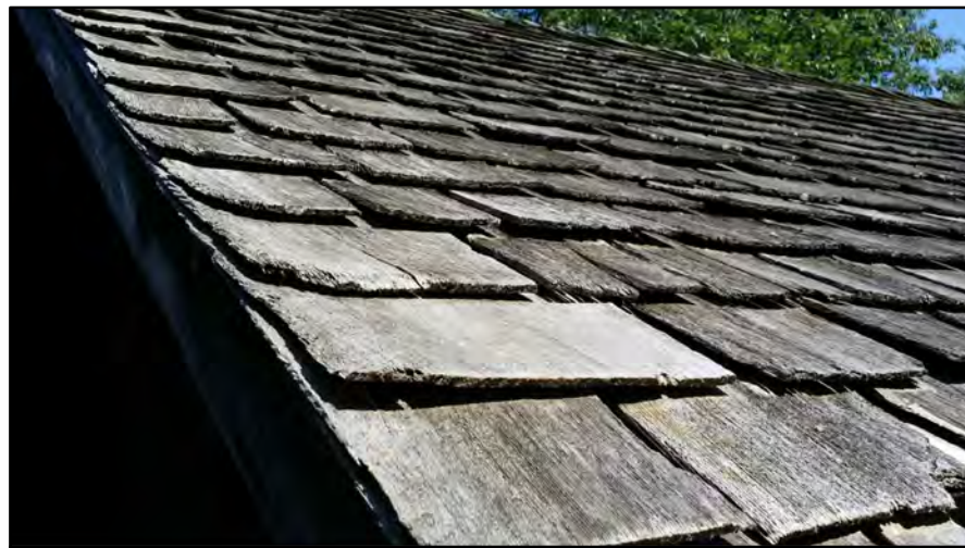
GENERAL DETERIORATION OF CEDAR SHINGLES
