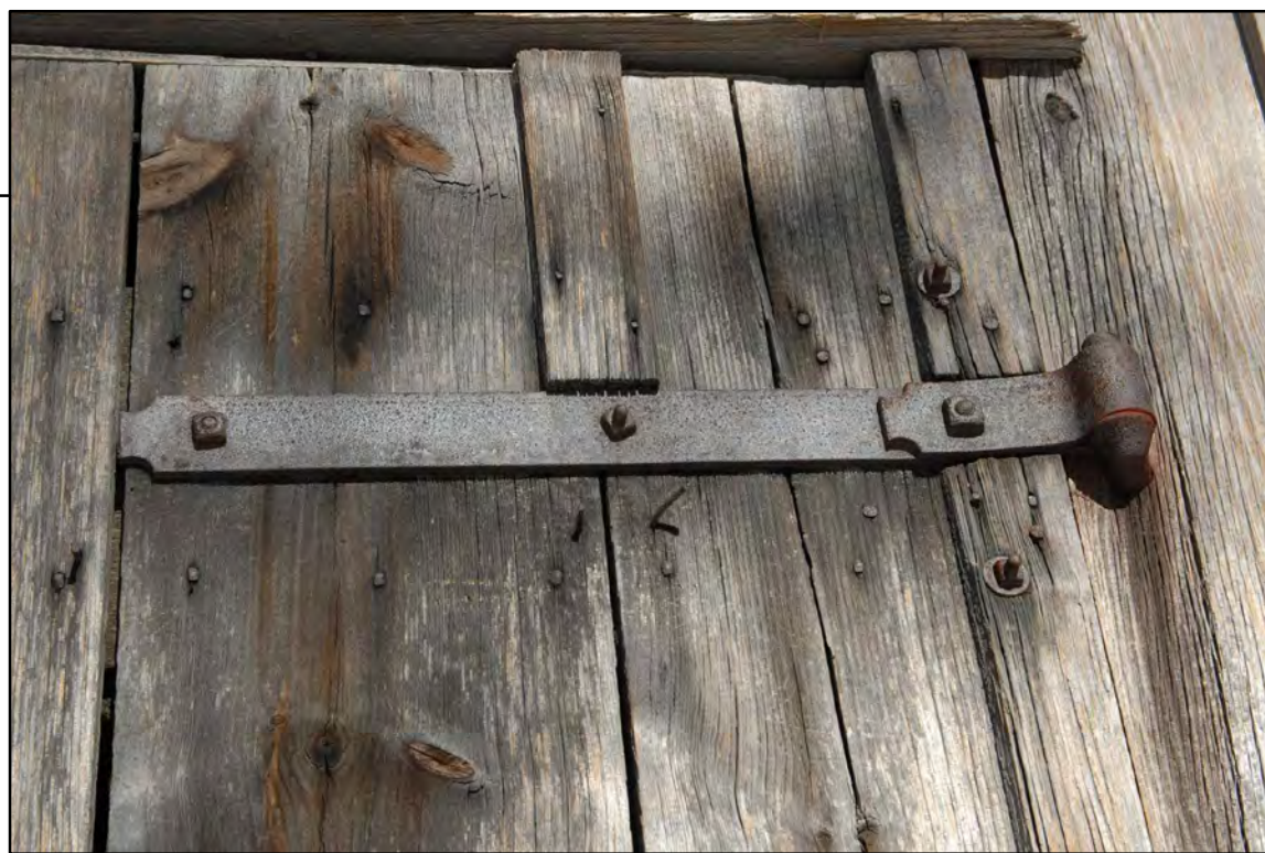
DOOR — NOTE ORIGINAL METAL STRAP HINGE AND ORIGINAL HARDWARE. THIS MUST BE CONSERVED AND RE-USED. NOTE ORIGINAL WOOD DRIP EDGE ABOVE
