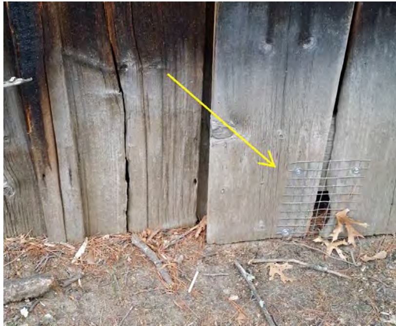
Neatly fitted wire mesh used to keep out rodents
