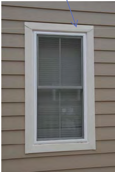
INSTALLED WINDOW WITH ALUMINUM TRIM – SIDES AND REAR
