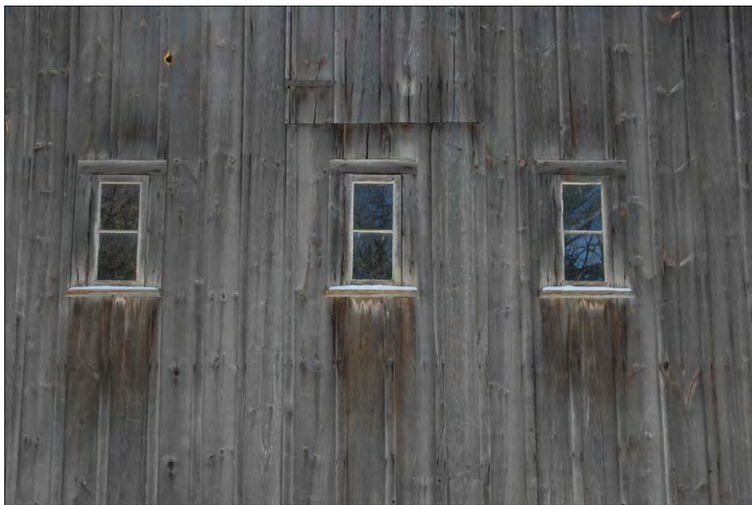
WINDOWS AT NORTH ELEVATION - ALL WINDOWS TO BE REMOVED AND SENT TO WINDOW CONSERVATOR FOR OFF-SITE RESTORATION
