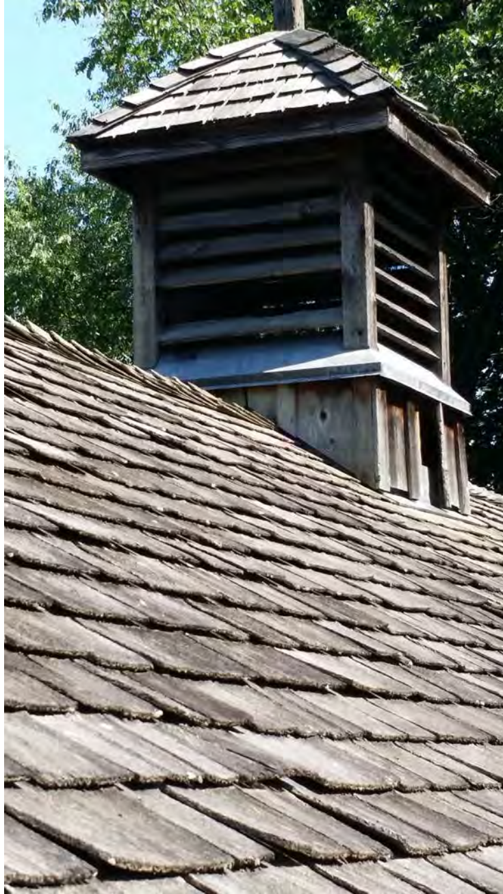
Cupola showing loose, missing pieces (note cupped, lifted shingles)
