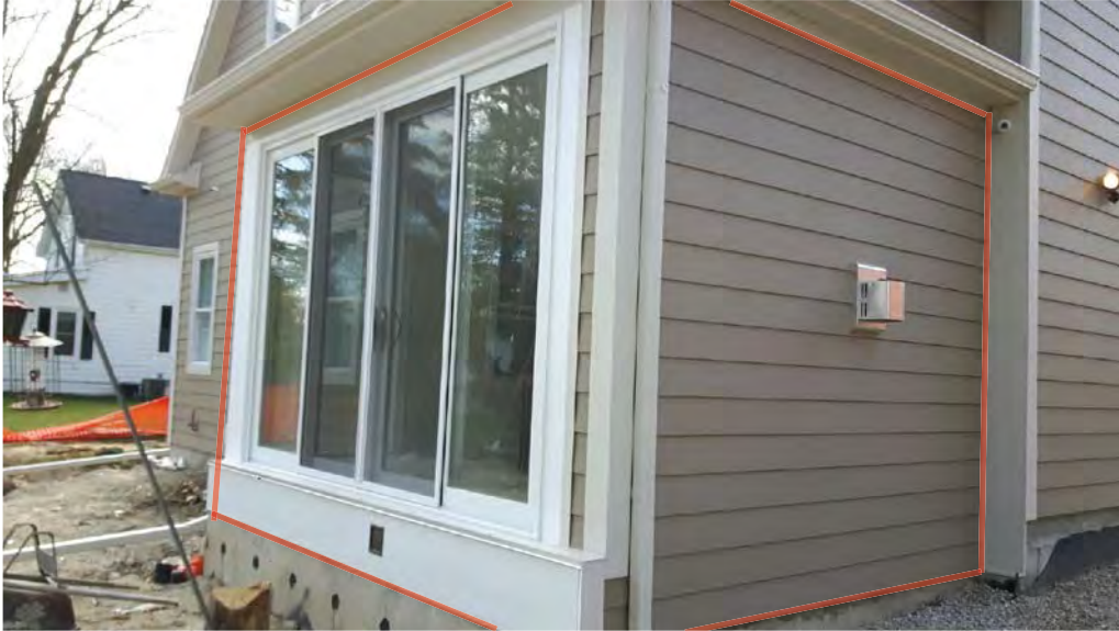
Detail of enclosed porch showing area of side elevation filled in, new sliding glass door
