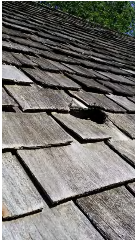
Roof showing hole in shingles
