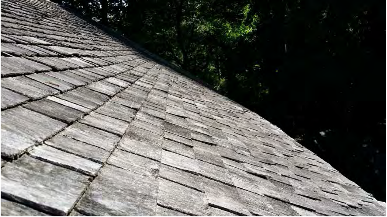
General view of roof showing deteriorated shingles
