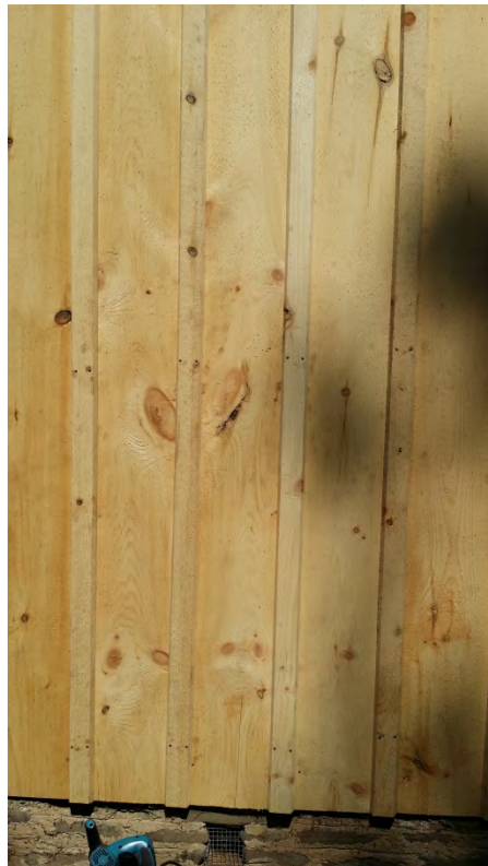
Detail of board & batten siding
