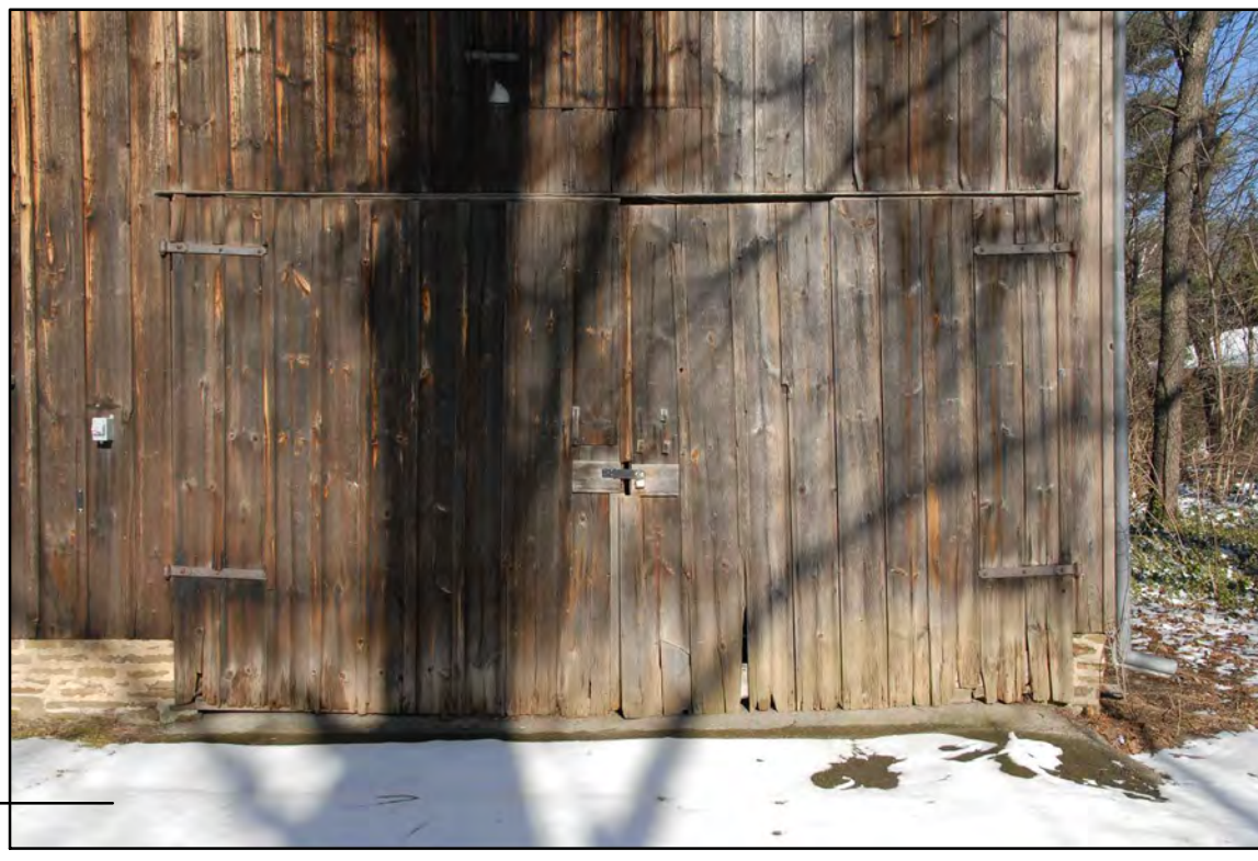
DOOR — NOTE GENERAL DETERIORATION, SAGGING OF DOOR PANELS. ALL DOORS ARE TO BE REMOVED AND ASSESSED ON-SITE AND REPAIRED ON SITE IF POSSIBLE. IF REPAIRS ON SITE ARE NOT POSSIBLE DOORS ARE TO BE SENT TO SPECIALIST FOR OFF-SITE CONSERVATION
