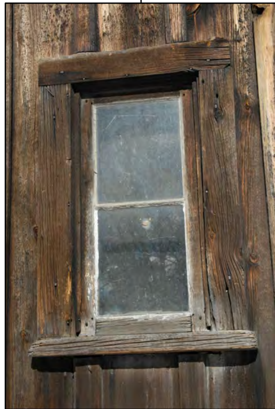
WINDOW — NOTE DETERIORATION AT LOWER SASH, SILL
