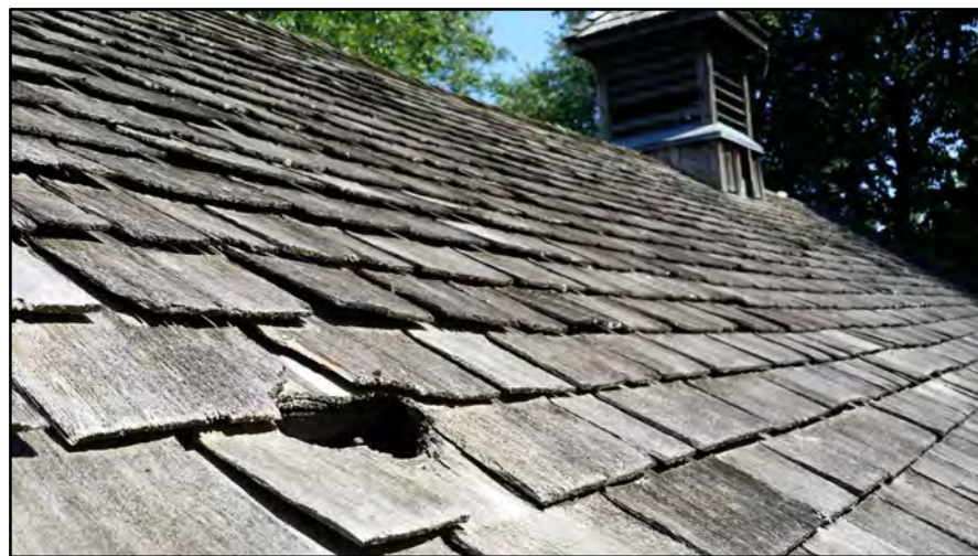
10CM HOLE IN EXISTING ROOF
