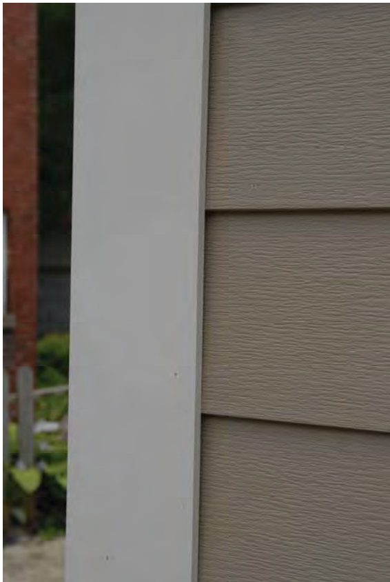
"CELECT" VINYL SIDING WITH JAMES HARDIE CORNER TRIM BOARD AS INSTALLED
