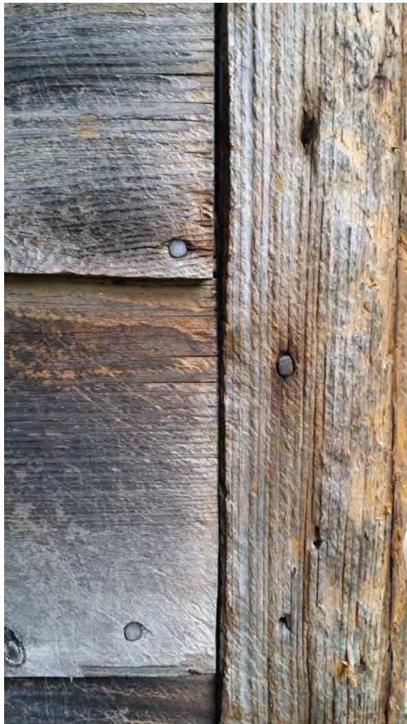
Existing siding detail showing differential nailing pattern. Horizontal siding at left fastened with newer, round galvanized nails. Vertical siding at right fastened by older, non-coated square head nail
