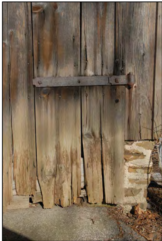
DOOR — NOTE DETERIORATION AT LOWER EDGE (TYPICAL FOR ALL DOORS)
