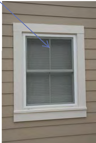
INSTALLED WINDOW WITH APPLIED WOOD TRIM – FRONT
