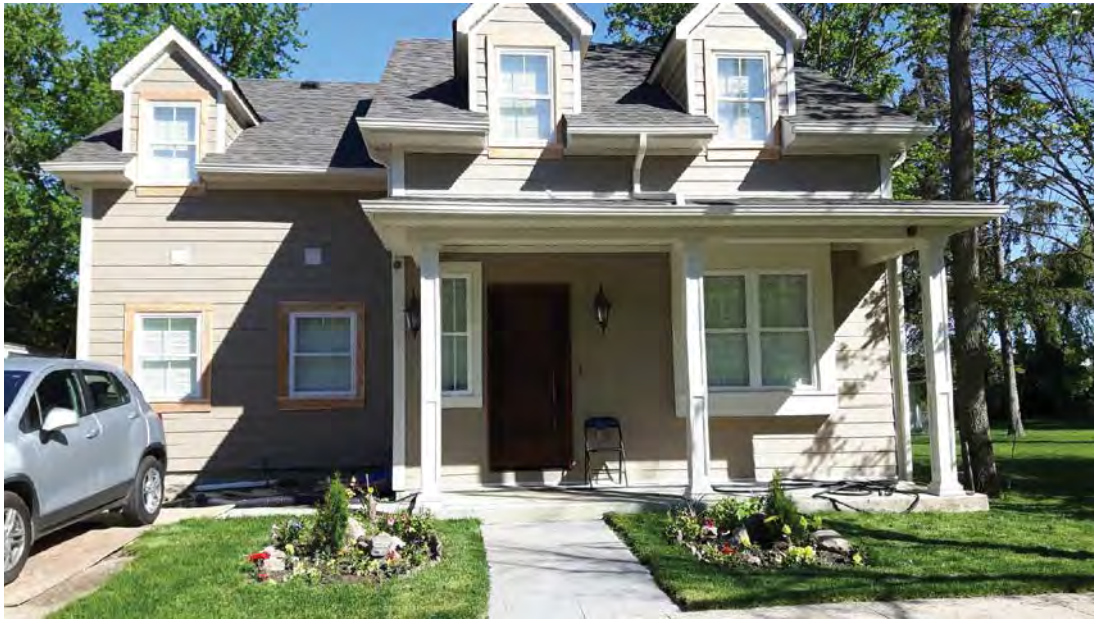
Front elevation showing vinyl siding, vinyl windows with wood trims (some not yet painted), vinyl porch columns
