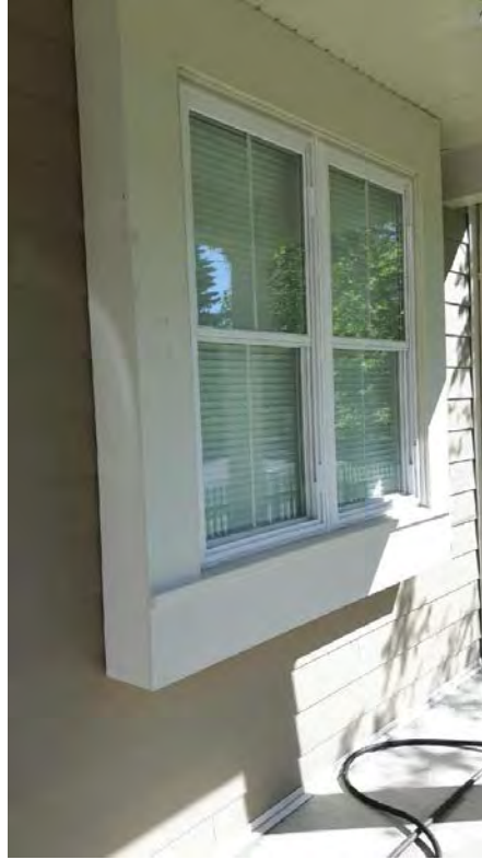
Detail of front Oriel window showing vinyl window with wood trim
