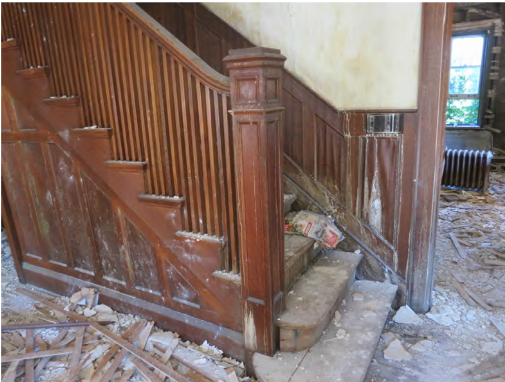
Figure 4: MAIN FLOOR - Detail of front stair newel post and hand rail
