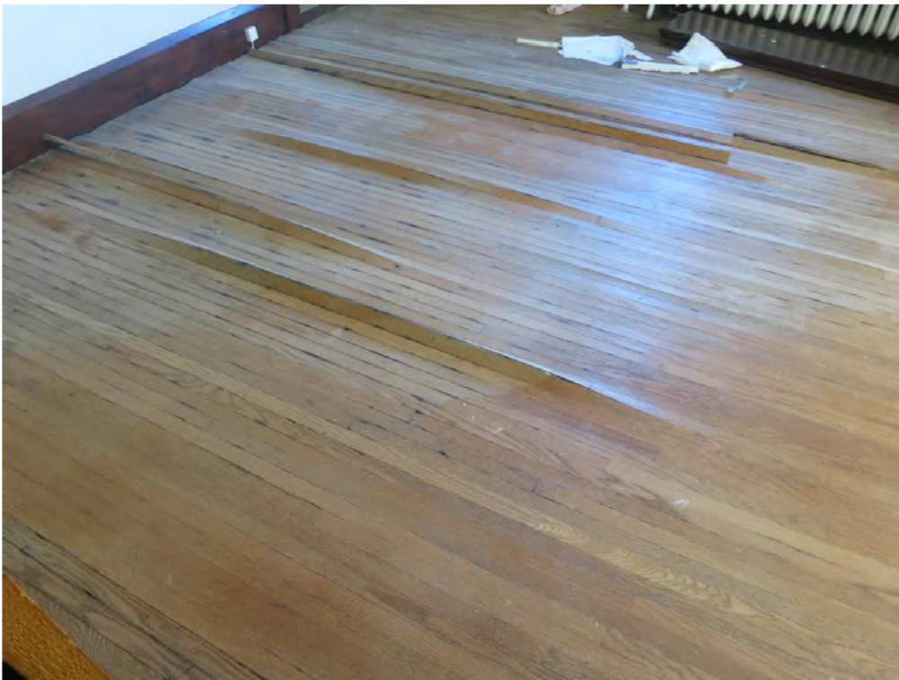
Figure 6: 2nd FLOOR - Detail showing water damaged wood flooring.
