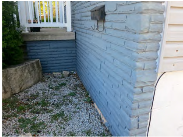
Figure 10: Raised concrete block foundation, vinyl siding and artificial stone facing.
