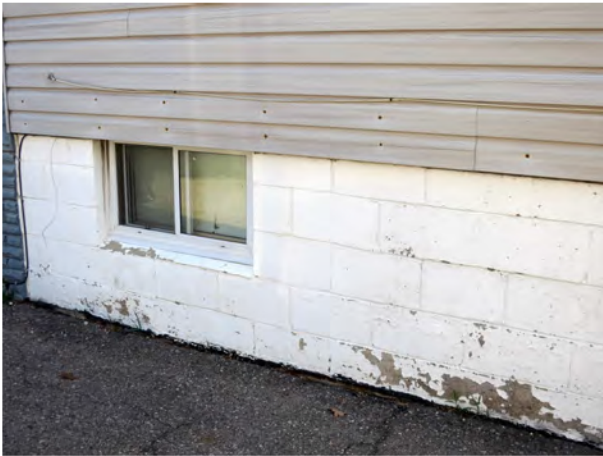
Figure 10: Raised concrete block foundation, vinyl siding and artificial stone facing.
