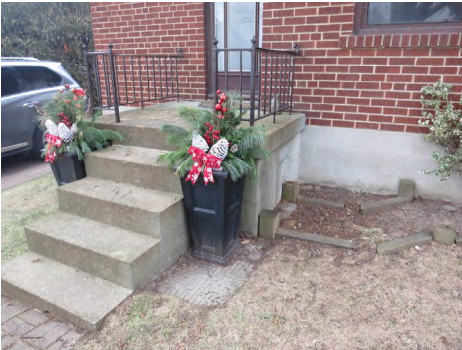
Figure 26: Main entrance, concrete stoop and concrete block foundation
