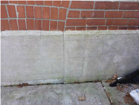
Cementitious parging rendered as unit masonry Parging delaminating in some locations
