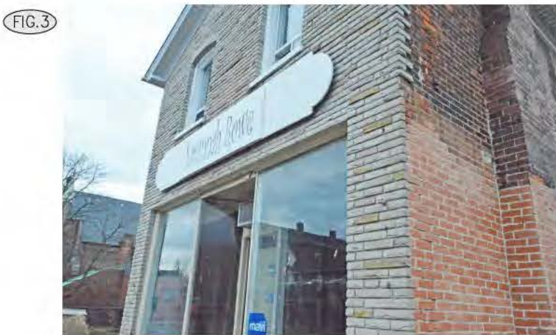
UNDERTAKE A TEST PANEL IN REMOVING "ANGEL STONE" FACADE FROM BUILDING FACADE TO INSPECT CONDITION OF BRICK BELOW. INTENT TO SALVAGE EXISTING BRICK AND REVERSE FACE USING BACK OF BRICK.
