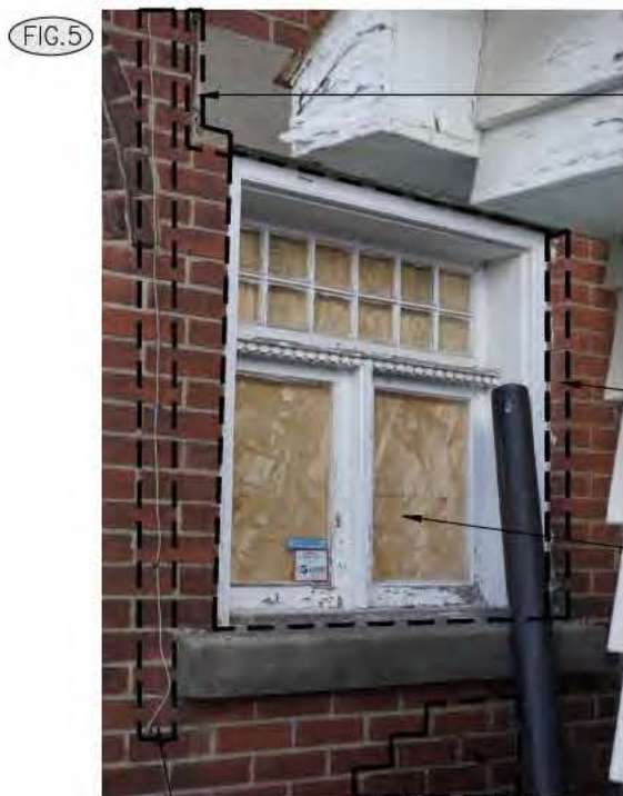
PANEL CLADDING SYSTEM TO BE USED OVER EXPOSED WOOD BOARDS.
