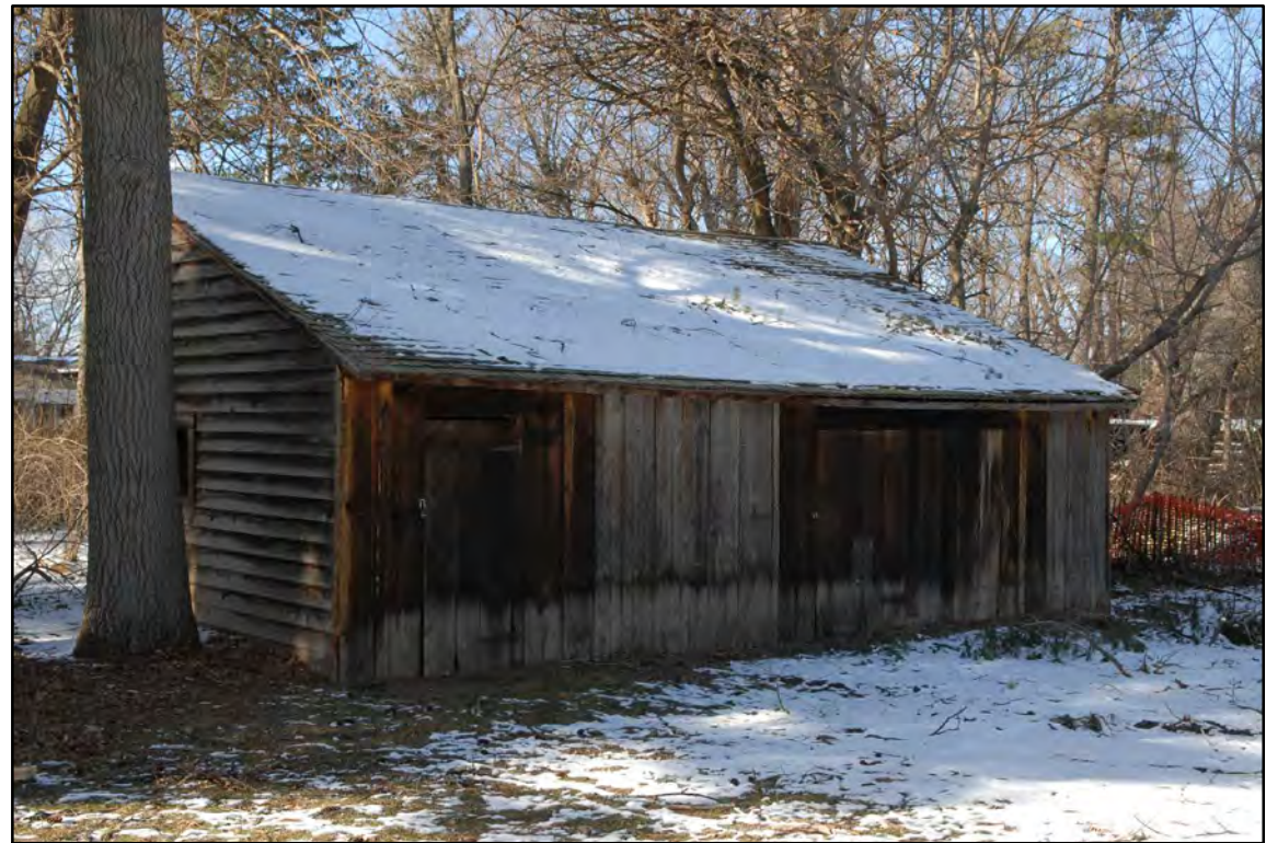
SOUTH-WEST OBLIQUE VIEW - NOTE DIS-SIMILAR SIDING, GENERAL DETERIORATION OF BUILDING
