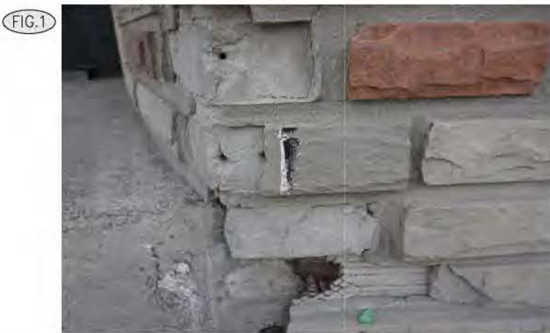
FIG.1 NORTH CORNER OF ENTRANCE STEPS TO THE STOREFRONT - SHOWING DETERIORATED ARCHITECTURAL STONE AND THE GROUND COAT OVER GALVANIZED METAL LATH BENEATH.
