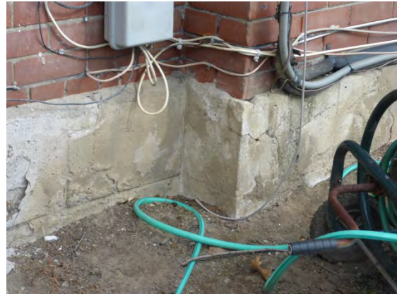
Cementitious parging rendered as unit masonry Parging delaminating in some locations
