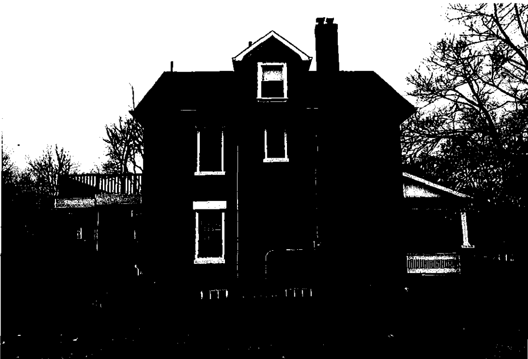
North Elevation showing original 1-storey brick element at rear, later wood-sided addition beyond
