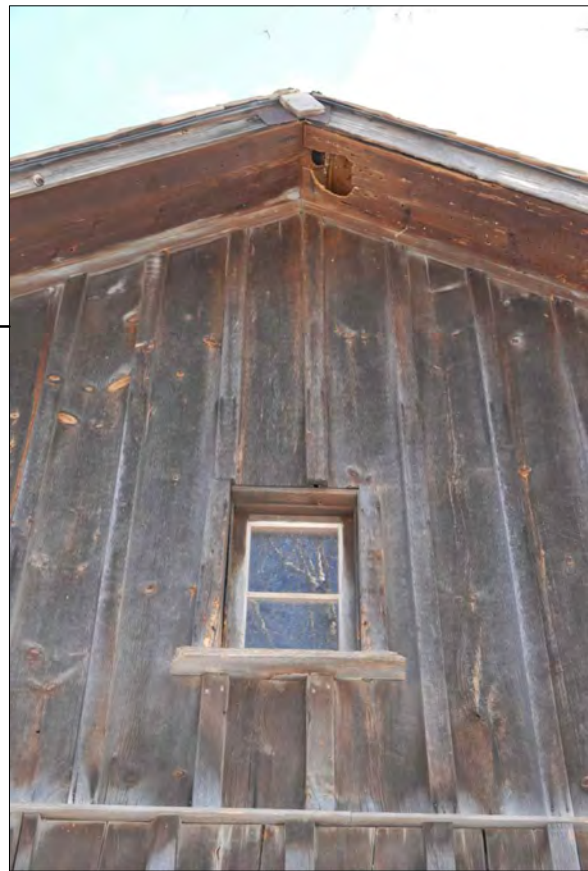
GABLE END – NOTE DETERIORATION AT WINDOW SILL AND TRIMS, DAMAGE FROM ANIMAL INFILTRATION AT SOFFIT, REPAIRED DAMAGED FROM ANIMAL INFILTRATION AT FASCIA
