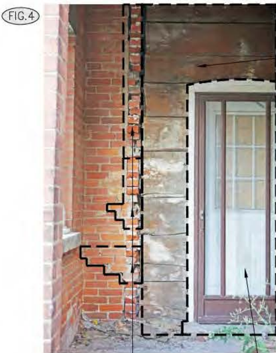
PANEL CLADDING SYSTEM TO BE USED OVER EXPOSED WOOD BOARDS.
