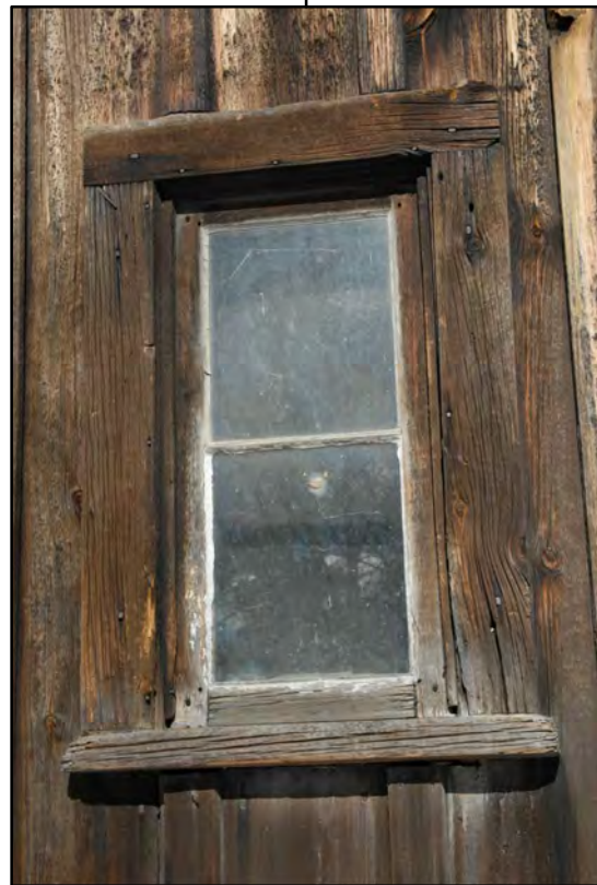
WINDOW — NOTE DETERIORATION AT LOWER SASH, SILL
