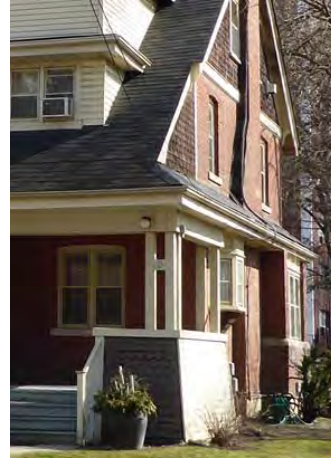
Vinyl Siding on side. All Wood members flashed in metal
