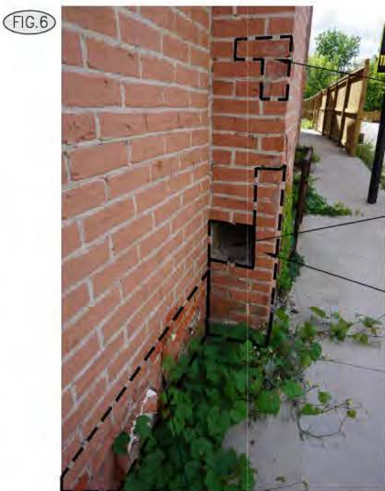
UNDERTAKE A TEST PANEL IN REMOVING "ANGEL STONE" FACADE FROM BUILDING FACADE TO INSPECT CONDITION OF BRICK BELOW. INTENT TO SALVAGE EXISTING BRICK AND REVERSE FACE USING BACK OF BRICK.
