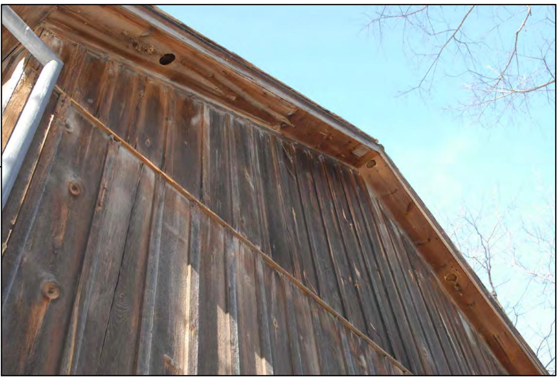
SOFFIT — NOTE HOLES GNAWED BY ANIMALS SEEKING ENTRY INTO BUILDING
