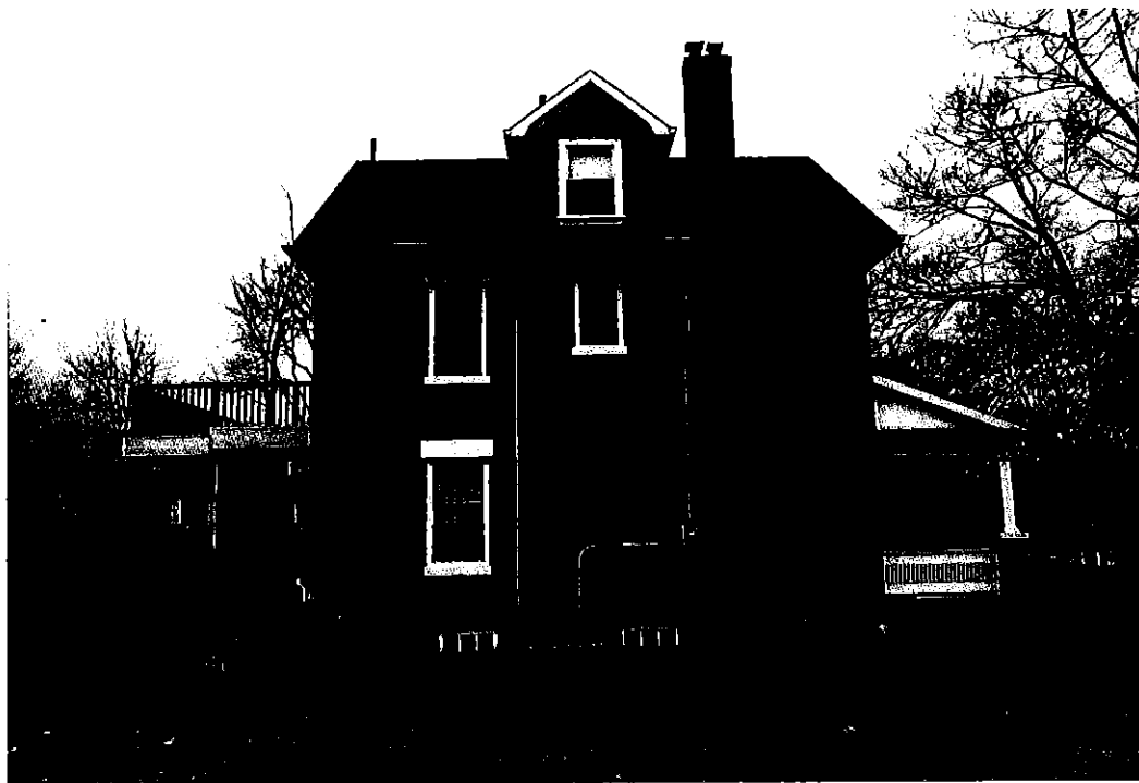
North Elevation showing original 1-storey brick element at rear, later wood-sided addition beyond
