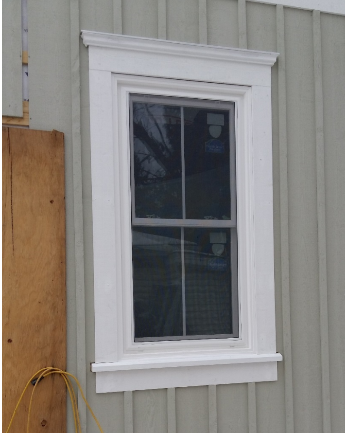
Figure 2: Close up of window on North West side - Double hung window with saddle bars dressed with wood trim & wood window sill
