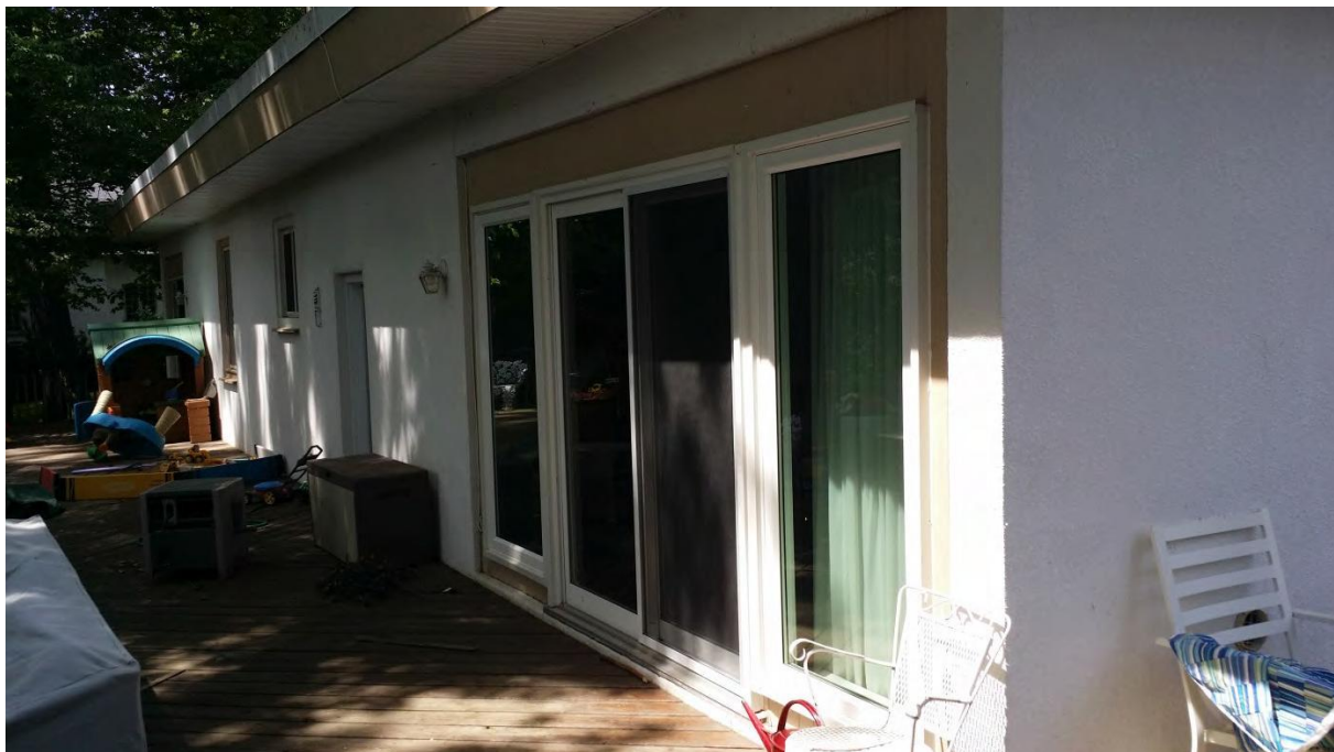
Back wall at deck (note punched opening detail at sliding door)
