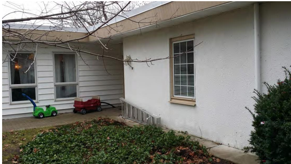
Original wall cladding and window detailing at right, later addition at left. Note downpipe at right
