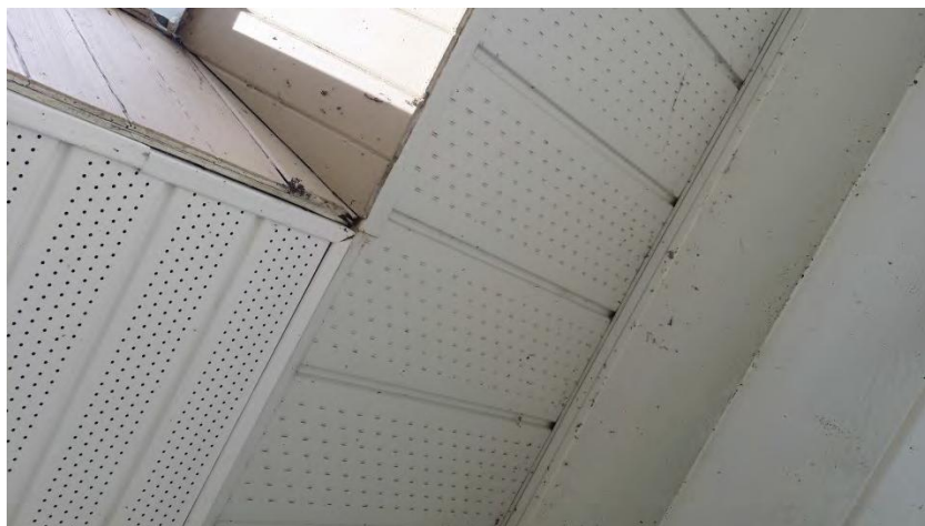
Soffit and fascia (note mis-matched newer materials, plywood covering fascia, poor detailing)
