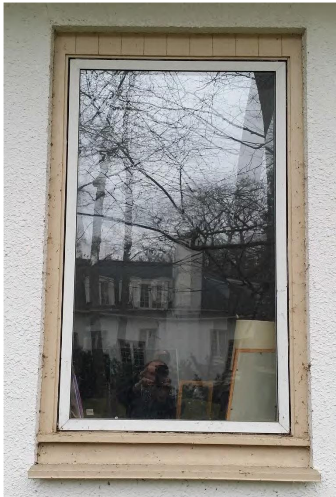
Original window detail (note oversized, punched opening, extruded metal sill)(note newer sash and glazing)
