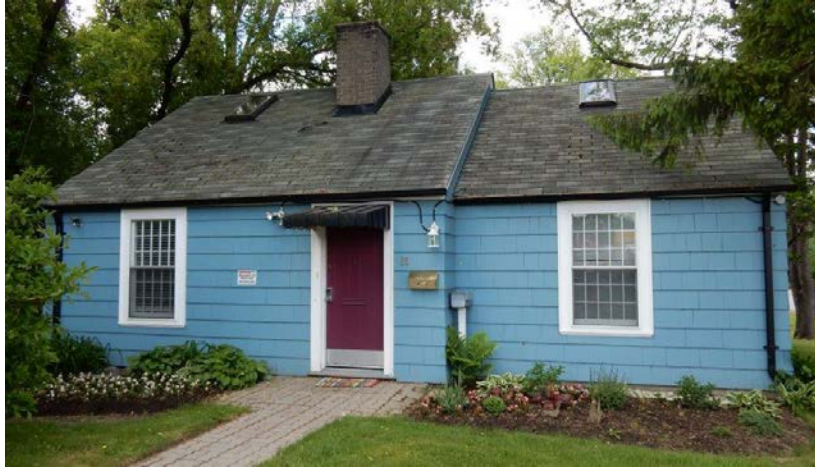
Contemporary additions, including skylights, metal awning and door hardware
