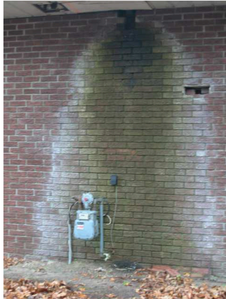
Significant staining of the brick from water runoff
