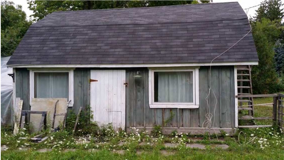
Barn south elevation. Note inappropriate newer windows, general lack of maintenance
