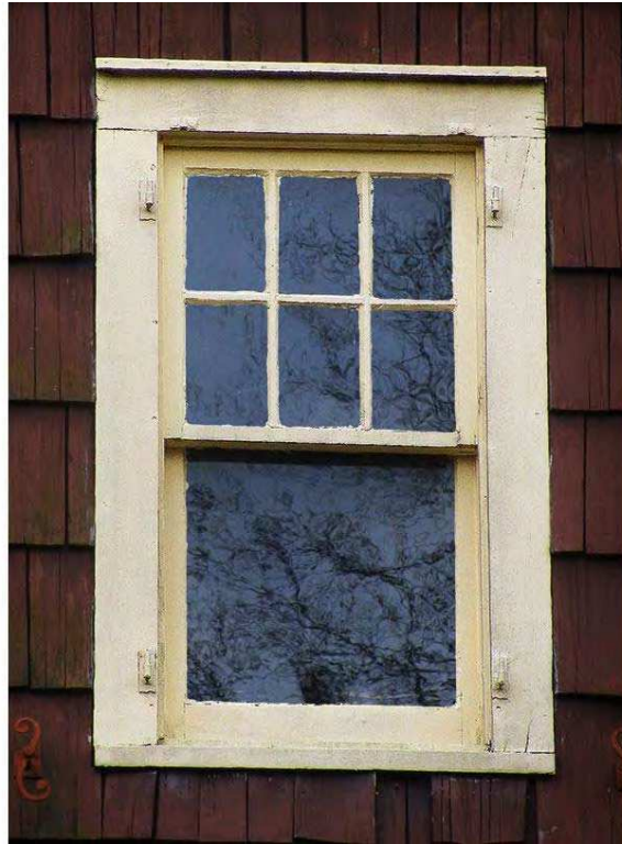
Typical 19th Century wood sash with simple flat casing, sill and head trim. Note lack of built up or composite elements and wood siding obviously fitted around window (example only - not from this project)
