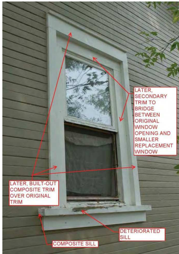
Detail of trims on south elevation showing composite trims, poor detailing and workmanship
