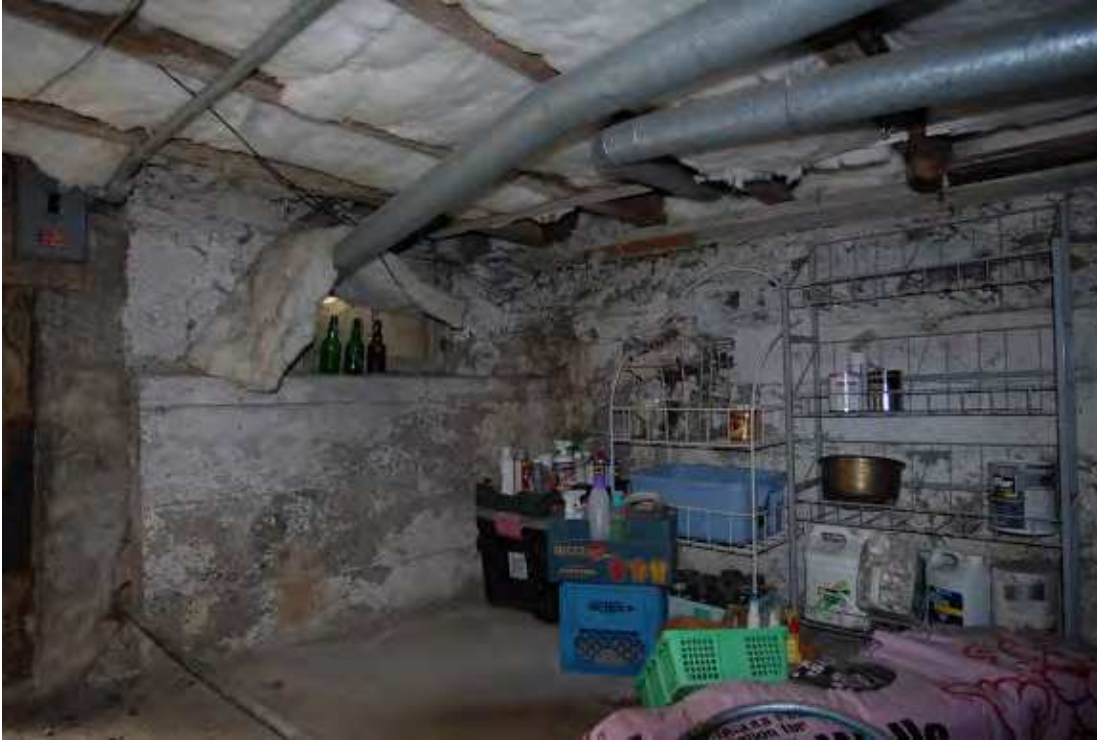
Existing Basement - note original stone wall at right, later underpinning at left
