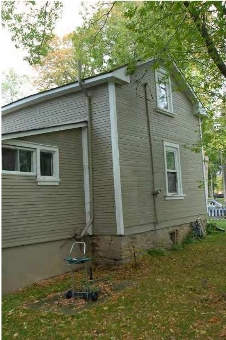
South-west oblique view showing rear addition. Note lack of foundation at addition.
