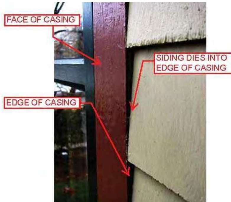
Typical 19th Century flat casing and siding detail showing correct minimal projection of casing beyond siding (example only - not from this project)
