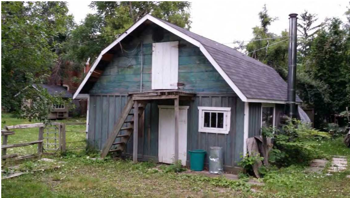
East and north barn elevations. Note metal chimney from wood stove within and stairs to second floor loft. These stairs and landing are in poor condition and missing handrails and guards. They are unsafe and should be removed
