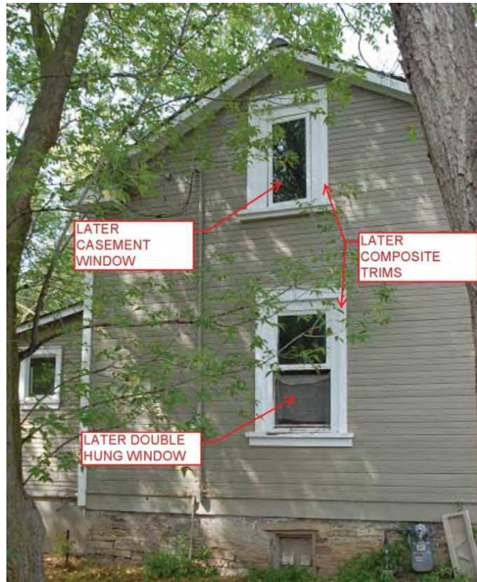
South elevation showing non-original windows and trims
