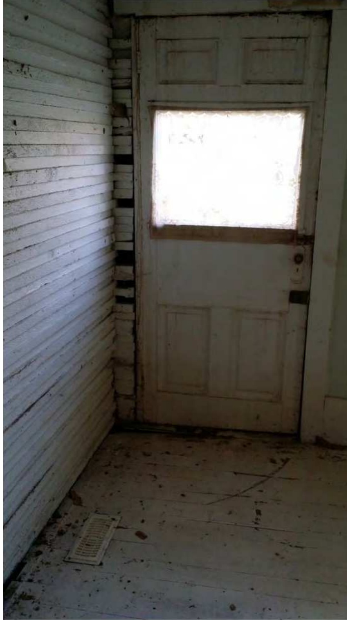
Front door from interior. Note general deterioration. Stacked plank construction can clearly be seen here
