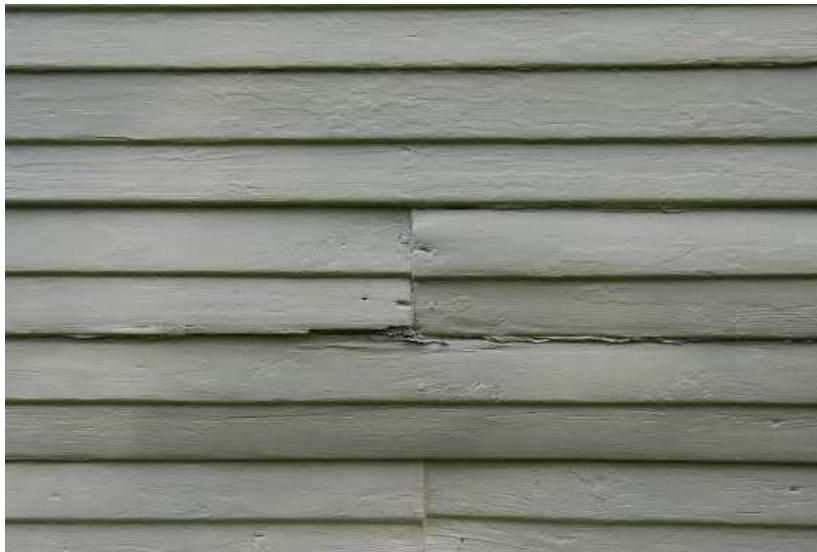
Weathered and deteriorated clapboard siding
