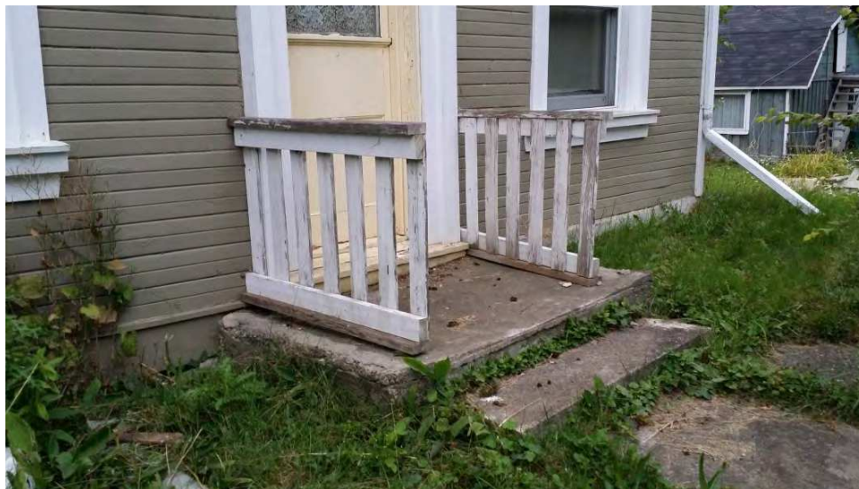
Present condition of encroaching front concrete landing and step
