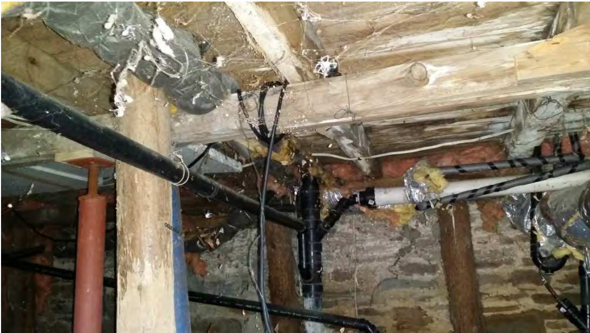
Rear addition under floor framing. House stone foundation is beyond. Note agglomeration of old and new posts, extensive deterioration, lack of insulation, haphazard construction
