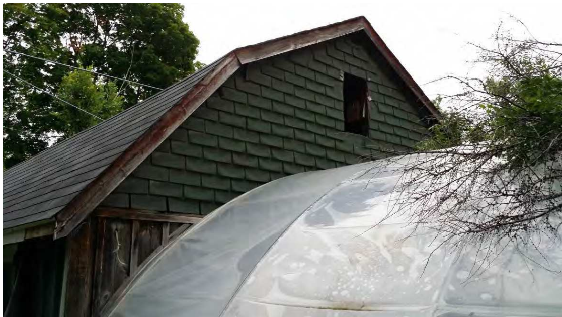
Barn west elevation. Later greenhouse structure in foreground. Note that trims and siding have not been painted here as they have on more visible east and south elevations
