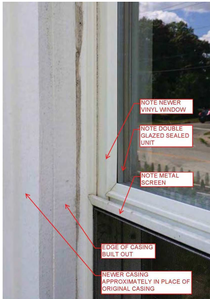
Detail of window on south elevation showing modern components, built out trims
