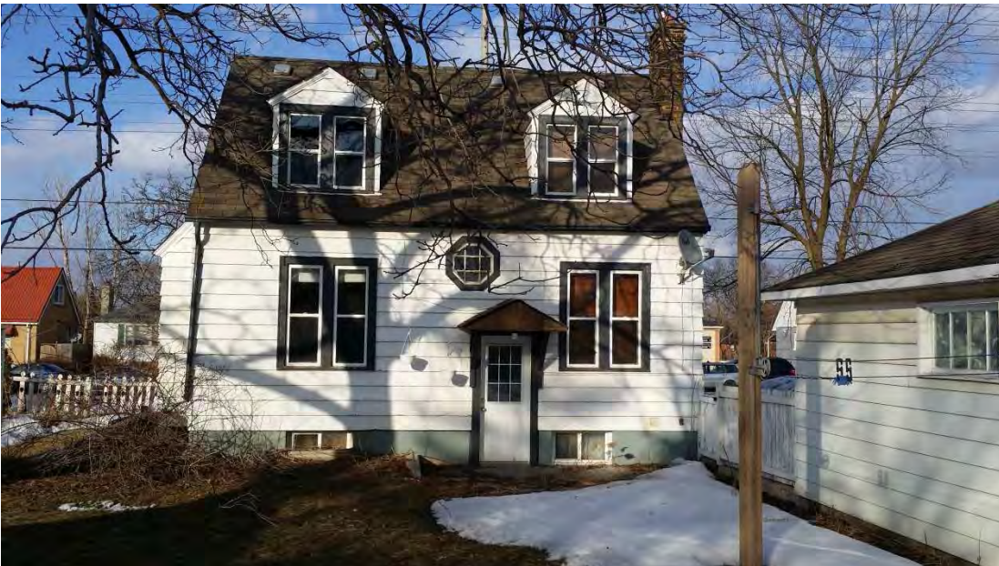
12 Queen Street South - rear elevation
