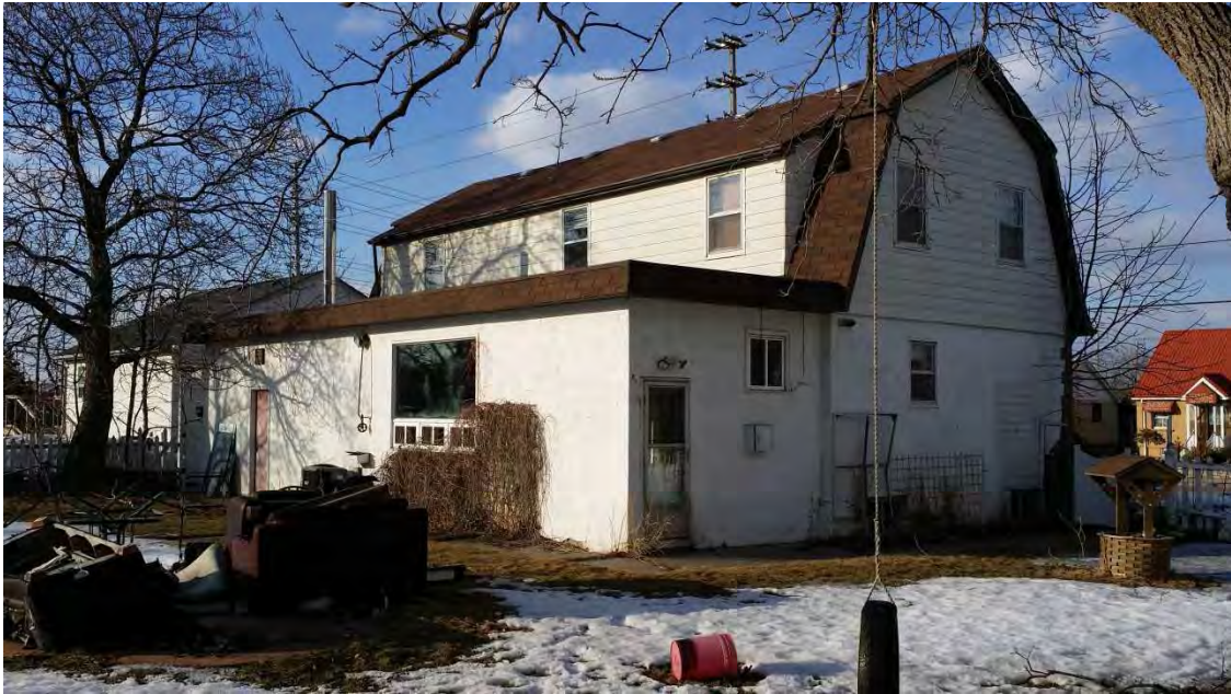
10 Queen Street South - south-west oblique view
