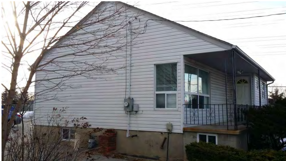
6 Queen Street South - south-east oblique view
