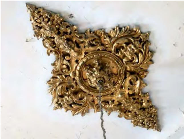
Figure 34: One of two gilded plaster medallions on the ground floor ceiling. This is similar to a medallion on the 2 nd floor and may be original.
