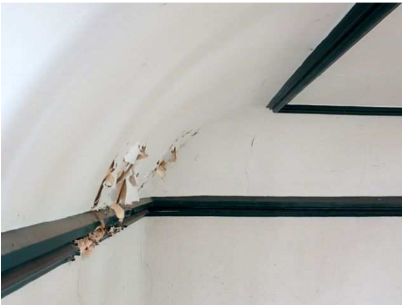
Figure 41: Detail of the plaster cove and plaster cornices.
