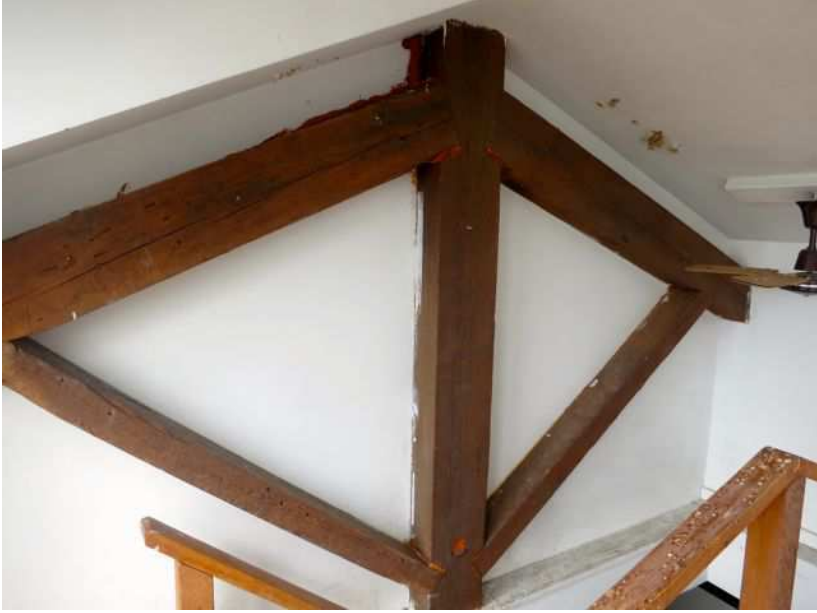
Figure 46: Detail of the original roof timbers in the loft.
