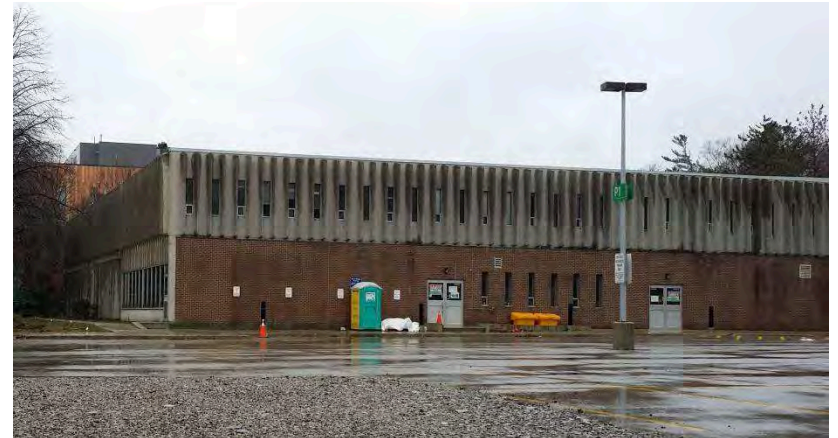
North Building awaiting demolition. Deerfield Hall in background.
