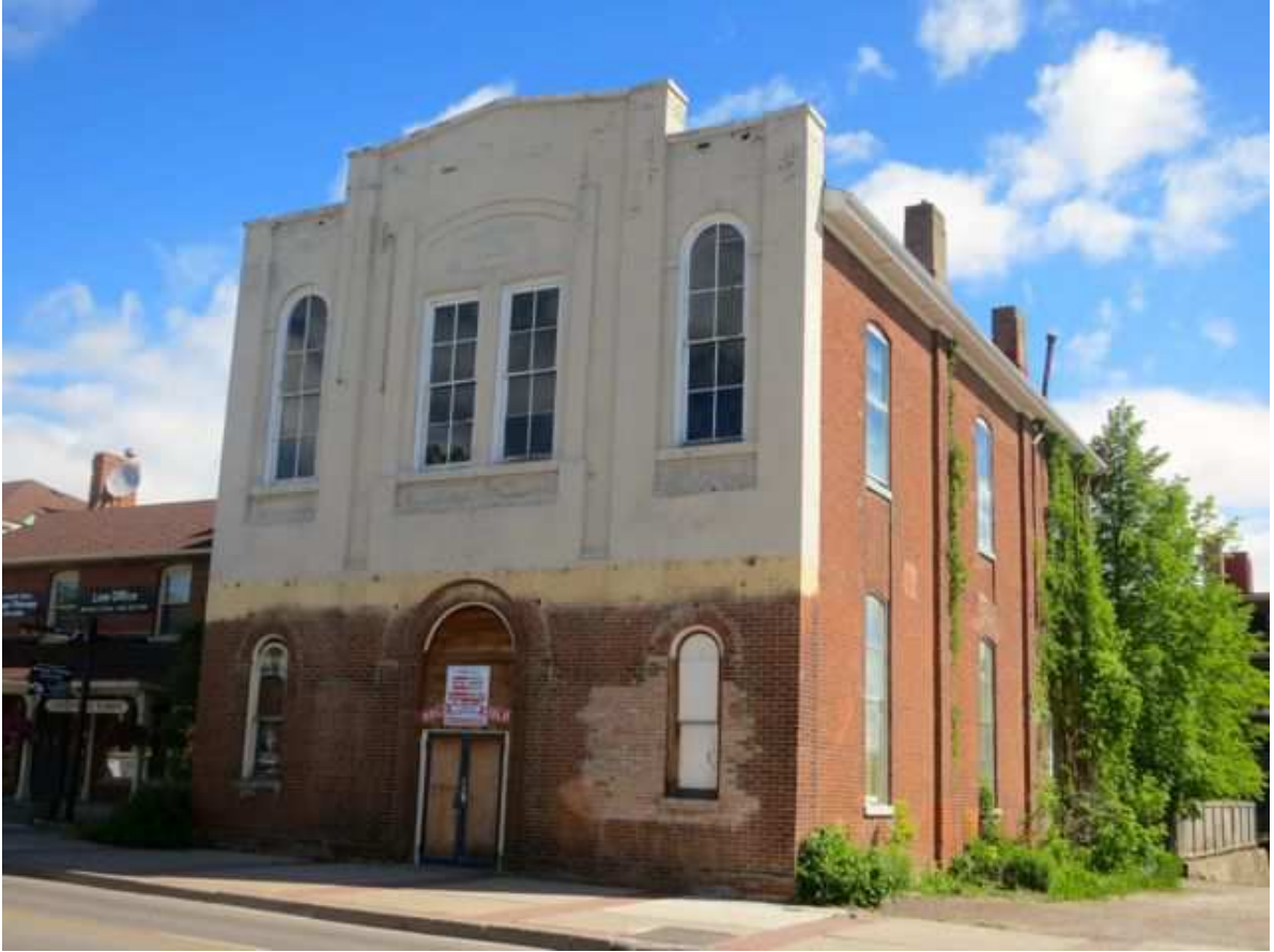
Figure 12: 471 Queen Street South, current condition. A previous owner removed the modern cladding from the ground floor and re-instated the arched windows. This work was poorly done and is not sympathetic to the original in materials or workmanship. The paint on the upper floor has not been removed. [M. Hobson June 2014]
