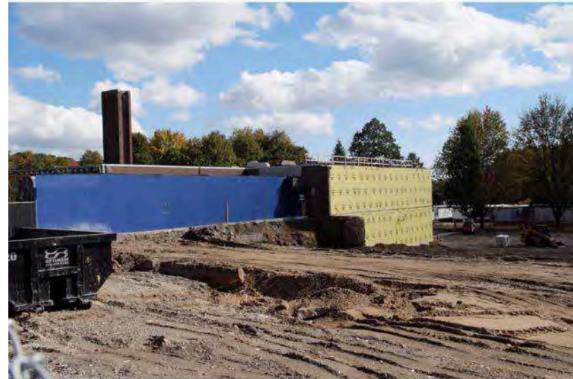
WEST ELEVATION (SHOWING RECENT PARTIAL DEMOLITION)
