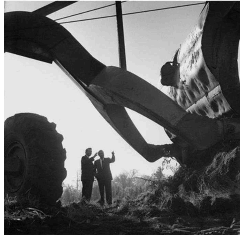
BILL DAVIS (LEFT) AT CONSTRUCTION OF NORTH BUILDING
