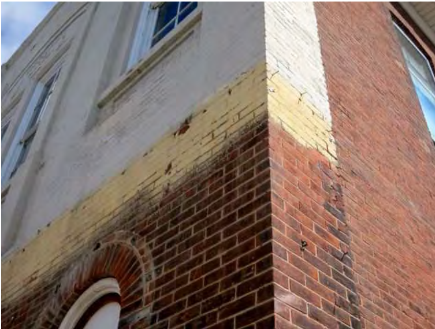
Figure 30; Detail showing painted and un-painted areas on the front facade.
