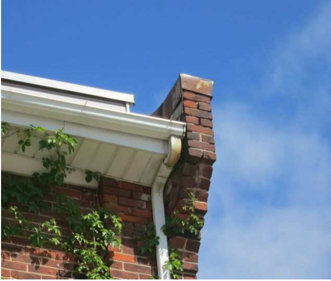
Figure 24: Brick corbels at the corners of the roof.
