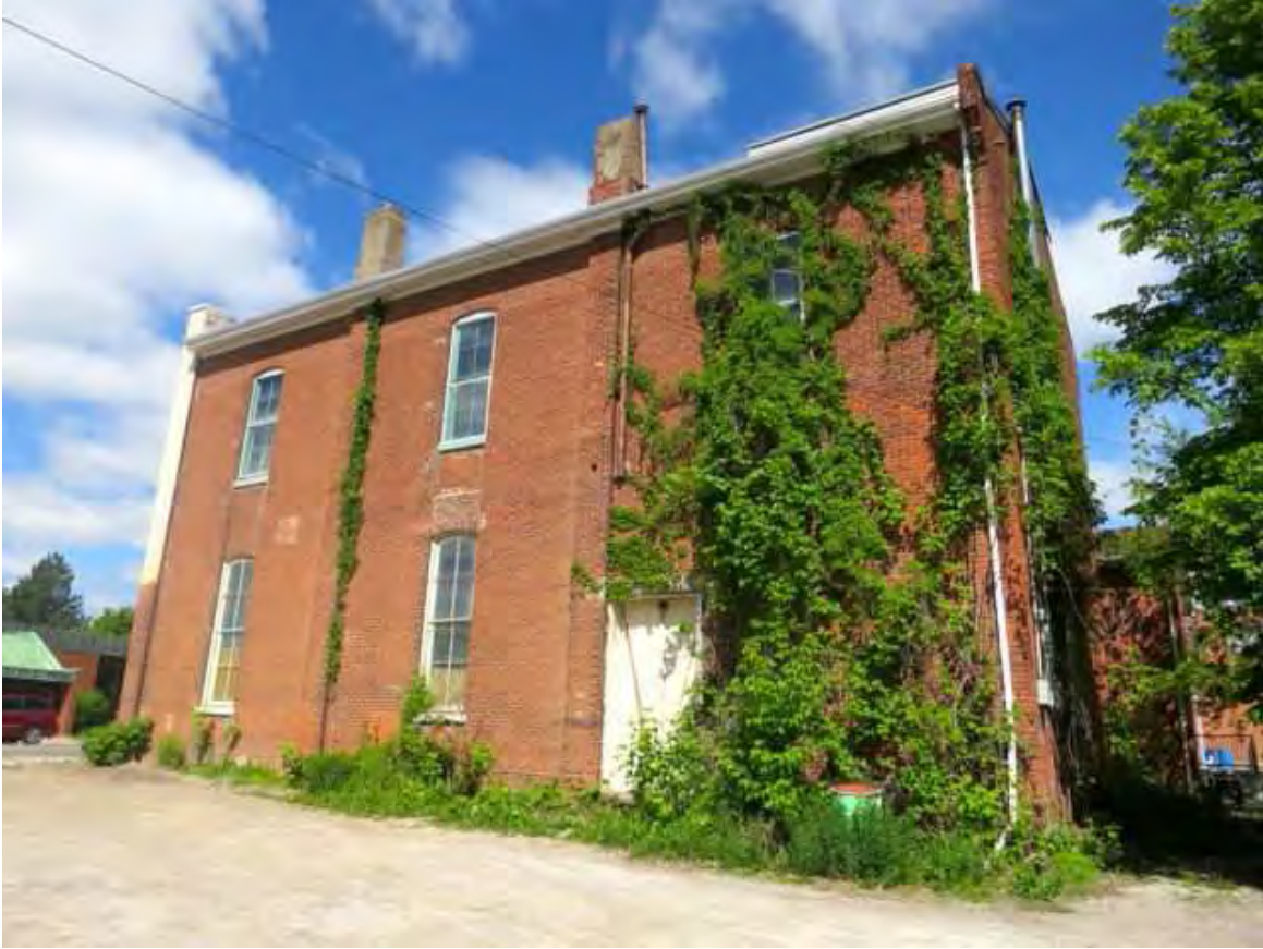
Figure 15: Side elevation adjacent to an empty lot. A door has been added at the rear for a loading dock. The chimneys have been parged with a cementitious material.
