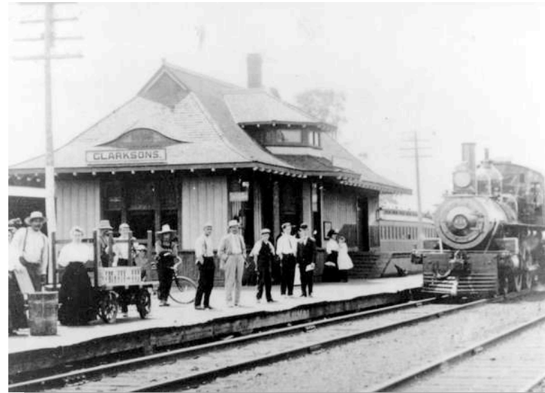
Above: Railway station at Clarkson
