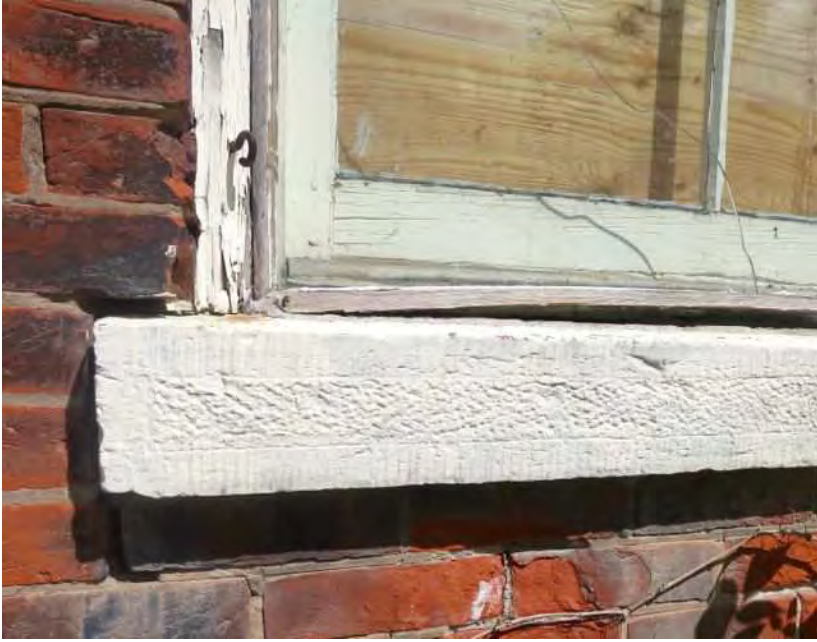
Figure 18: Cut and hammered stone window sill.
