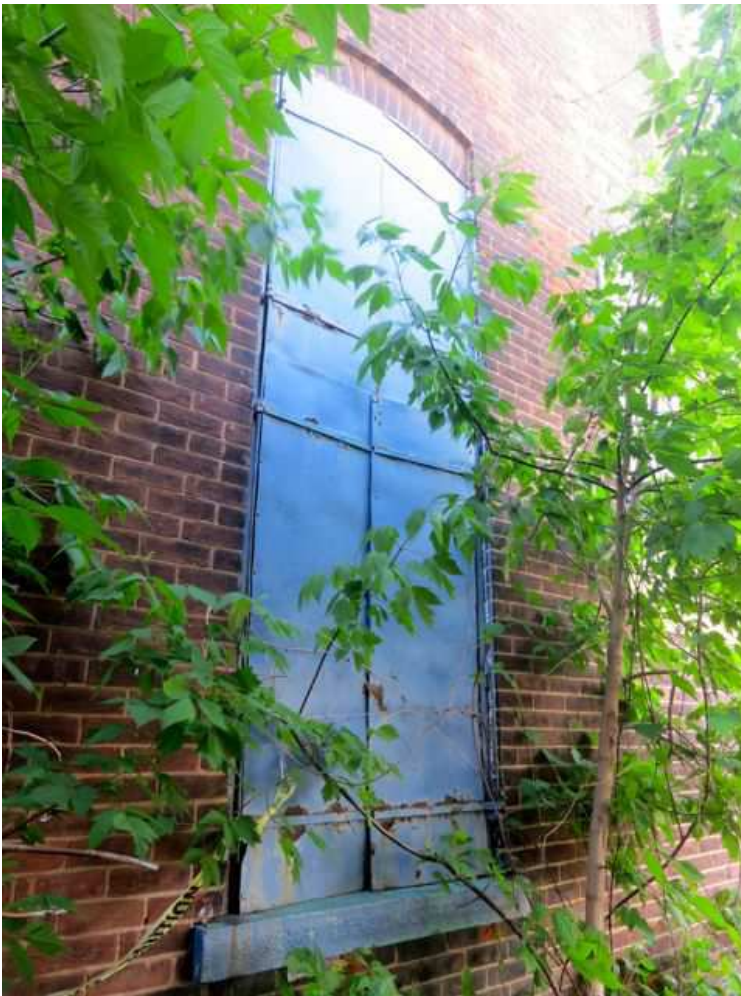
Figure 25: Metal doors or shutters on a window on the side elevation.
