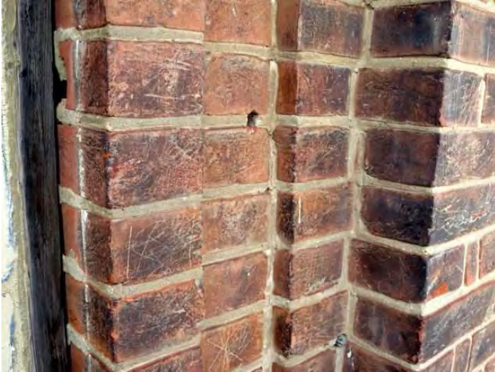
Figure 22: Detail of the brick arch around the front entrance.
