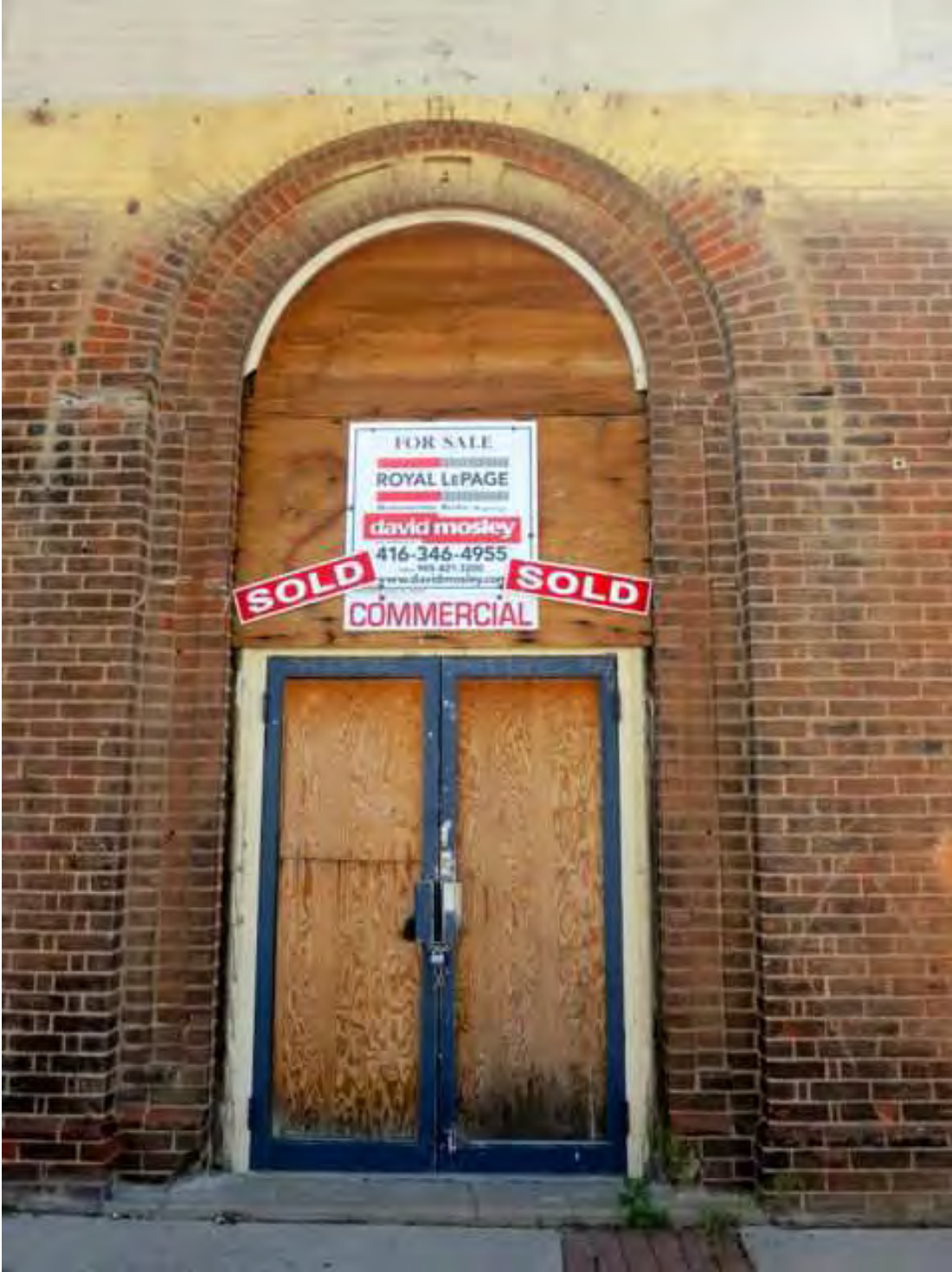
Figure 21: The original wood panelled door and arched transom have been removed and replaced by modern metal and plate glass doors. The recessed brick arch remains but the stone molding above has been removed.
