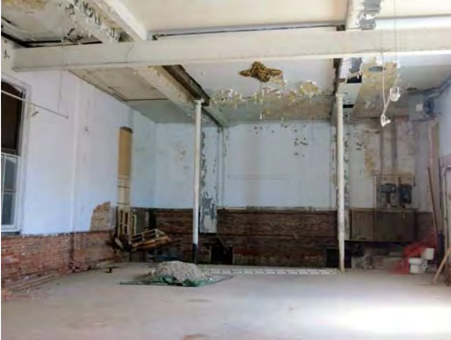
Figure 31: The ground floor interior is one large open space. Two cast iron columns support wooden timbers that extend from the front to the back. The walls have lime plaster with the exception of the area below the window sills which is bare and may have had wood panelling.
