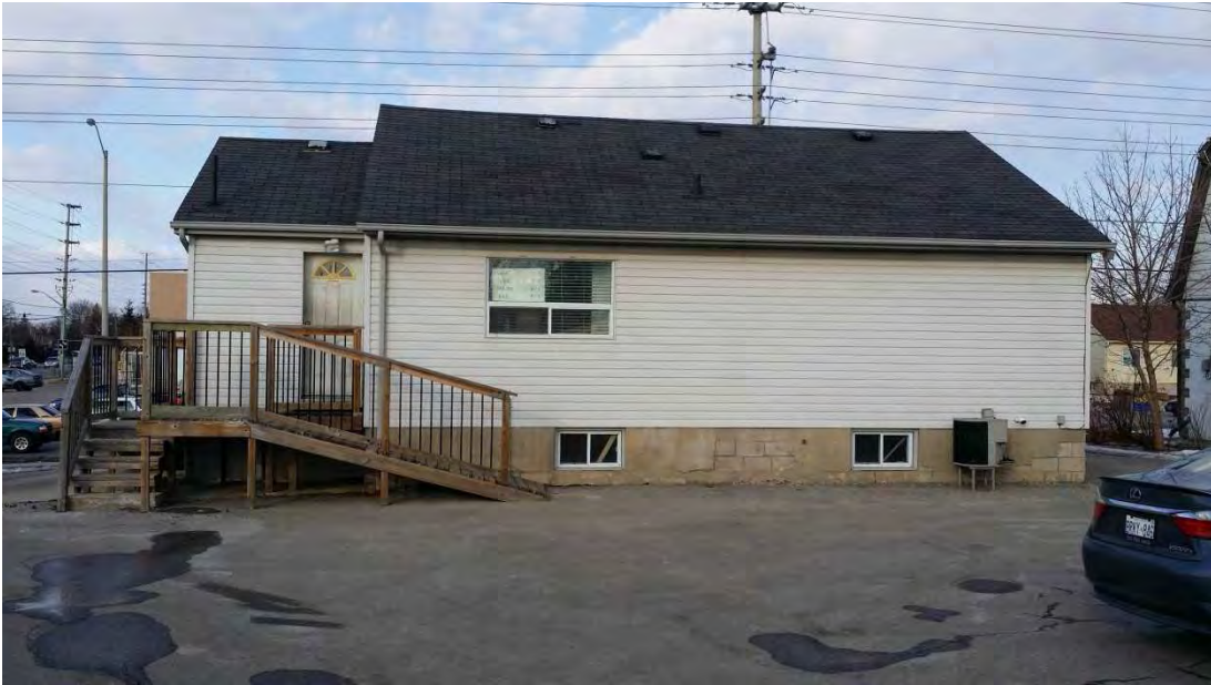
6 Queen Street South - rear elevation
