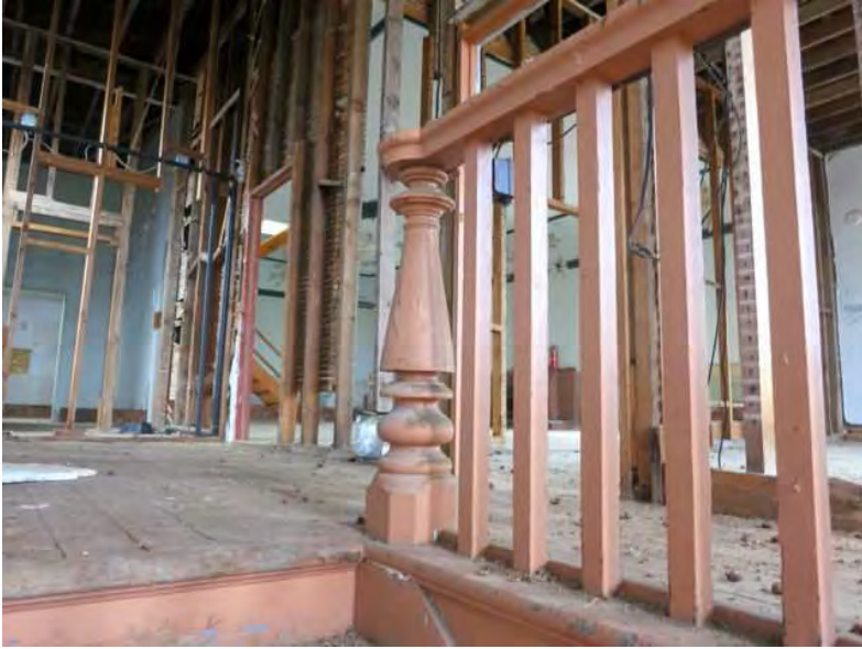
Figure 37: Newell post at the top of the stairs.
