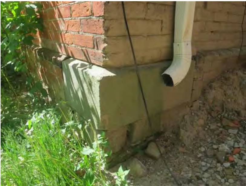
Figure 17: Cut and tooled limestone corner block.
