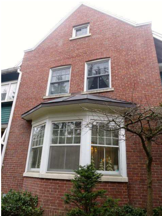
Figure 26: Dutch gable and bay window on the north elevation.
