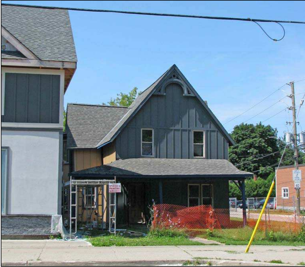
Front (east) elevation of the William Clarkson House [July 2015].
