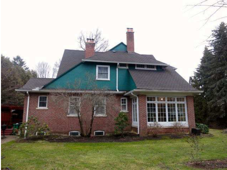
Figure 25: East elevation of the house fronting on Ben Machree Drive.
