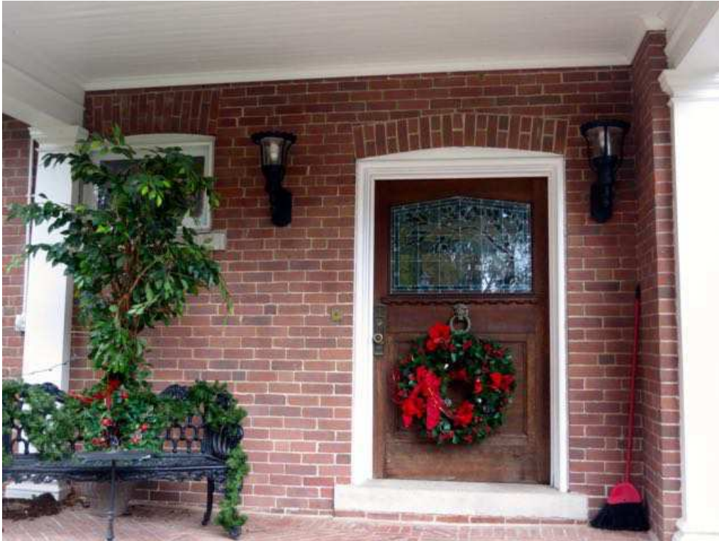
Figure 29: Front entrance on the North elevation.
