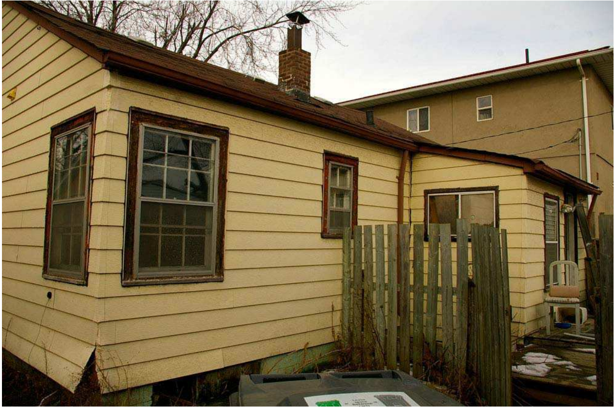
Photo 19: Rear façade looking north, showing two original corner windows in the rear bedroom, the original bathroom window (blocked up from inside) and a horizontal sliding window (covered on the inside). Also shows section of siding lifted to determine the original cladding material: asbestos-cement shingles, as illustrated in detail below.
