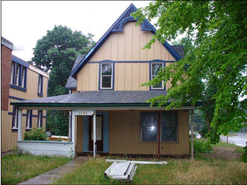
William Clarkson House, front (east) elevation [Heritage Mississauga, 2005].
