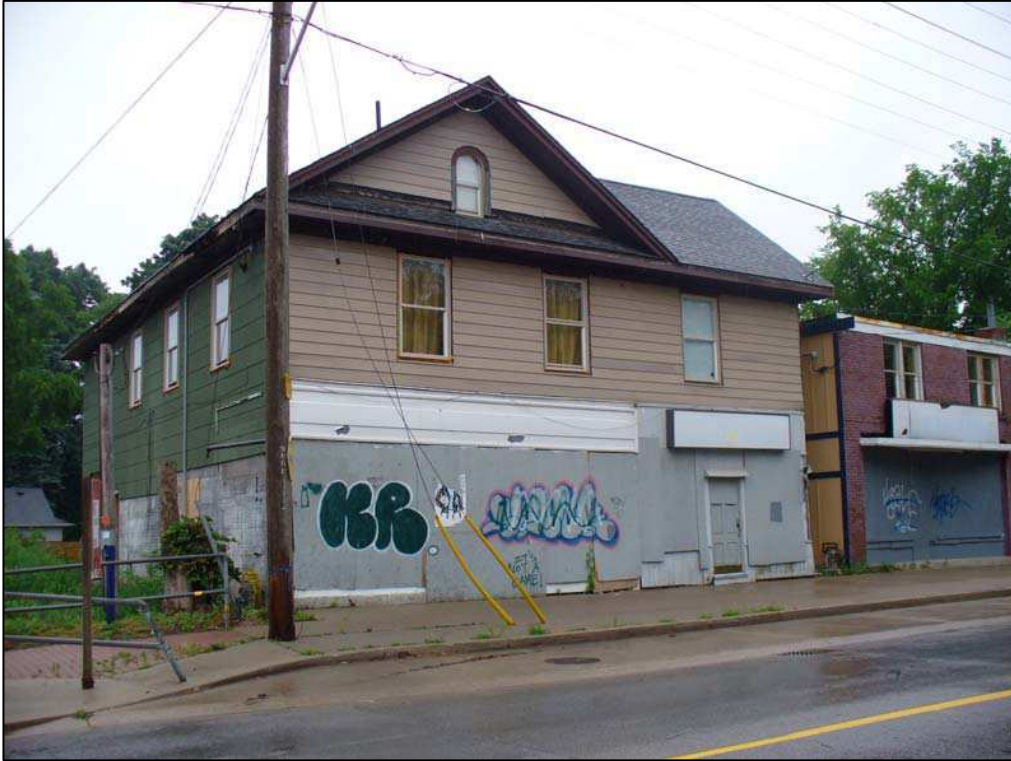
Clarkson Store, front (east) elevation [Heritage Mississauga, 2005].
