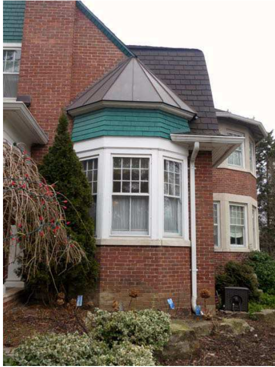
Figure 27: Tower on the north elevation.
