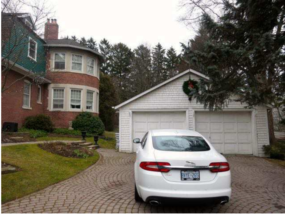
Figure 3: Existing 2-car detached frame garage constructed c. 1970.
