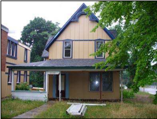
Figure 28. The front (east) elevation of the William Clarkson House [Heritage Mississauga, 2005].
