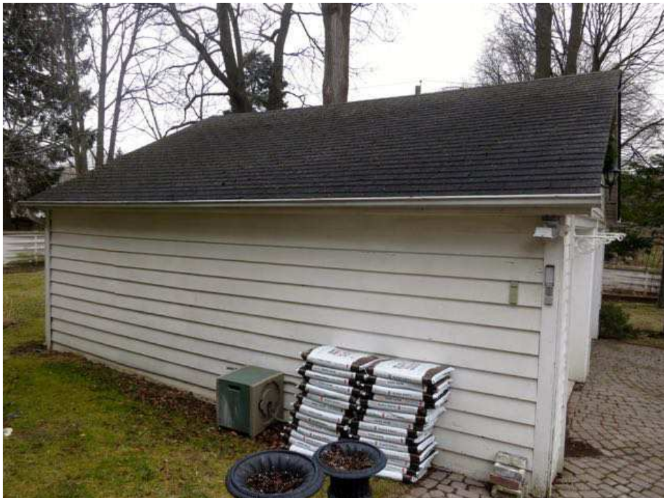
Figure 4: Side view of existing garage.
