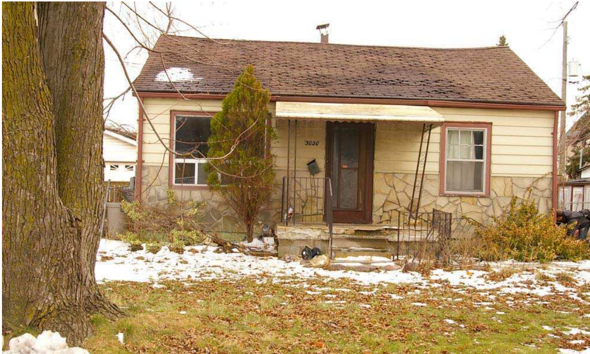
Photo 17: Front façade shows the aluminum siding with a flagstone-like synthetic cladding material added to the lower half of the wall.
