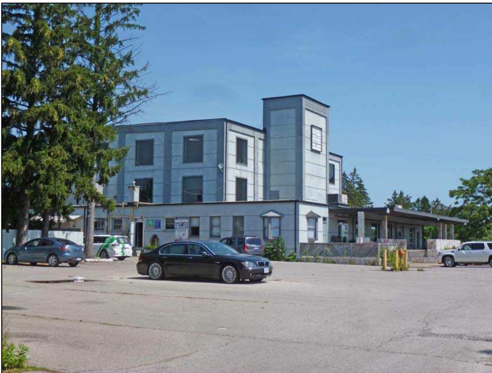
Former Clarkson Basket Factory buildings behind 1119 Clarkson Road North.
