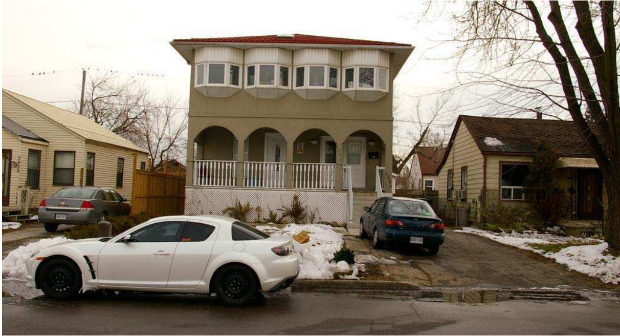
Photo 5: This two-storey dwelling at #3024 is definitely an original wartime bungalow, enlarged by the addition of a projecting second storey in 2000, when the entire exterior was stuccoed. (CM Property Information) The oriel-like second storey windows projecting over the colonnaded verandah border on the bizarre.
