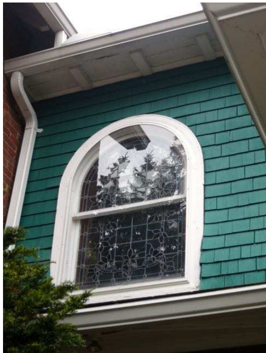
Figure 28: Round arched window and wood shingle on the north elevation.
