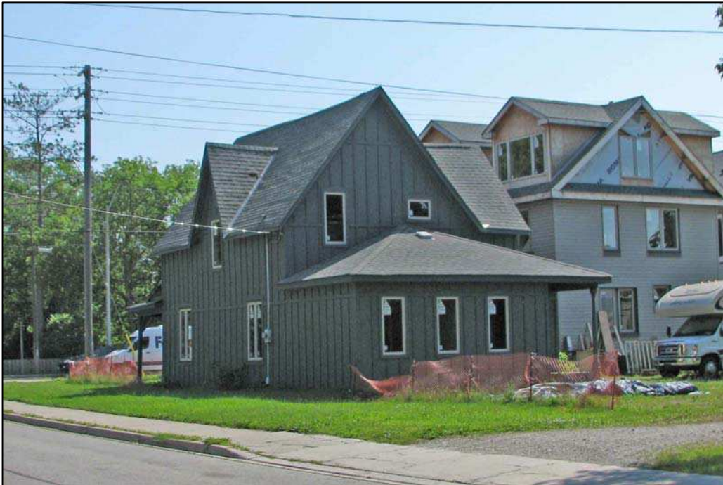
Rear (east) elevations of the William Clarkson House [July 2015].
