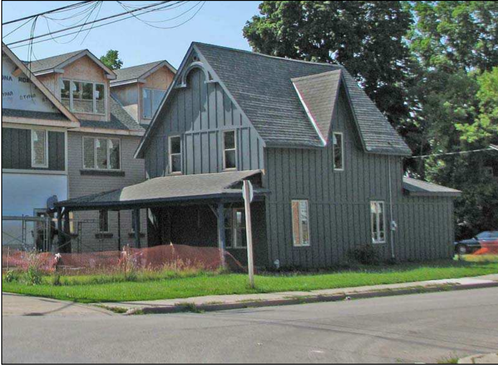
North and east elevations of the William Clarkson House [July 2015].
