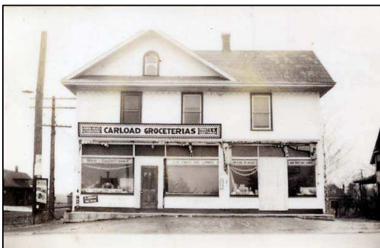
Figure 22. The front elevation of the Carload Groceterias [Clarkson Store] on Clarkson Road North [MLS, Historic Gallery, BA0074, undated].
