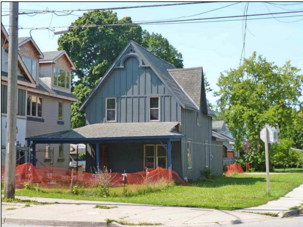
Front (east) elevation of the William Clarkson House [July 2015].
