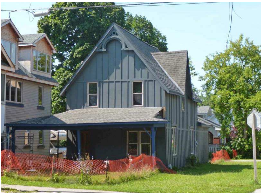
Figure 25. The front (east) elevation of the William Clarkson House [July 2015].
