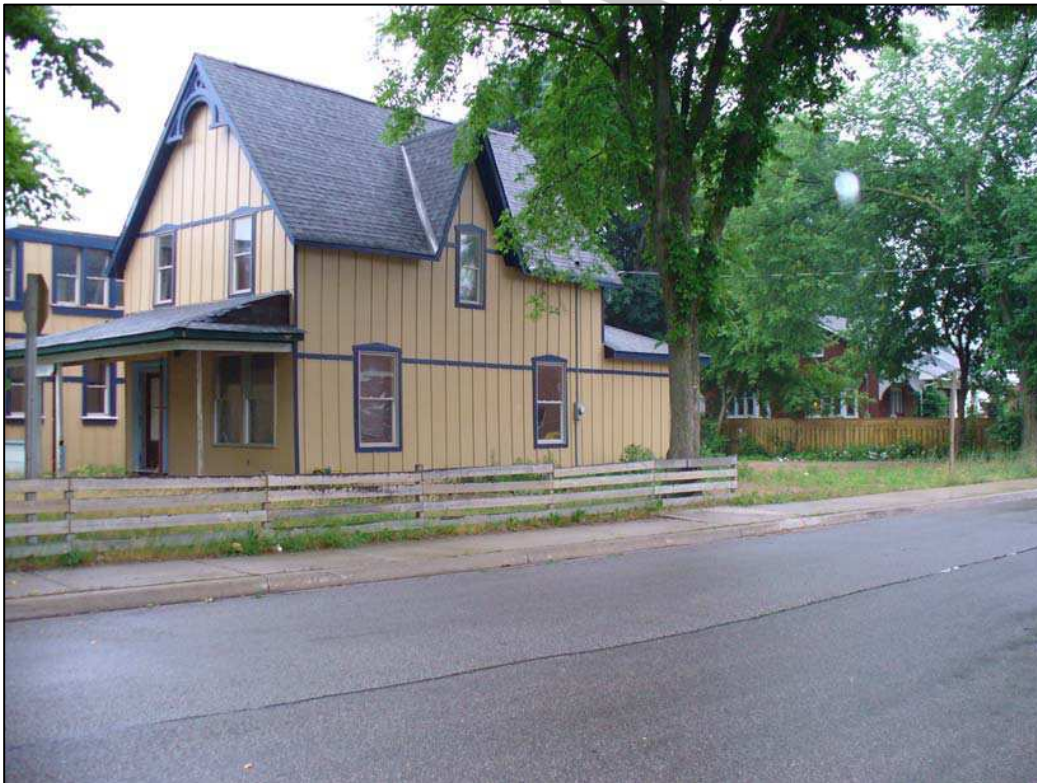
William Clarkson House, northeast corner [Heritage Mississauga, 2005].
