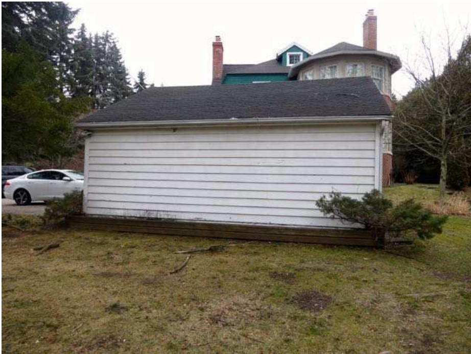
Figure 6: Side view of existing garage.
