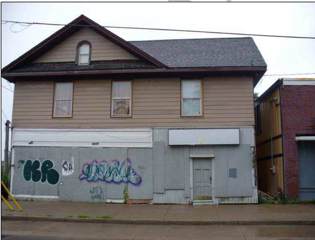
Clarkson Store, front (east) elevation [Heritage Mississauga, 2005].
