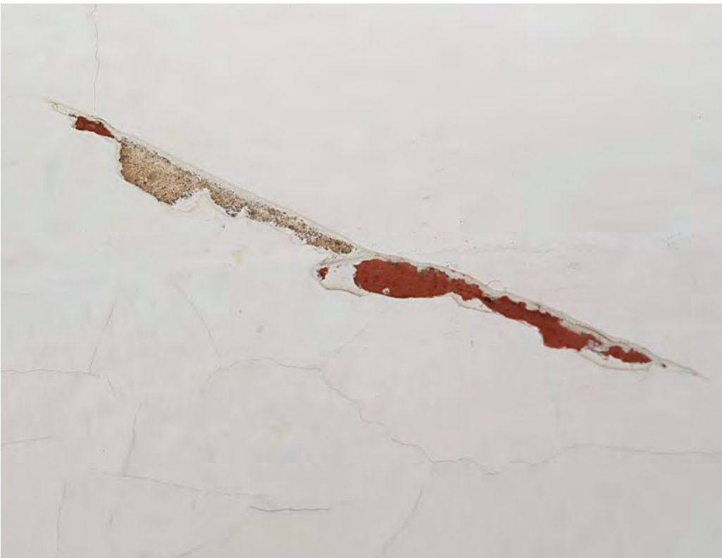
Figure 16: Paint loss showing possible yellow brick at second storey enclosed patio [July 2016]
