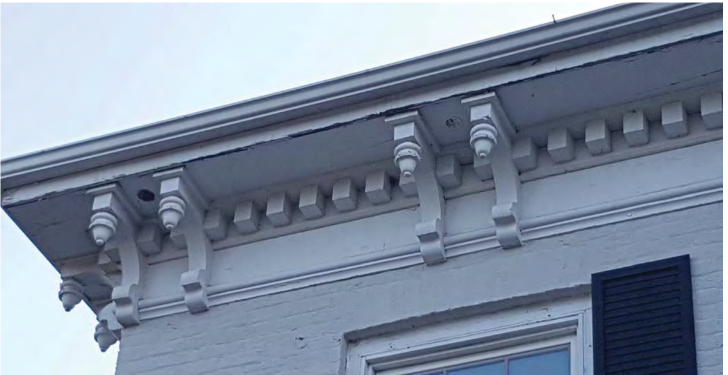
Eaves detail, with brackets, dentils and fascia [July 2016]
