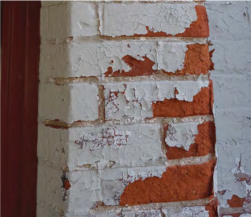
Figure 15: Paint loss showing brick colour at front entrance [July 2016]
