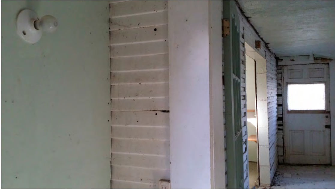
Interior view from vestibule toward front door. Note newer drywall on north wall of vestibule, older siding material on west wall of vestibule, stacked plank construction visible in living room beyond
