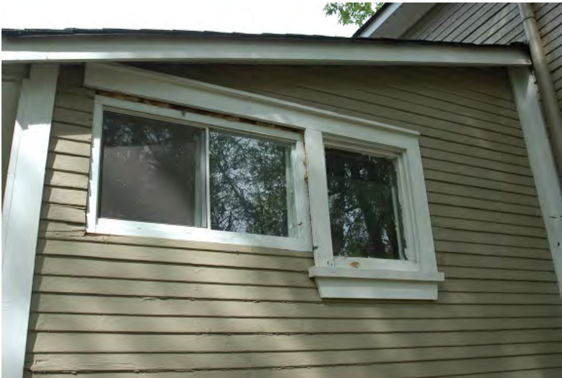
South elevation of rear addition showing newer windows, haphazard, poorly detailed trims, deteriorated siding.
