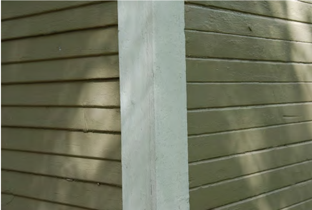
Corner detail showing differential siding materials. Material at left is horizontal clapboard with 4" exposure. Material at right is 8" shiplap with center dado detail to make it appear as 4" widths. Corner boards are all later replacements.
