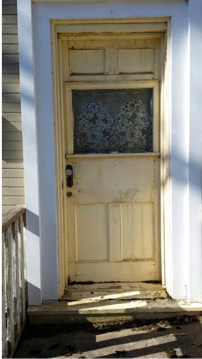
Front door from exterior. Note deterioration at bottom of door and sill. Note inappropriate opening cut for window and associated trimwork
