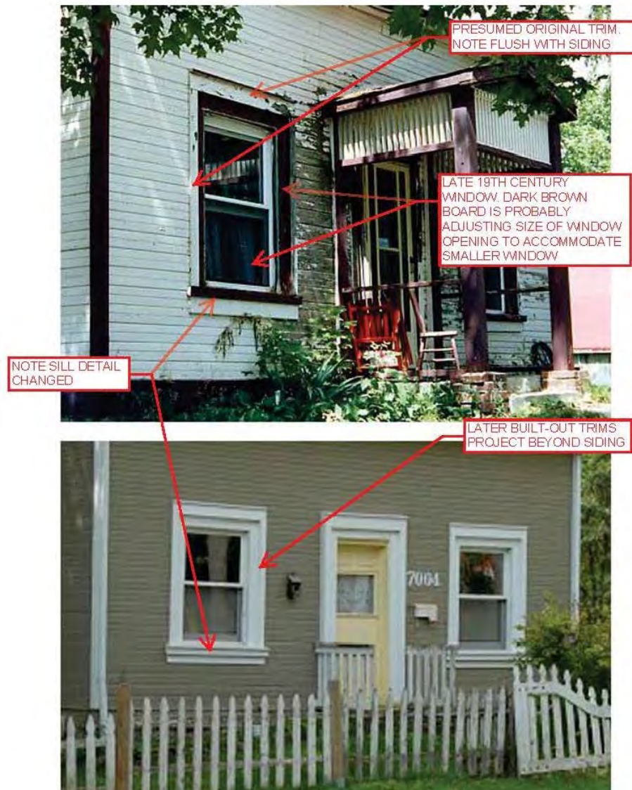
Front elevation comparing images from 1980's and present day showing non-original windows and trims
