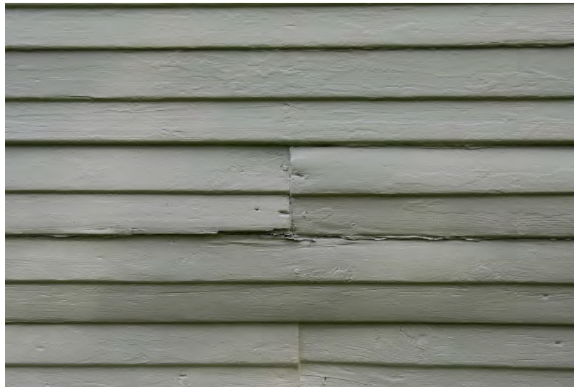
Weathered and deteriorated clapboard siding
