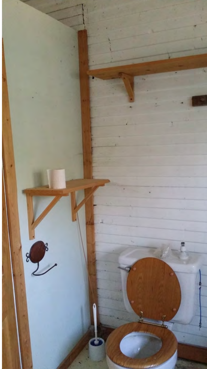
Bathroom interior showing older siding material as wall finish. Note patched siding material at upper left
