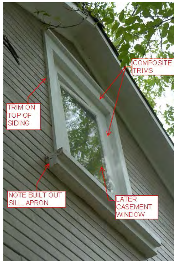
Detail of window on south elevation showing built out trims, poor detailing and workmanship
