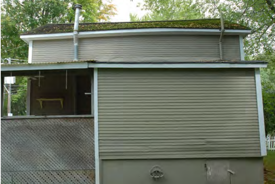
West elevation of rear addition and later covered porch. Note deformation of upper roof/rear wall on main building.
