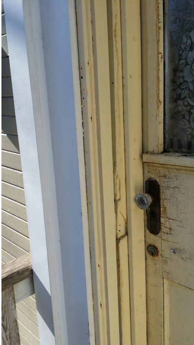
Detail at front door jamb. Note layers of built-up trimwork, deterioration of door
