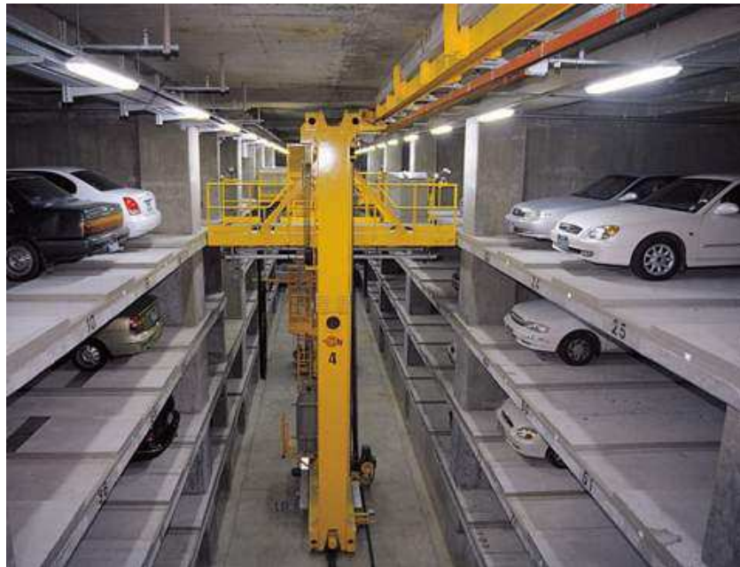
Figure 4 - 1 Parking Stacker, an example of a space-saving 'Terminal Facility'
