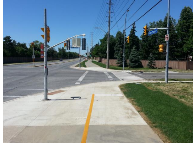
Figure 8: Adding a crossride with a smooth curb cut, trail markings with a stop bar, and bicycle signals makes the path clear for cyclists, and shows motorists where to expect cyclists. Reducing the curb radius of the turns would also significantly increase safety. Pedestrians have a crosswalk, which leads to less conflict between trail users, at a point where all have to concentrate on making a safe crossing.
