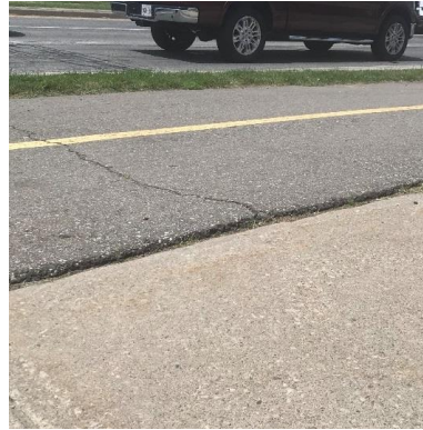
Figure 11: Differential Settling of Concrete and Asphalt
