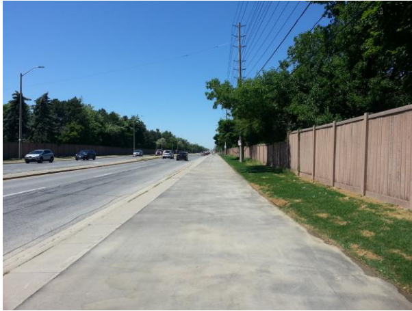
Figure 3: Looking north from Oka Road, on the east side of Winston Churchill Boulevard. The asphalt trail is 3.75 m wide, with a standard 0.75 m concrete splash pad as a buffer.
