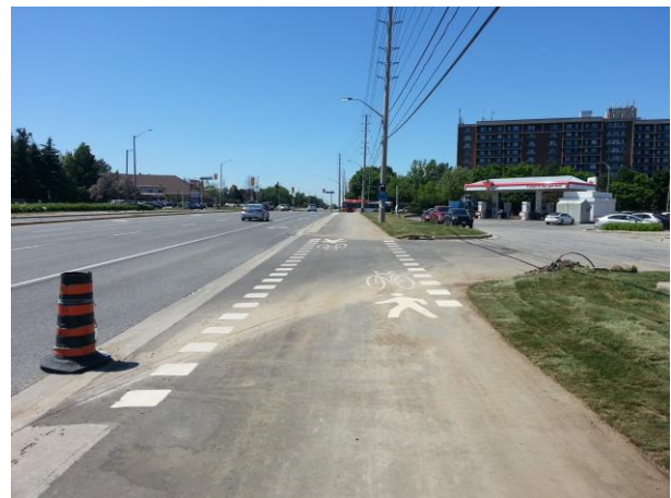
Figure 10: A mixed crossride (cyclists and pedestrians share the space) shows a clear path of travel, and indicates to both trail users and motorists that this is a conflict point.
