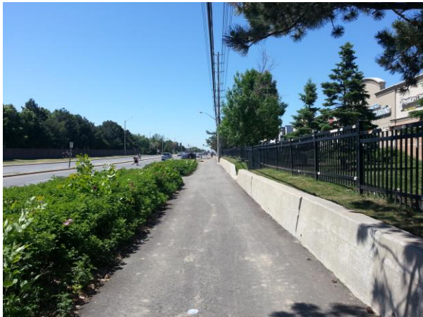
Figure 5: A narrower section of trail between Meadowvale Town Centre Circle and Battleford Road. The trail is 3.0 m wide, but well buffered from the roadway by shrubs and grass. However heavier pedestrian use in this area can cause conflicts between users.
