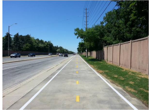
Figure 4: Conceptual graphic of edge and centre lines applied to the trail. The road buffer can be increased by moving the edge line. In this case, moving the line 0.25 m inwards results in a 1.0 m buffer, and 3.5 m wide trail.
