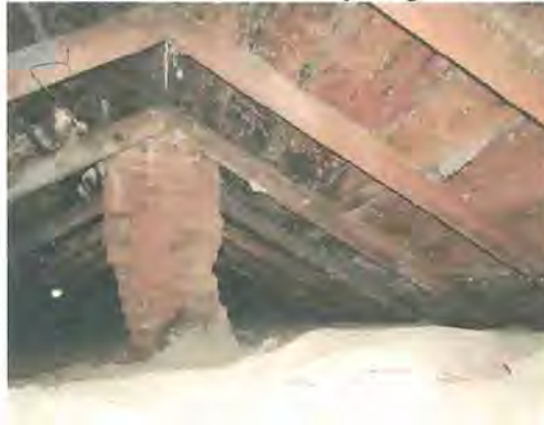
Absence of dormer framing in attic
