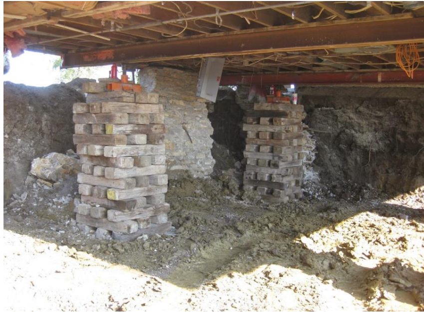
BUILDING SUPPORTED BY BEAMS, JACKS AND CRIBS
