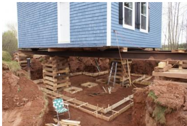
FORMWORK FOR NEW FOOTINGS/FOUNDATION UNDER TEMPORARILY SUPPORTED HOUSE
