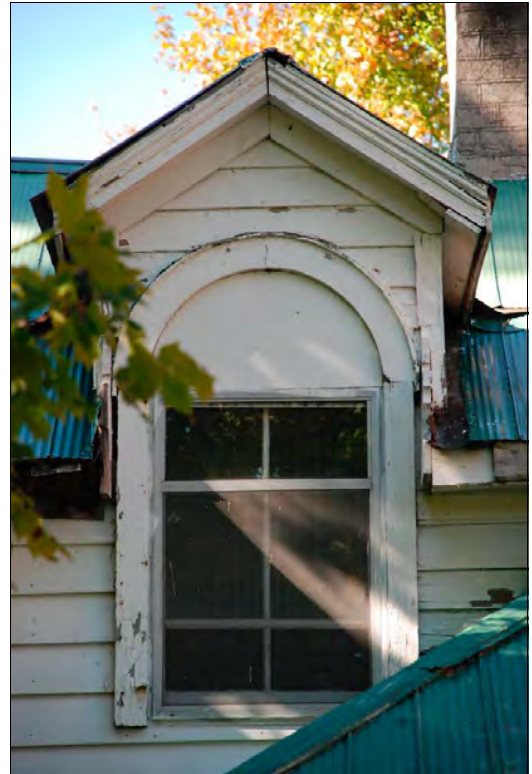
Figure 13 window head blocked-in with plywood circa 1843 tail section
