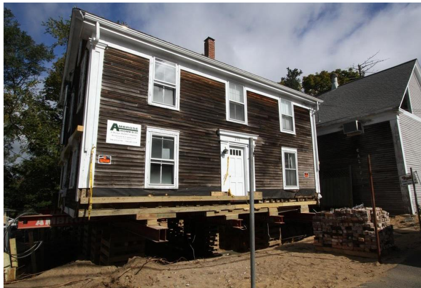
BUILDING ON TEMPORARY SUPPORTS, FOUNDATION ENTIRELY REMOVED
