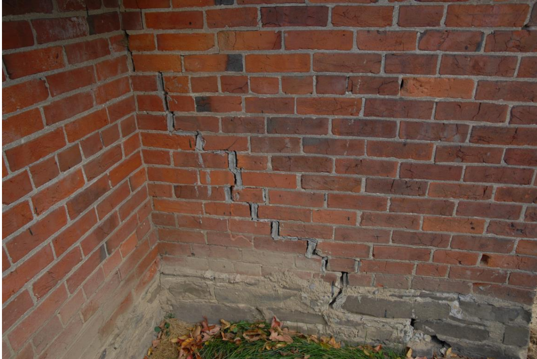
DAIRY SHED - EXAMPLE OF ORIGINAL BRICK AND STONE WORK REQUIRING CONSERVATION –BRICK AND STONE CRACKING PATTERN MAY INDICATE FOUNDATION WEAKNESS
