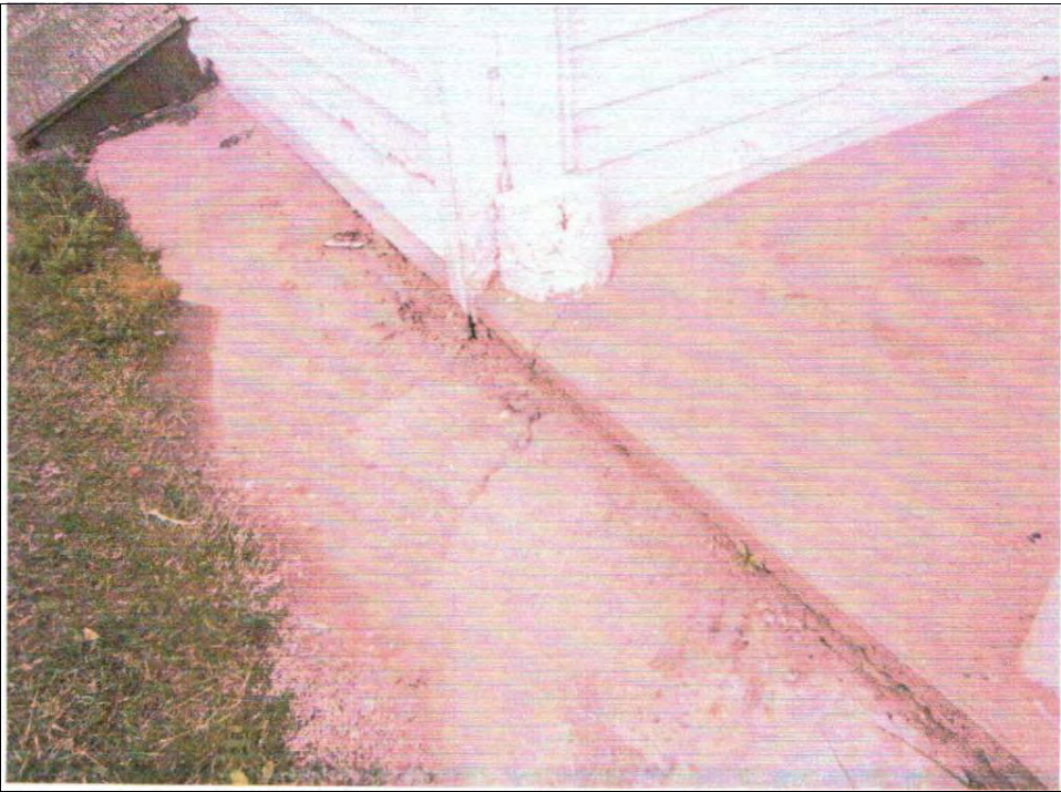
cracking to porch slab & foundation wall
