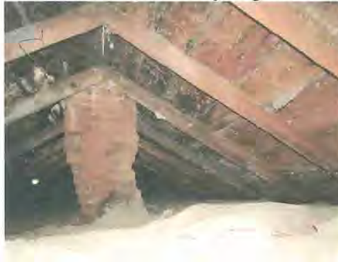
Absence of dormer framing in attic
