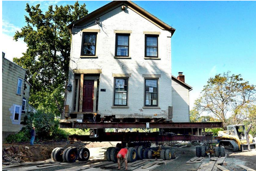
HOUSE SUPPORTED ON TEMPORARY WHEELS
