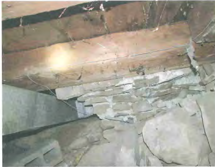
1880s foundation beyond 1840s timber sill plate
