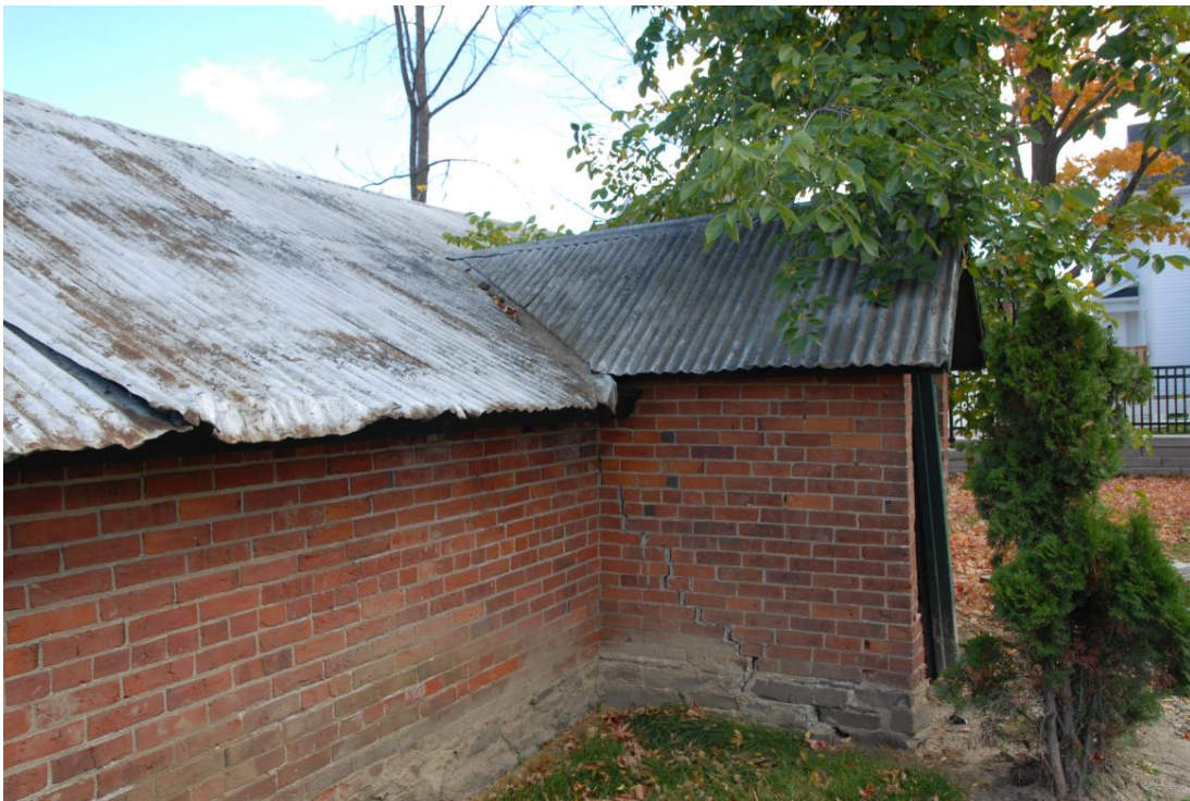
DAIRY SHED SHOWING DETERIORATED ROOF CONDITION
