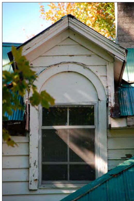
Figure 13 window head blocked-in with plywood circa 1843 tail section
