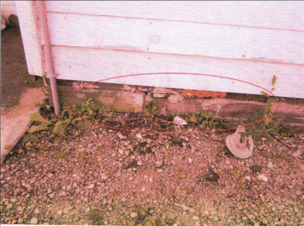
Figure 5 external cracking of foundation wall
