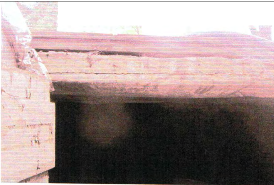
Figure 14 damaged doorway lintel
