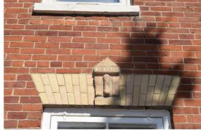
Plate 34: West elevation lower storey window with date keystone
