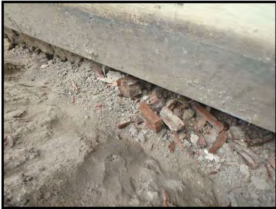
Photograph No. 19 – View of Degradation of Floor Framing of Rear Addition
