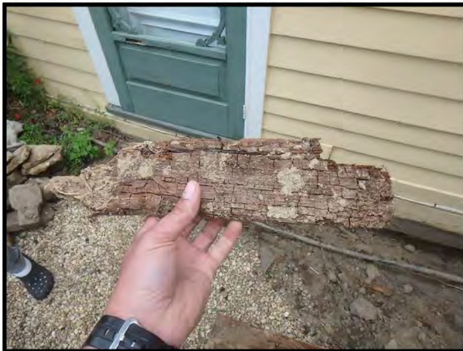
Photograph No. 18 – View of Degradation of Floor Framing of Rear Addition
