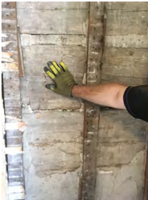
Left: wood framing and wood plank walls
