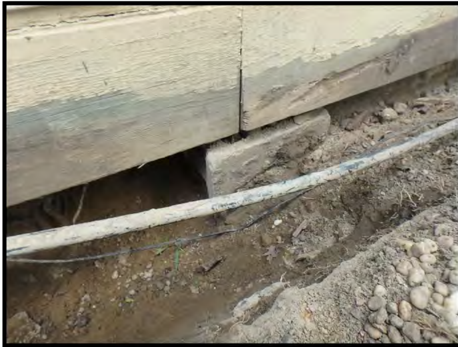
Photograph No. 15 – View of 8” Concrete Block Foundation Elements of Rear Addition
