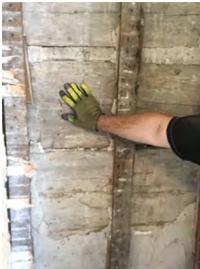
Left: wood framing and wood plank walls
