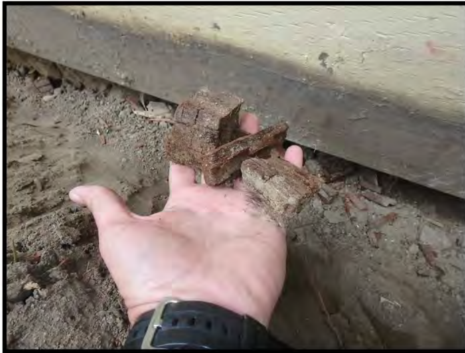
Photograph No. 17 – View of Degradation of Floor Framing of Rear Addition
