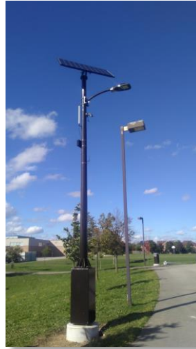
Duncairn Downs Park - Solar PV lighting installation
