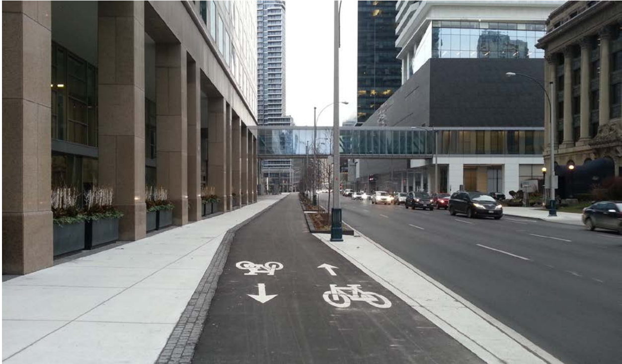
Image: Cycle track parallel to sidewalk with texture separation, City of Toronto
