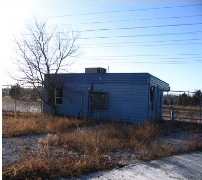
Photo 16 Structure No. 9 – HEPCO Building South Elevation
