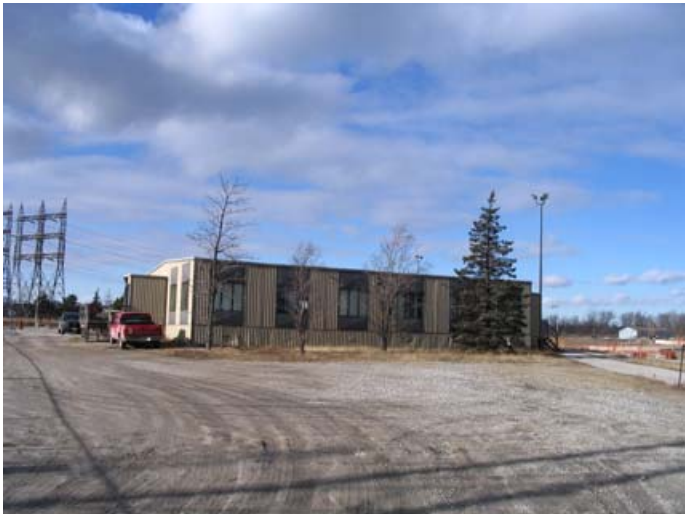
Photo 1 Structure No.1 – Lakeview Rehabilitation Commissioning Office South Elevation
