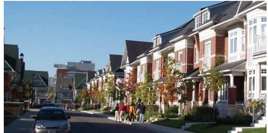
2.2.1- BUILDING RELATIONSHIP TO STREET
