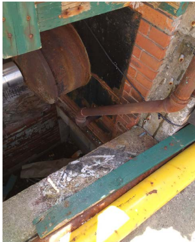
Photograph No. 4 – View of fill line from exterior of building to AST in the basement
