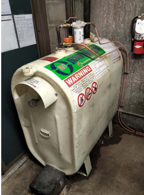
Photograph No. 1 –View of 450 L double-walled steel aboveground storage tank
