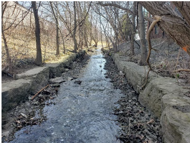
Figure 2-4. Looking downstream. Combination of armourstone banks and gabion bed
