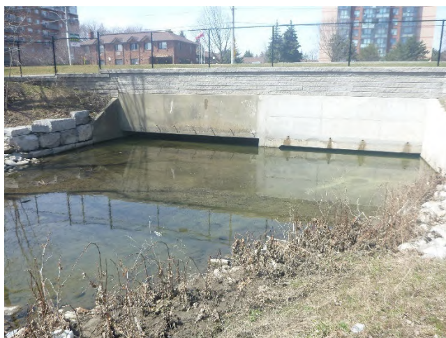
Figure 2-8. Looking upstream towards Applewood Creek and Lakeshore Road East. Aggraded sediment on the downstream of culvert openings
