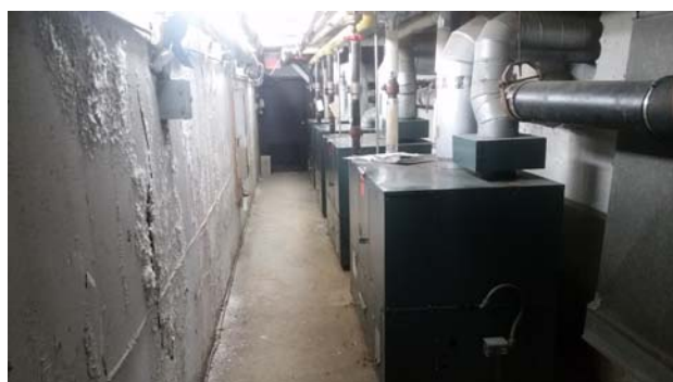
Photograph 3: View of furnace units for the Site Buildings in underground garage
