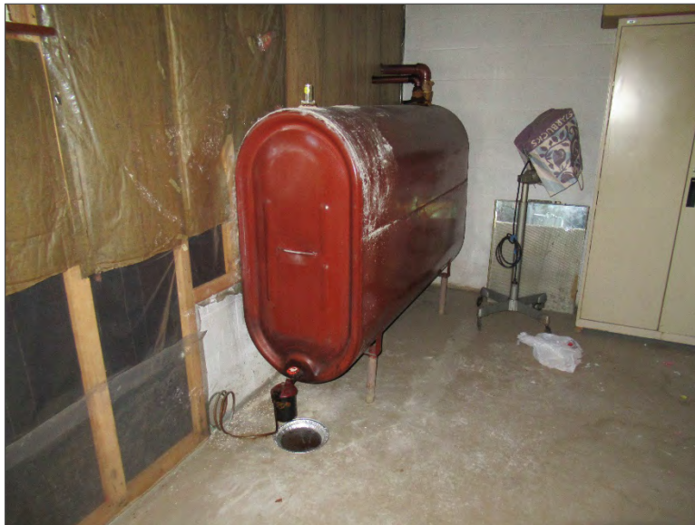
Photo 6 – Fuel oil AST located in the basement of Site Building A.
